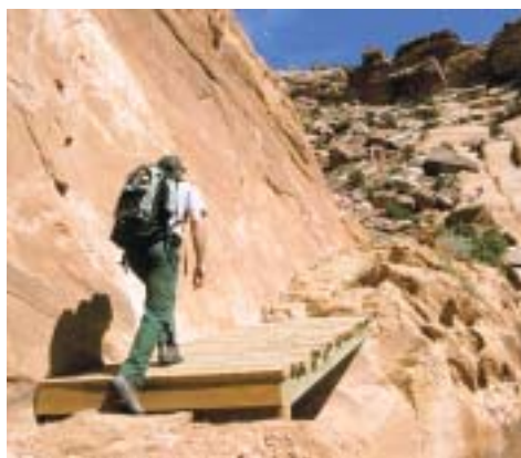
Bridge restoration on the Murphy Trail
