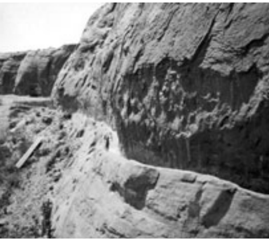
Irrigation ditch constructed by Mormon pioneers, Moenkopi Canyon, Coconino County, Arizona, 1909. Courtesy of USGS.
