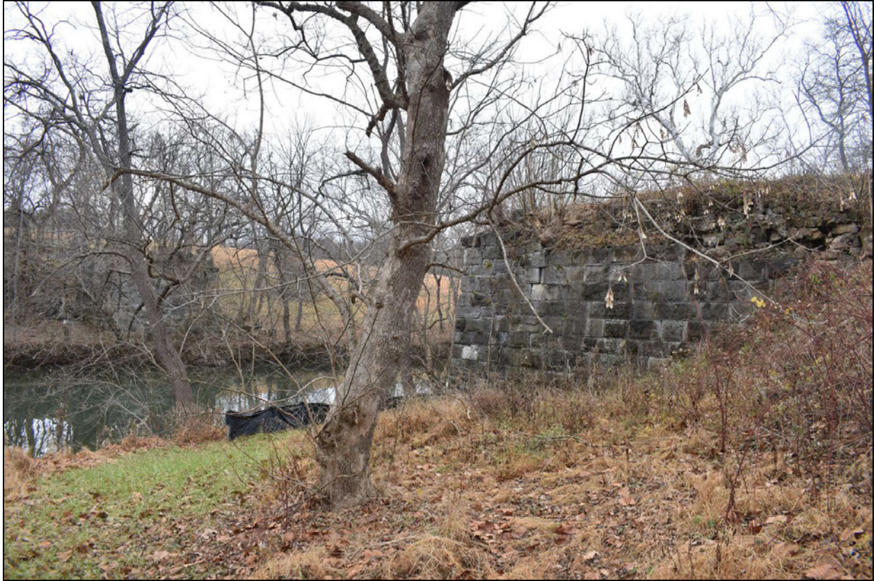
35 of 55. Valley Pike Bridge South Abutment over Cedar Creek, facing north.
