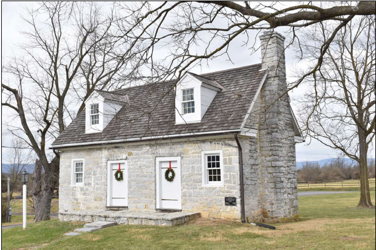
26 of 55. Plantation Office and Store, facing northwest.
