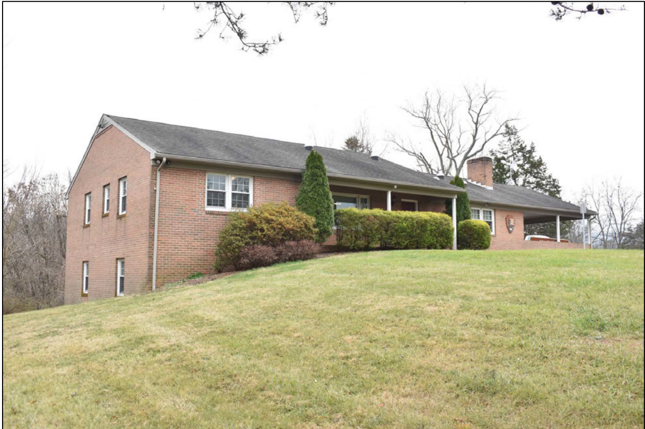
55 of 55. Park Headquarters, 8693 Valley Pike, facing south.
