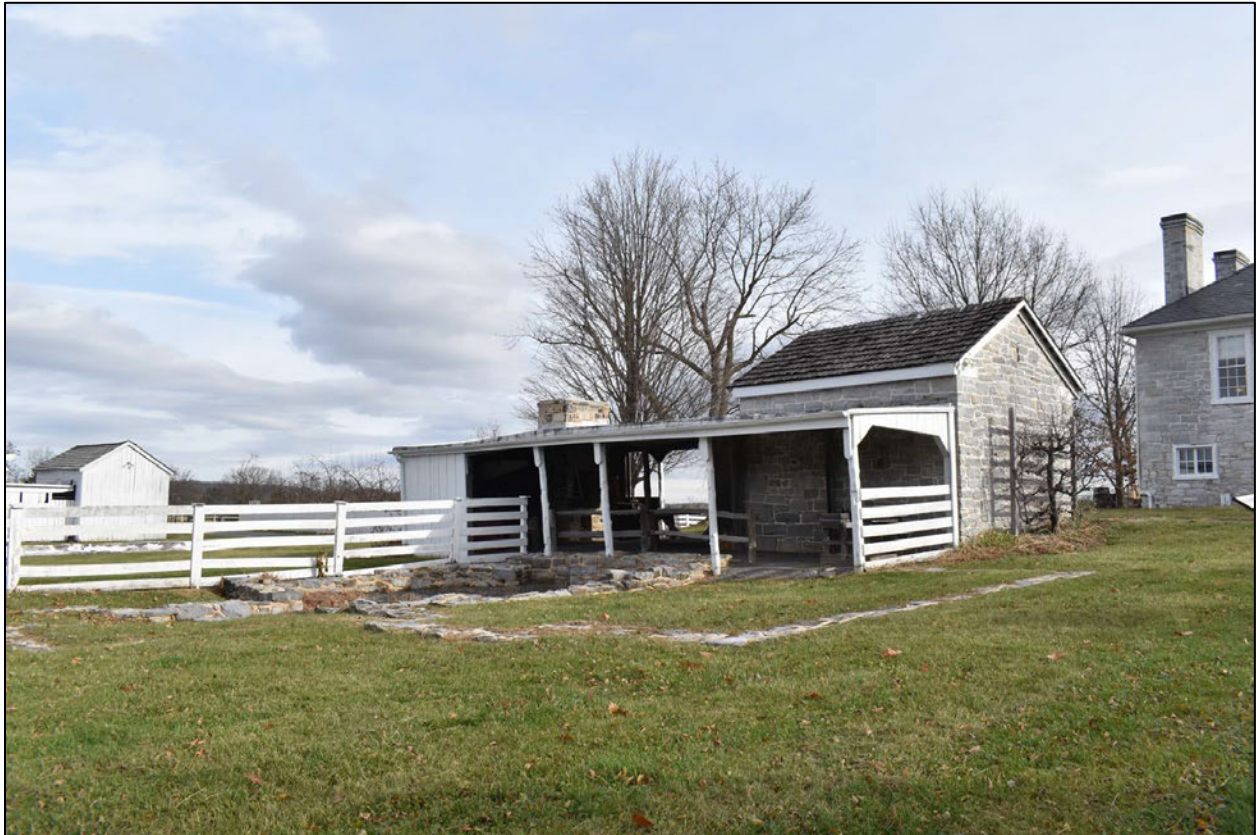
22 of 55. Belle Grove Shed 1, Old Hall Foundation, and Belle Grove Meat House (left to right), facing northeast.
