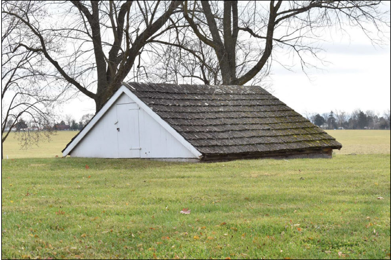
20 of 55. Belle Grove Icehouse, facing southeast.
