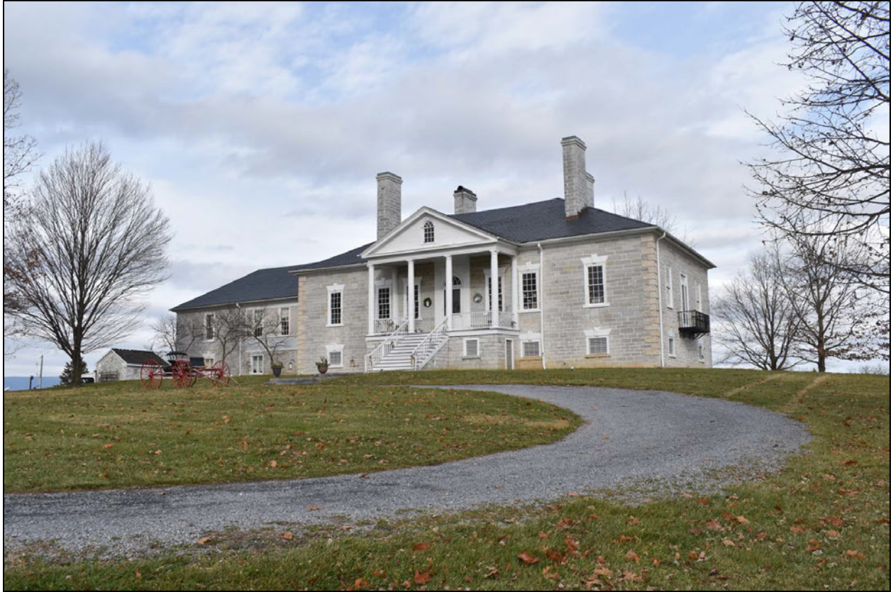
16 of 55. Belle Grove Manor House and Belle Grove Meat House (behind), facing north.
