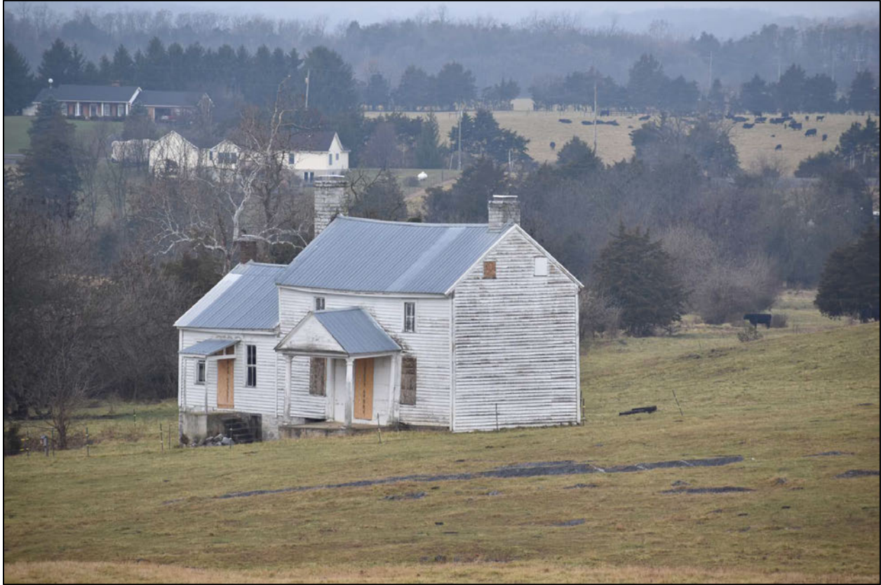
13 of 55. Solomon Heater House and Heater Farmstead, looking northwest.
