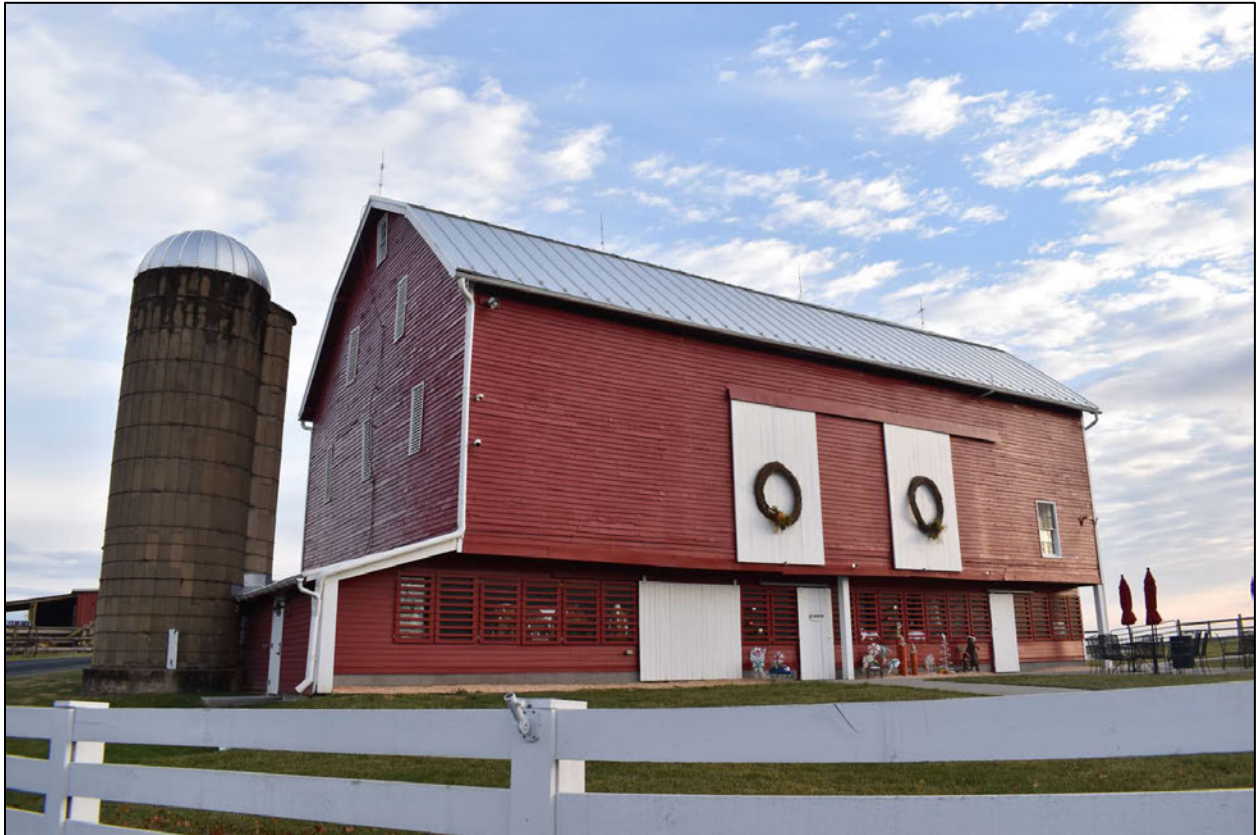
24 of 55. Belle Grove 1918 Bank Barn, facing northeast.
