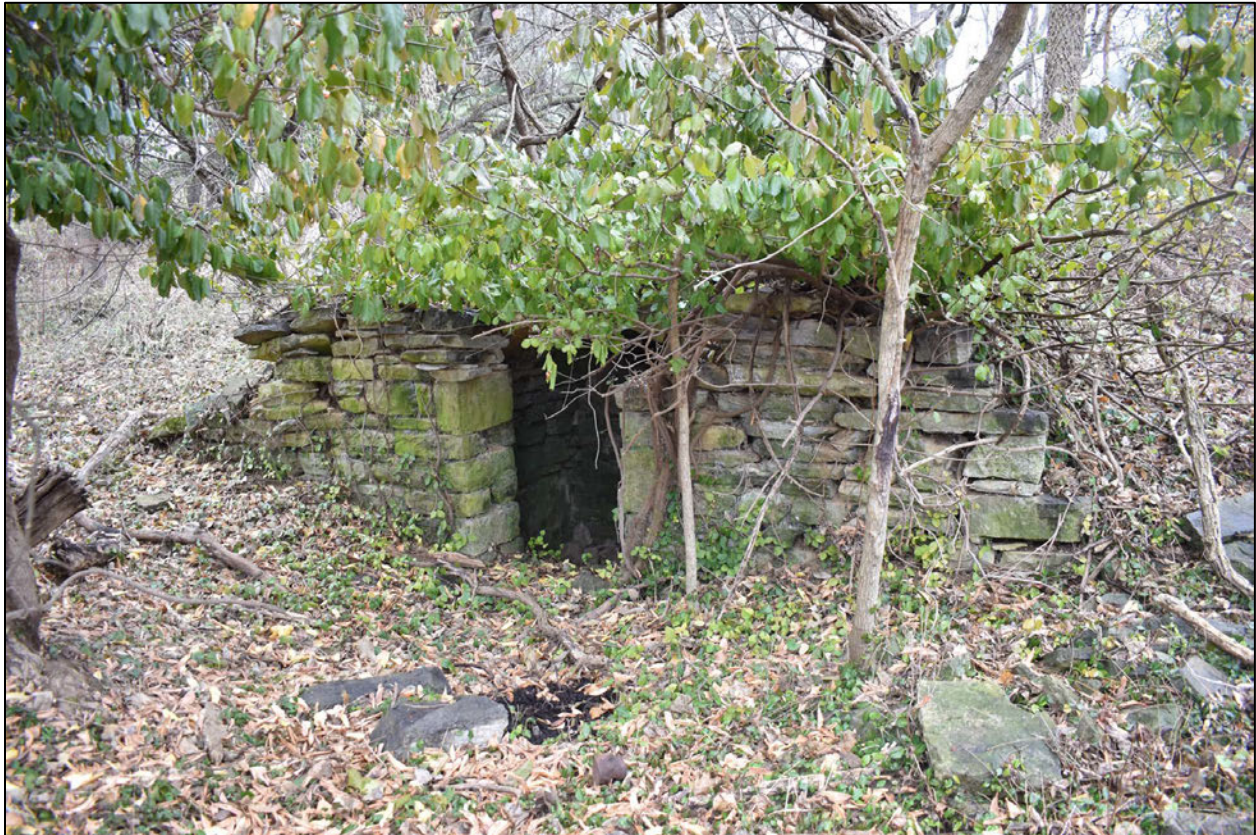
8 of 55. Miller-Kendrick-Walter Root Cellar, facing southeast.
