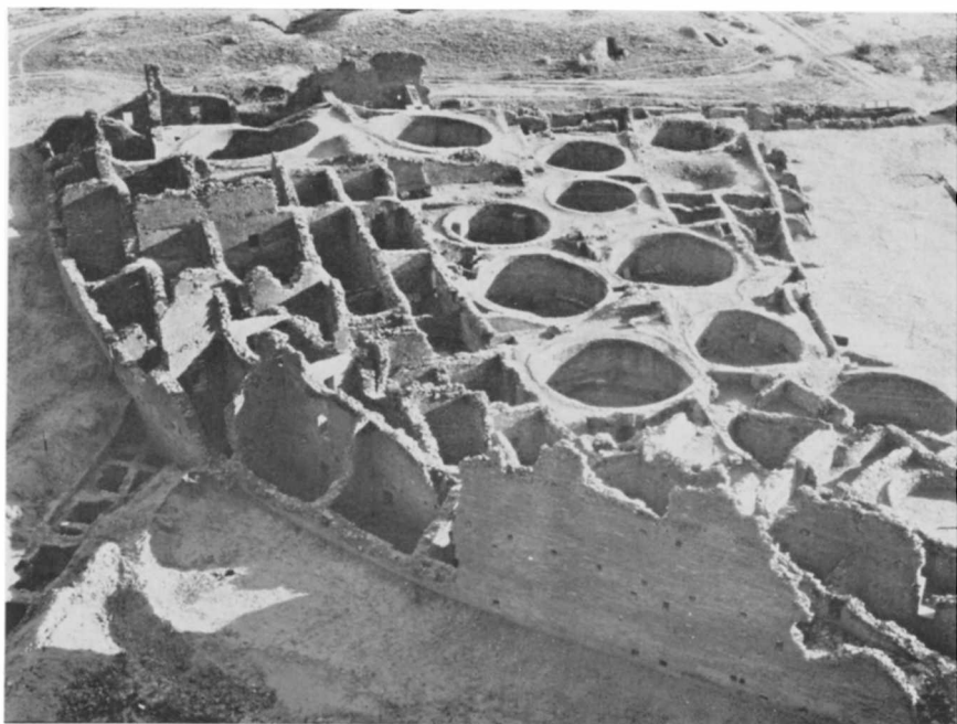
The Late Bonitians' third and final addition to the pueblo overlies units of the Northeast Foundation Complex. National Geographic Society repairs appear in the 4-story wall at right. (Photograph by E. L. Wisherd, 1923.)
