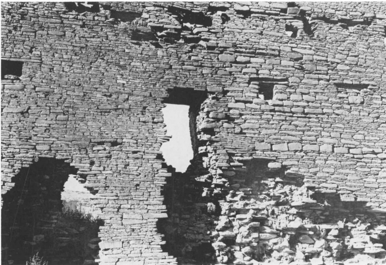
PLATE 53.—Late Bonitian architects inserted tie-poles at intervals to bond their fourth-type veneering (left) to the older stonework.
