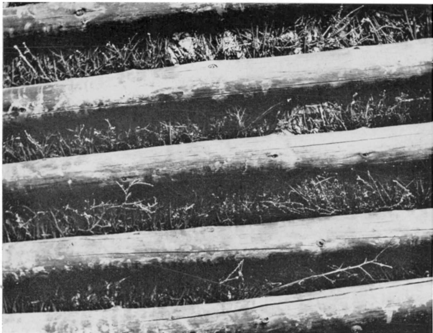
A typical Old Bonitian ceiling usually contained a layer of chico brush.
