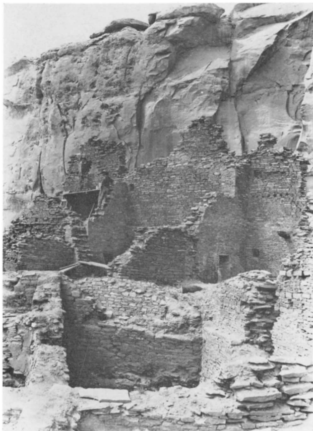
Repairing north wall of fourth-story Room 189D. At right, holes for 7-pole storage shelf, Room 186C, and repaired areas (lighter stonework).
