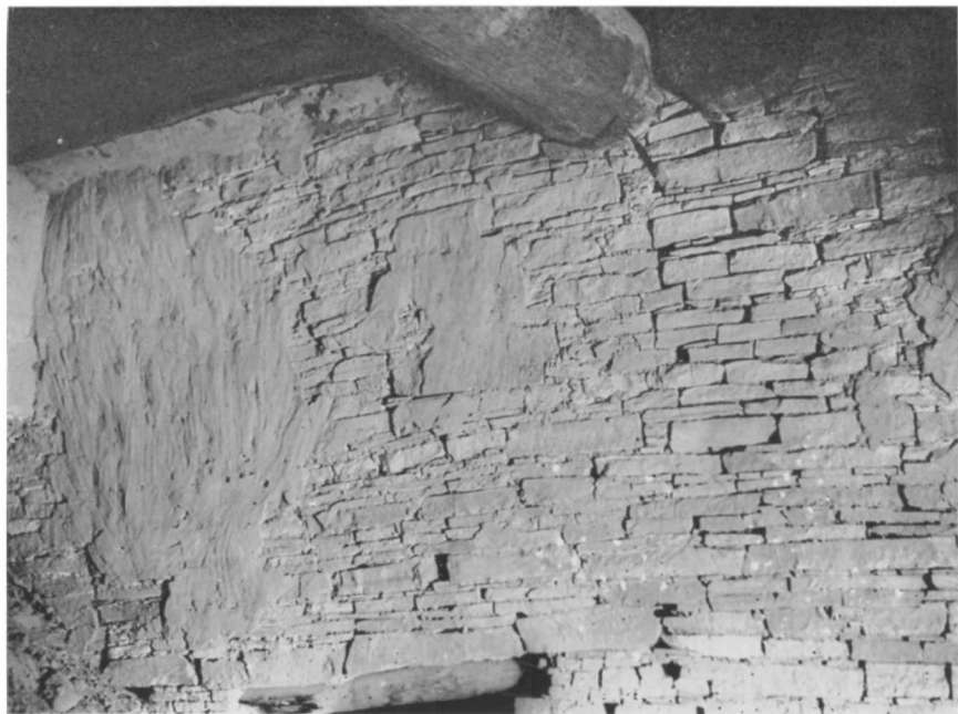
A single 10-inch beam supported the ceiling of Room 227 with the end of another protruding from 227-I.
