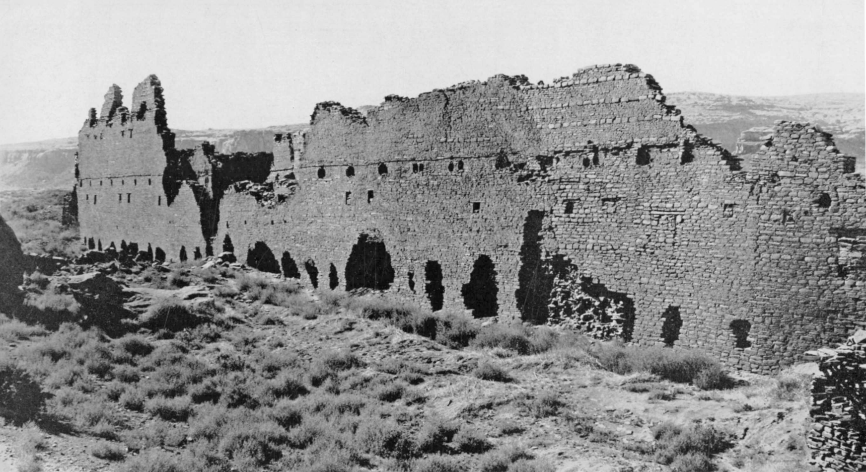
PLATE 28.—Ceiling beams in Room 297B were seated higher than those in 299B (above blocked door, right margin) to approximate roof level of Old Bonitian Room 298C. Fourth-type masonry merges with second-type outside 297.
