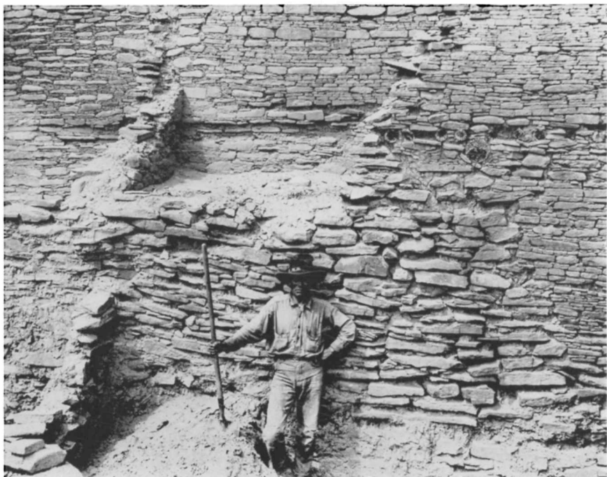
Third-type replacement of first-type masonry, north wall of Room 86B. Second-type interior, room north of 296B, at upper left.
