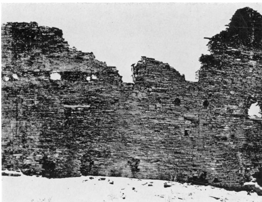
Empty beam holes in Room 299B (right center) are about 2 feet lower than those of Room 297B, next on the left. At lower right, the broken north door of Room 301.
