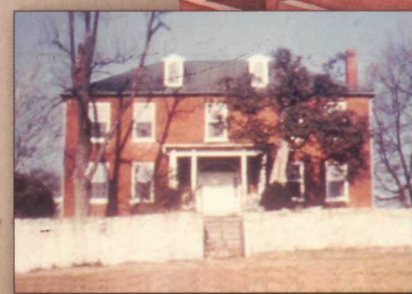
Ferry Hill mansion with one-story porch, 1945.
