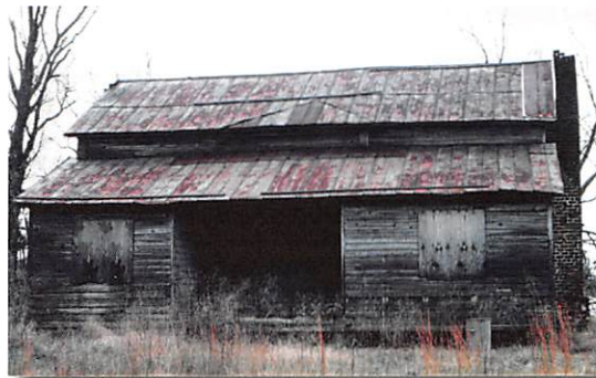
Before NPS Restoration
