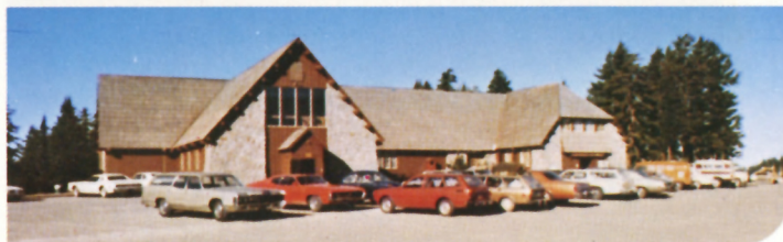
EXTERIOR OF BUILDING. FRONT VIEW OF CAFETERIA/GIFT SHOP
