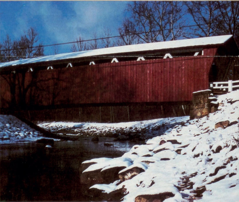
The Everett Road covered bridge keeps snow off the roadway.
