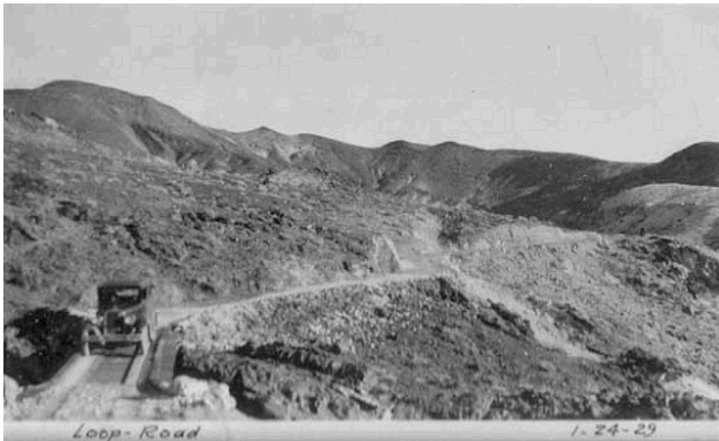
Photograph of the loop road and the wooden bridge, view north. The bridge was built on the northeast portion of the Lower Vine property in 1926 (Album 13732 DEVA 40674).
