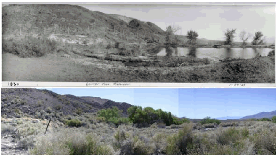
Images of the reservoir located approximately one mile west of Scotty's ranch house, view east. Although the structure remains intact, it is no longer in use (Top: Album 17372 DEVA 40721 Bottom: PWR 2004).
