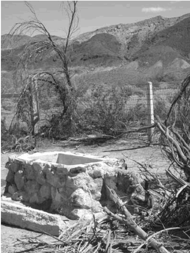
Image of the Lower Vine ranch trough, built by Johnson to maintain the water rights of his property, view northwest (PWR 2004).
