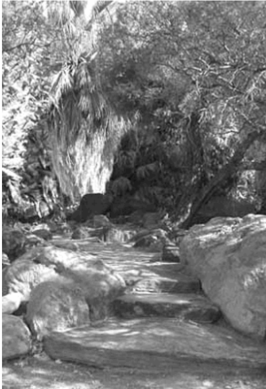
Photograph of a typical stone stairway in the watercourse. Stone walkways were also constructed at the cook and guest houses (PWR 2004).
