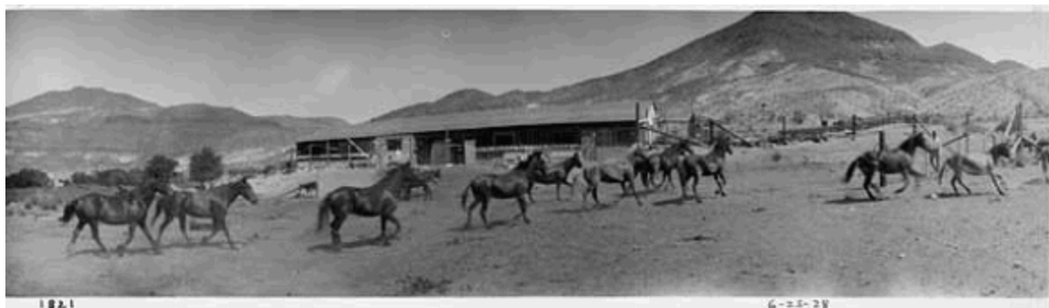
The stables was designed as a support building where Scotty spent time tending to the horses. The corral, seen in the foreground, was in use throughout the historic period. View north (DEVA 40712).
