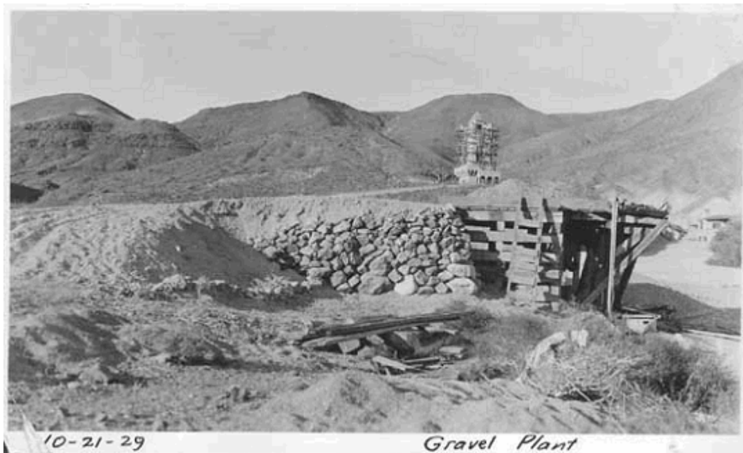
Image of the gravel separator in 1929, view west. This utility structure was used to manufacture concrete (DEVA 40790).
