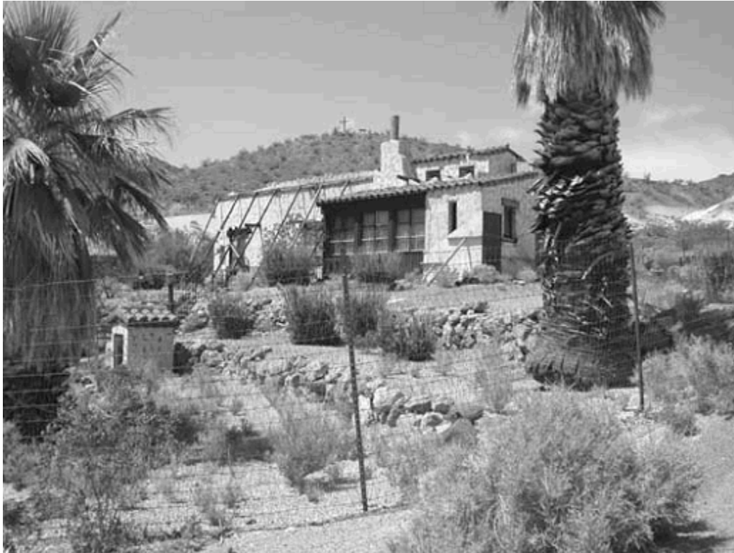
In addition to buildings, several stone and concrete retaining walls were built to create planting beds. This dry-stack rock wall was built by Dewey Kruckeberg (PWR 2004).
