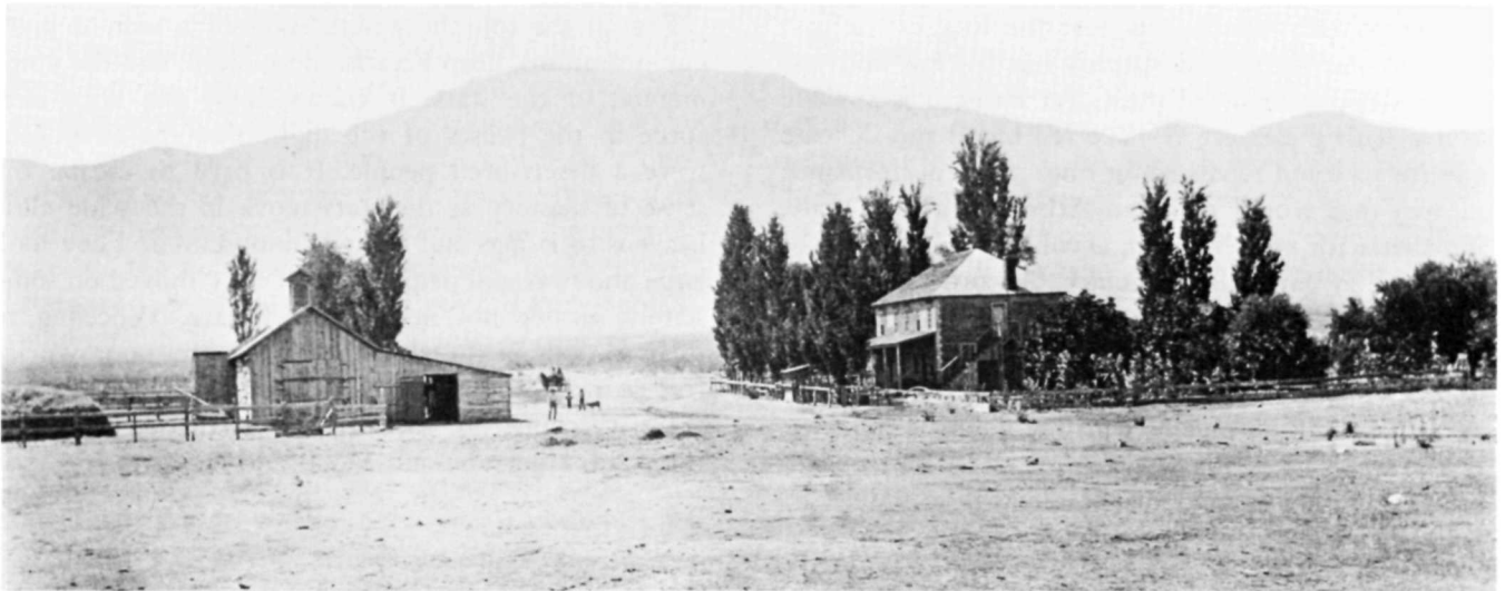
Rose Station, Kern County. Photo courtesy Tejon Ranch Co.
