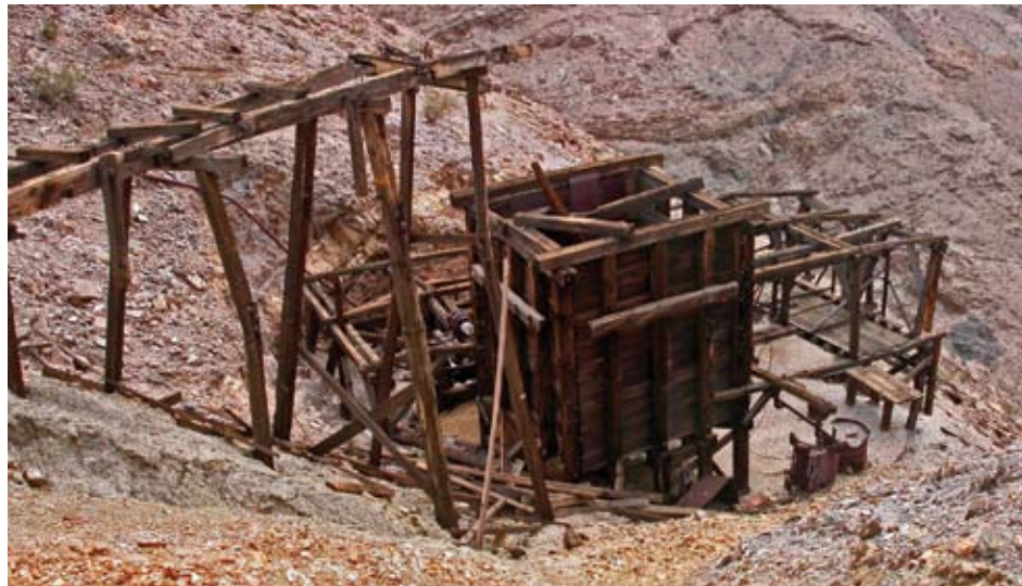
The Keane Wonder Mine, Mill, and surrounding mining area are currently CLOSED to all public access until the numerous hazards can be mitigated.
