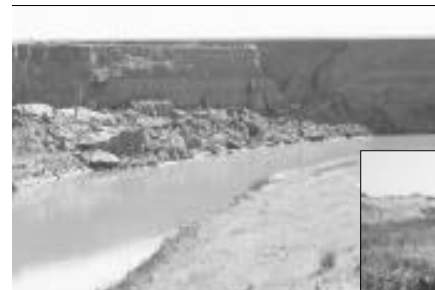
Erosion along Muddy Creek, like that shown above, has cut the bank so severely that it forms a 20-foot vertical wall above the stream bed. Low-profile rock grade control on both sides of the creek, at right in foreground, has improved riparian areas in the Muddy Creek corridor. Photos by R. Wittler
