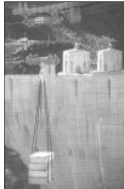
Hoover Dam's 1932 cableway is still able to lift 187 tons. BOR photo by Andrew Pernick
