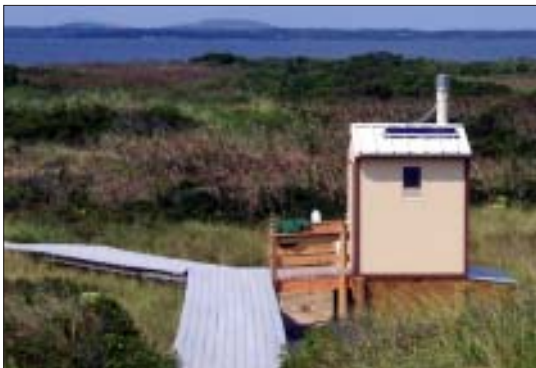
Thanks to generous contributions and cooperative efforts, an environmentally friendly replacement for the Old Inlet comfort station was installed in the wilderness area.
