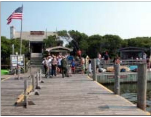
Sailors Haven facilities show signs of deterioration. Plans for the new marina were reviewed in 2003.
