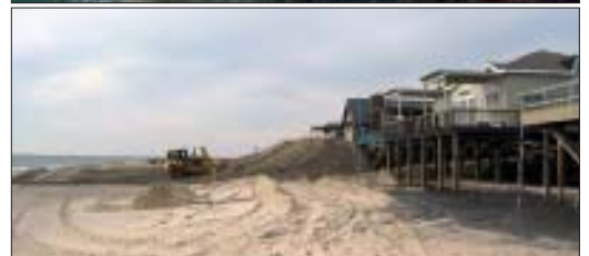
Fire Island Pines planned to add 1.2 million cubic yards of sand to its beach. Western Fire Island communities will restore 700,000 cubic yards.
