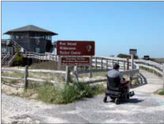
The accessible boardwalk west of the Fire Island Wilderness Visitor Center was partially refurbished during the fall of 2003.
