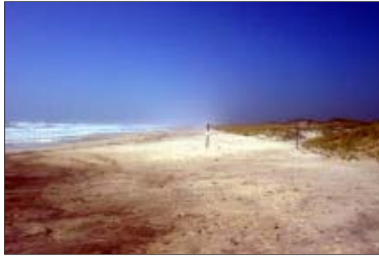
Beach in front of Wilderness Visitor Center gained sand during Hurricane Isabel, while Watch Hill beach and dunes (right) were eroded.
