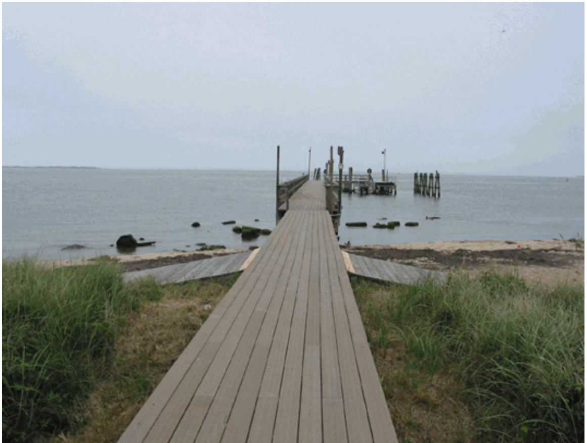
Boardwalk leading from Radio Compass Station complex towards Pier. (OCLP 2004)
