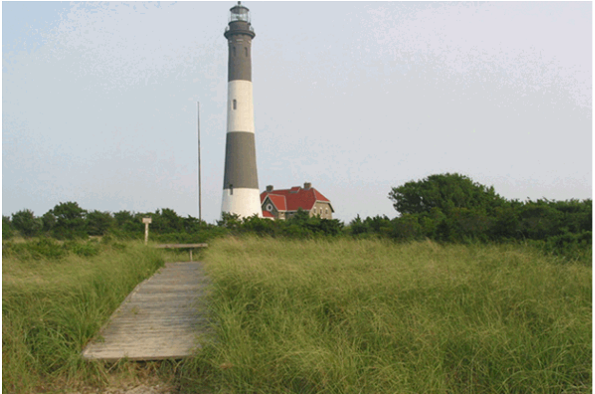
Fire Island Lighthouse and Keeper's Quarters. The Terrace isn't visible. (OCLP 2004)
