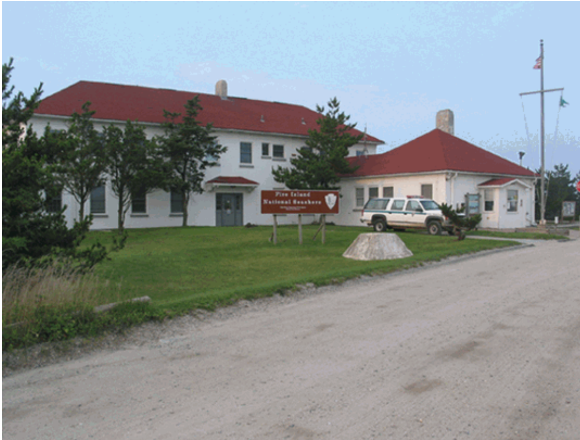
U.S.C.G. Annex from Burma Road. A radio tower foundation is in the midground. (OCLP 2004)
