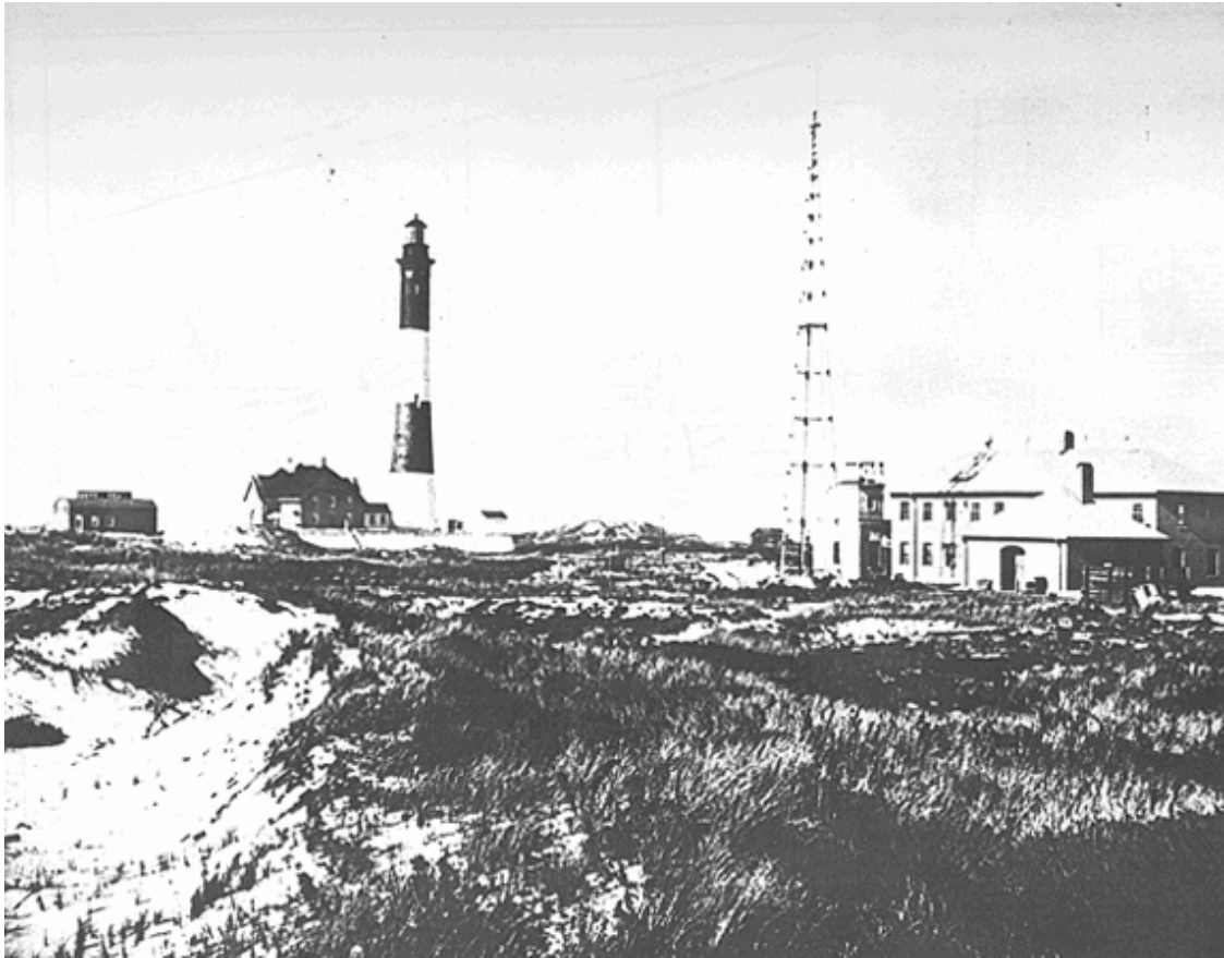
U.S. Naval Radio Compass Station. Radio towers were installed throughout the property, including the one pictured here to the left of the Annex Building, 1920-1936. (HSR)
