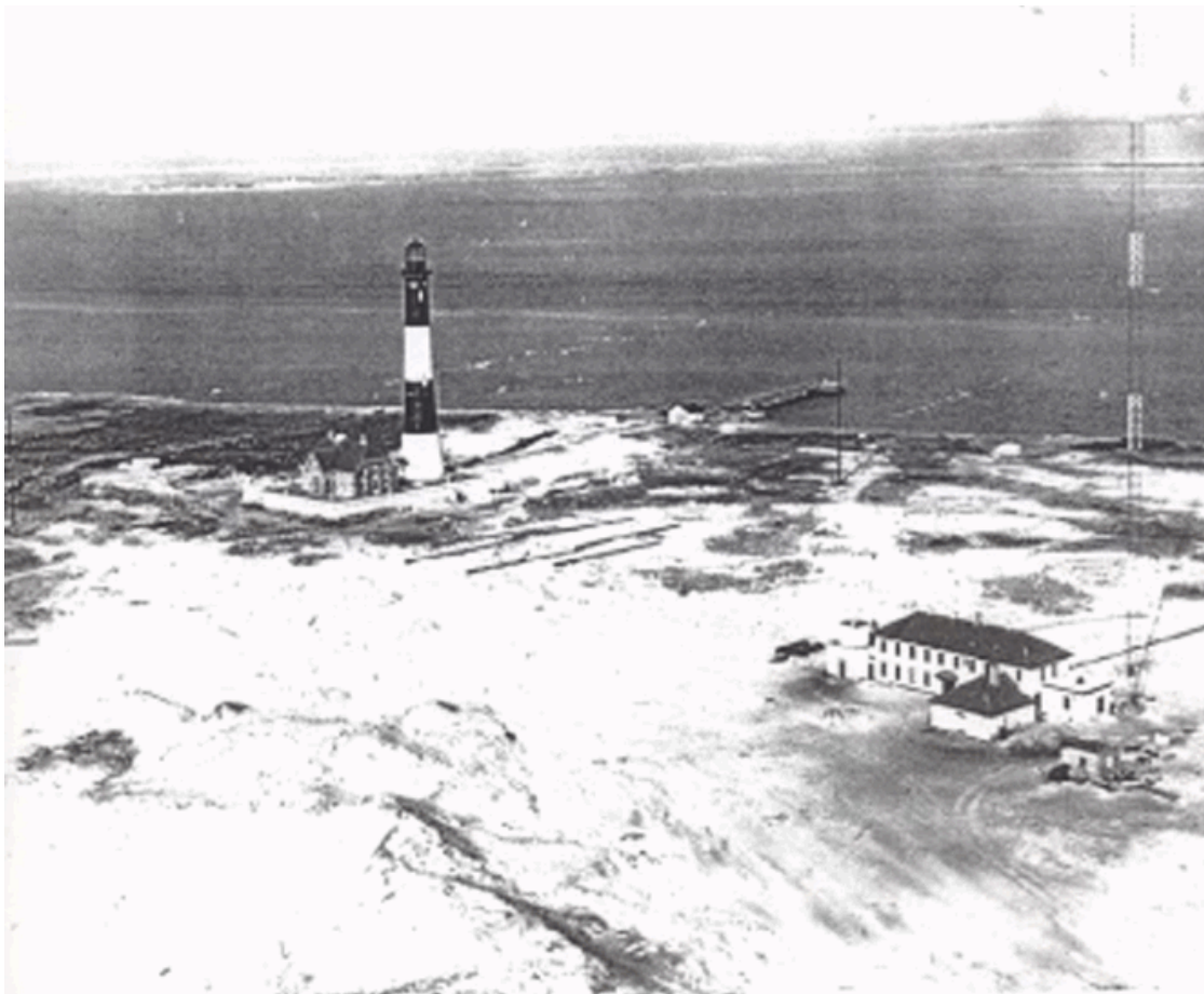
Fire Island Light Station and U.S. Naval Radio Compass Station depicts changes that have occurred in landscape including: elimination of Power house and Fire Island Marine Station. Notice clear view of boathouse, pier, 300' radio tower, after 1939. (HSR)
