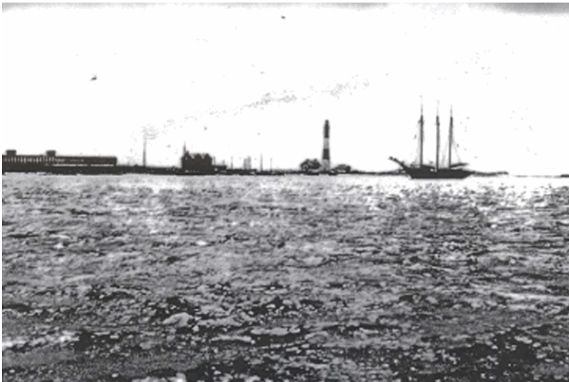
View of west end of Fire Island from Great South Bay. Surf Hotel appears at far left with Fire Island Light Station at right. An unidentified building, perhaps a hotel or barracks sits between them, 1891-1917. (Source unknown)
