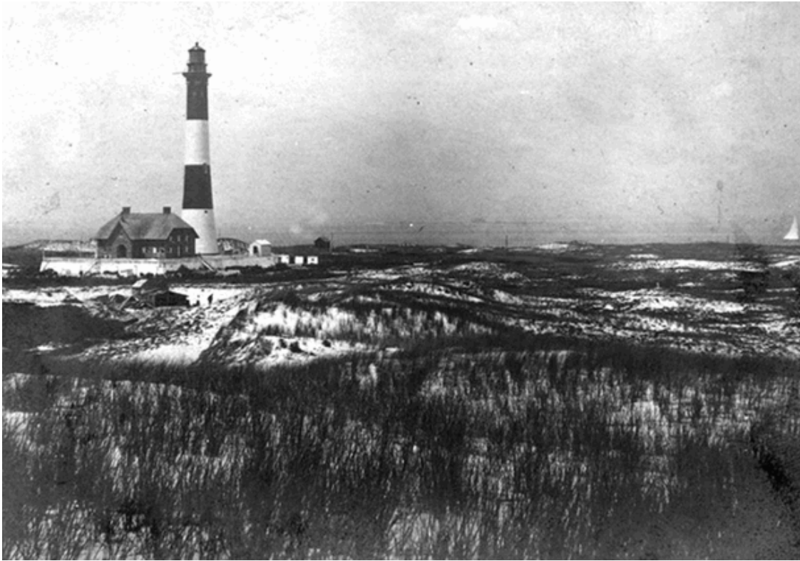
Looking NW from dunes towards Light Station. In view (L to R) is Terrace, Keeper's Quarters, Lighthouse, small shed, boathouse along shoreline, and identified structures just NE of Terrace, 1891-1936. (Library of Congress)
