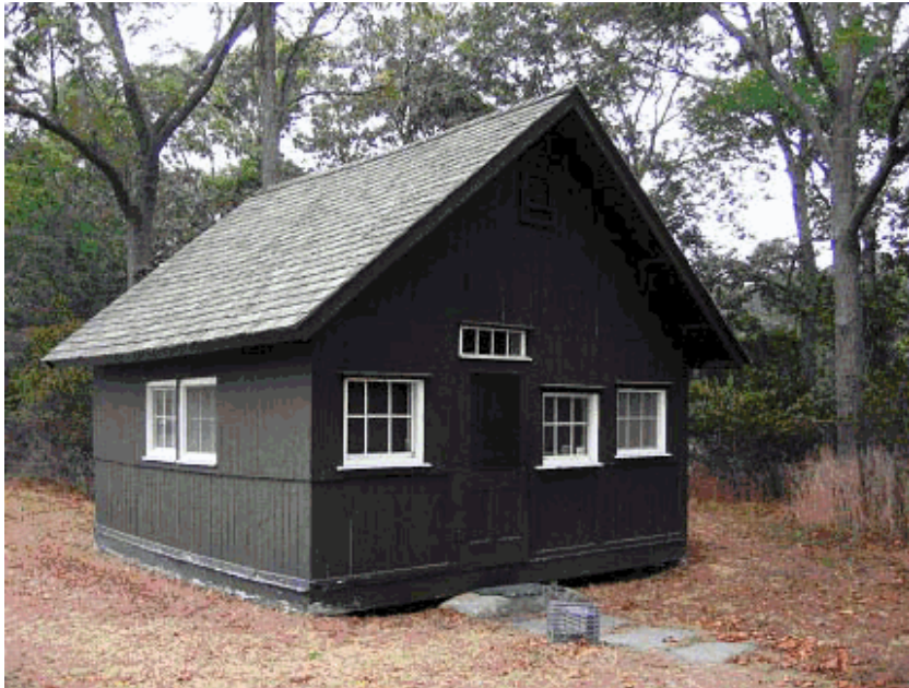
Caretaker's Workshop, now used as administrative office for the site. (OCLP, 2005)
