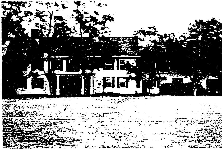
FRONT (SOUTH) VIEW, FLOYD HOUSE
