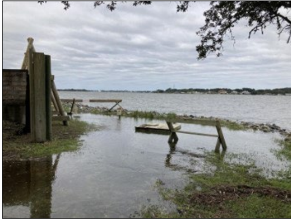
Figure 2. Flooded Walkway on Northeast Corner of Fort Exhibit
