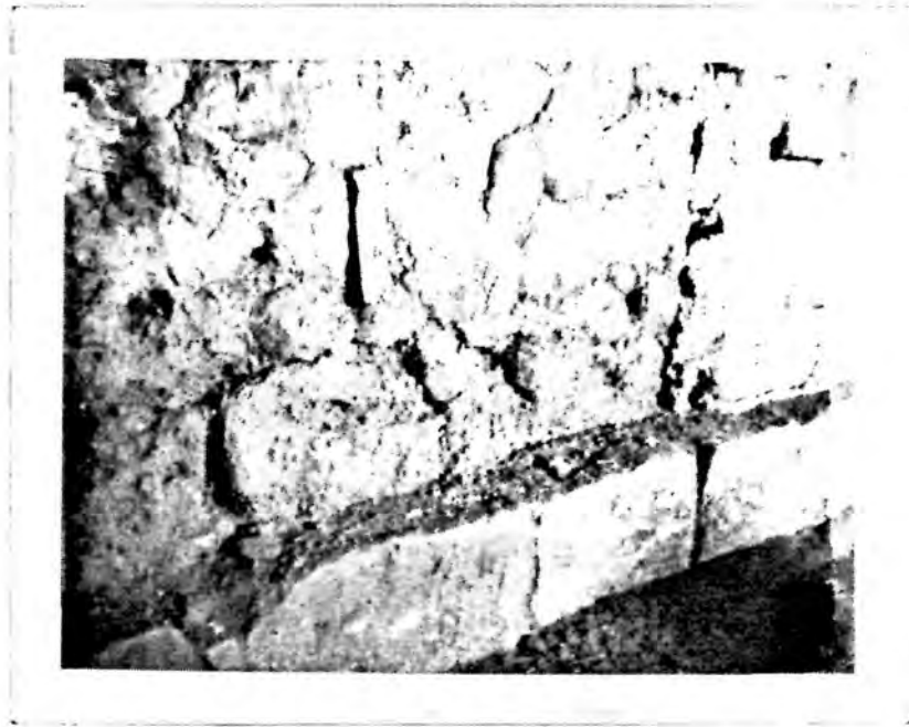
Illustration 9. Stone foundation with adobe wall, north squad room
