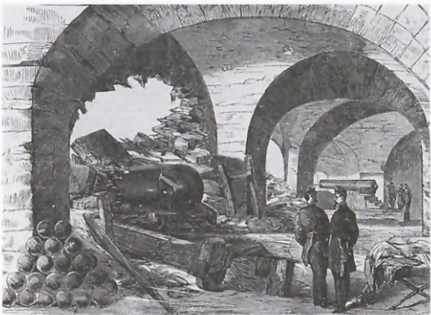
Interior view of Pulaski’s southeast casemates showing the breach made by the Federal batteries that helped bring about the surrender of the fort.
