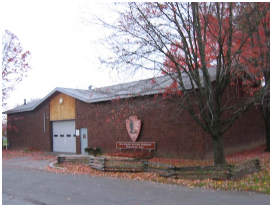
Figure 2: Fort Stanwix Maintenance Facility.
