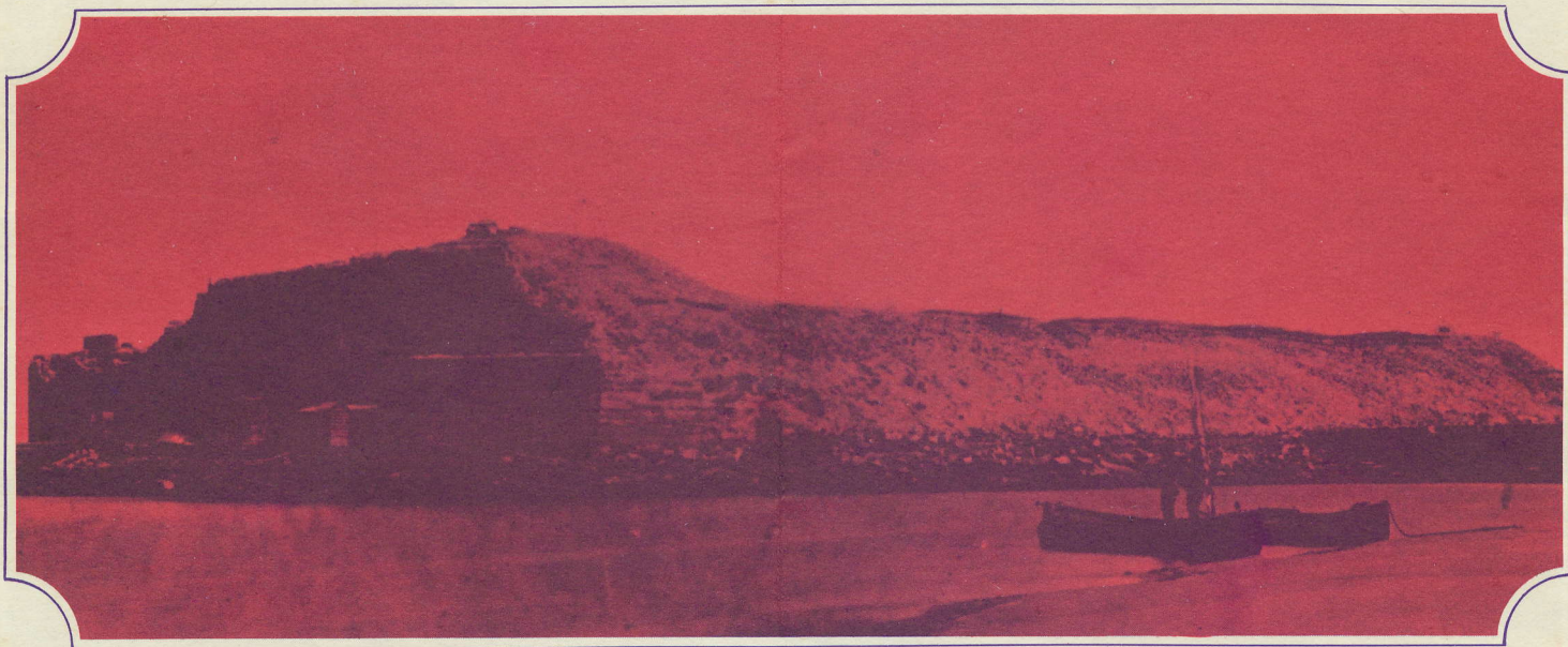
Pounded by 3,500 tons of metal, Fort Sumter was a mass of rubble and ruin by war's end. This view shows the condition of the left flank and gorge (right) in February 1865.
