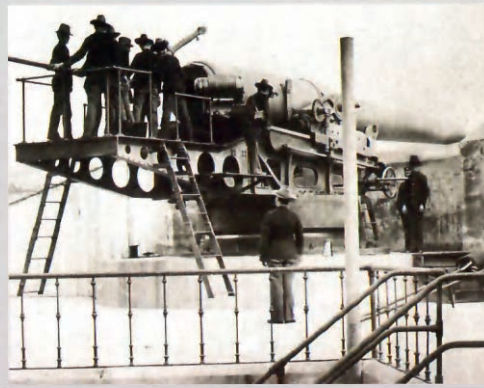
The massive concrete Spanish-American War structure known as Battery Isaac Huger has dominated the entire central section of Fort Sumter since 1899, when the battery was completed. Like the fort in which it stands, it was named for a South Carolina hero of the Revolutionary War. The photo at left, taken in 1901, shows one of the two long-range 12-inch rifles that made up the
