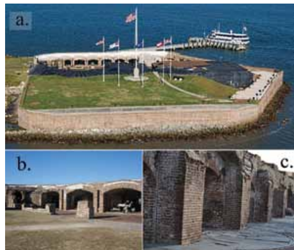
Figure 1: The current state of Fort Sumter National Monument: (a) aerial view, (b) barrel vaulted casemates, and (c) degradation of brick and mortar piers.
