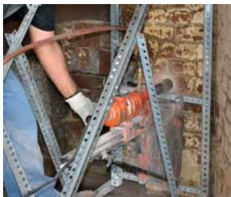
Figure 2: Coring of material samples revealed that although the construction drawings indicate a brick wall across the width, the construction of the fort is composite with tabby concrete infill.
