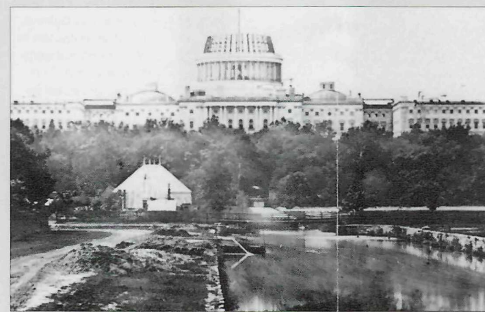
Lincoln's 1861 inauguration took place beneath the unfinished Capitol dome.
