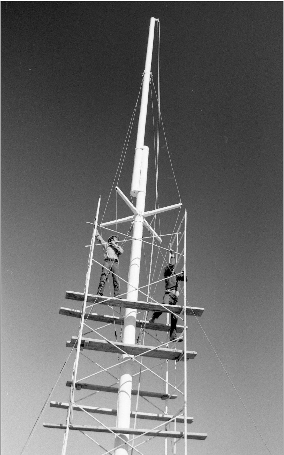
Figure 8 – Flagpole repairs and paint, 1986.
