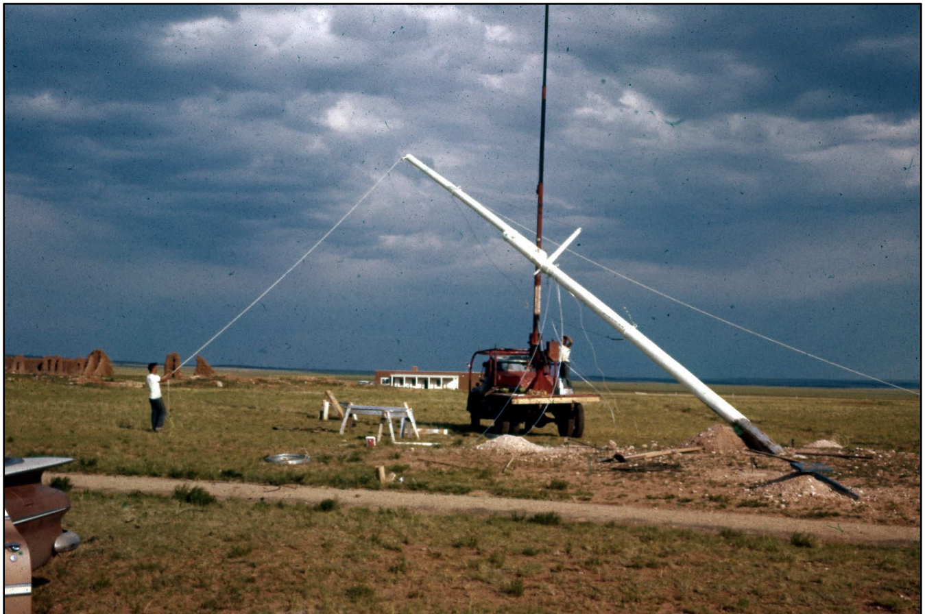
Figure 6 – Erection of replica 62-ft flagpole, 1959.
