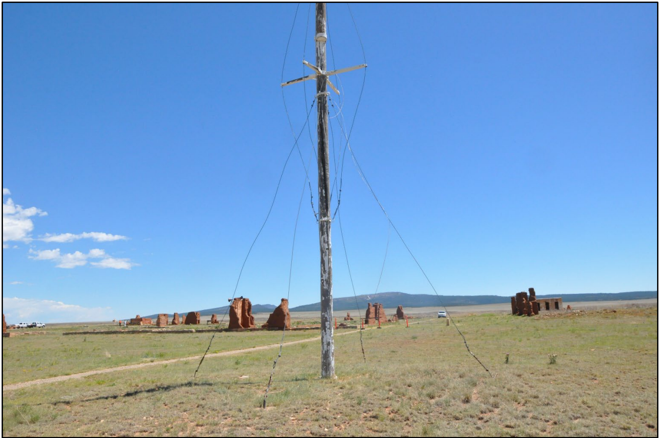
Figure 14 – Flagpole, Large structural crack on lower mast, facing north-east. July 10, 2026.
