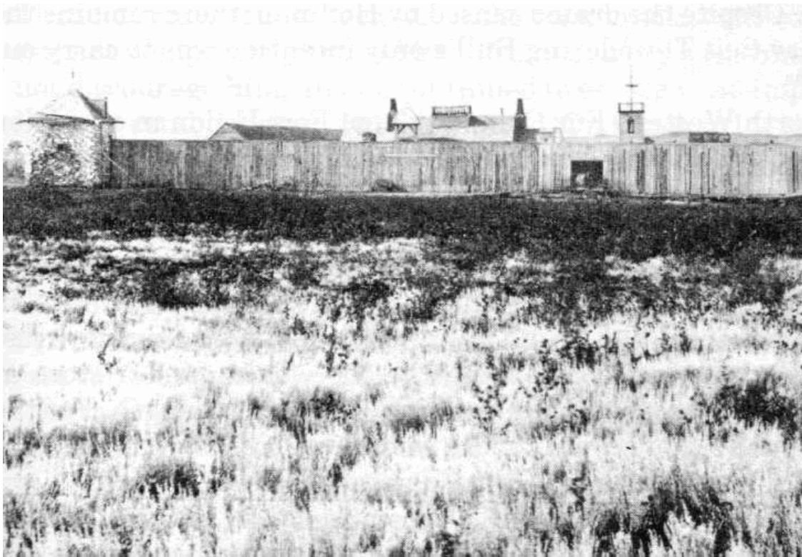
View of the North Palisade, 1866. Deterioration is becoming evident, especially the northeast (left) bastion. (Fort Union Trading Post, A Pictorial History, MWRO. Original is with the Montana Historical Society)
