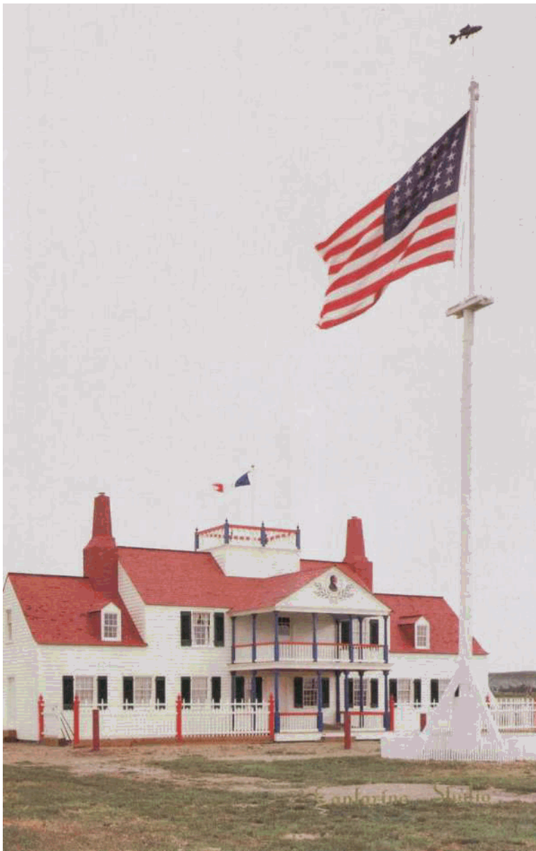
The completed reconstruction of the Bourgeois House and the flagpole. (Fort Union Trading Post, A Pictorial History, MWRO. Photo by Richard Cronenberger, NPS.)
