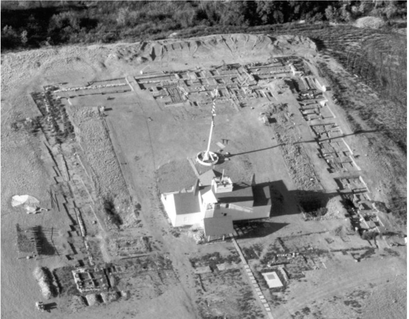
AERIAL OF FORT UNION TRADING POST EXCAVATION WORK, RECONSTRUCTED BOURGEOIS HOUSE AND FLAGSTAFF
