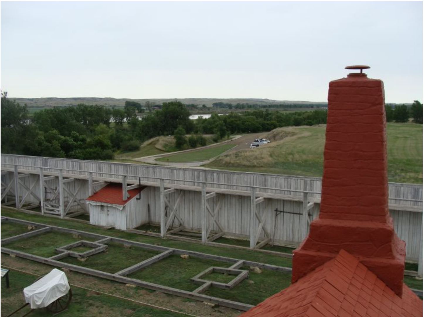
FORT UNION TRADING POST RECONSTRUCTION WEST PALISADE, DWELLING RANGE FOOTPRINT, VIEW TO MISSOURI RIVER
