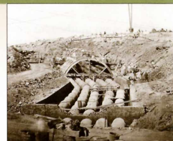
Workers install the Central Park water system.
