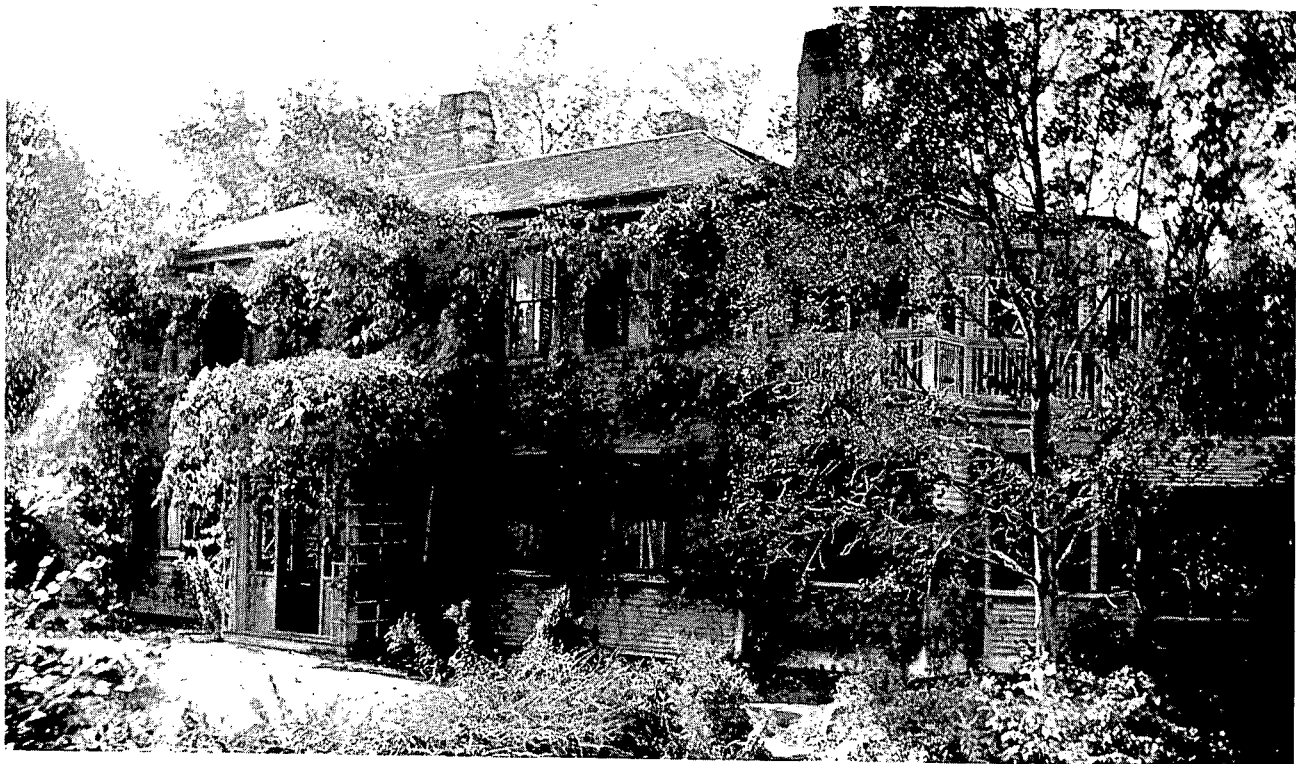
c. 1904. East Facade of House from across the hollow.
