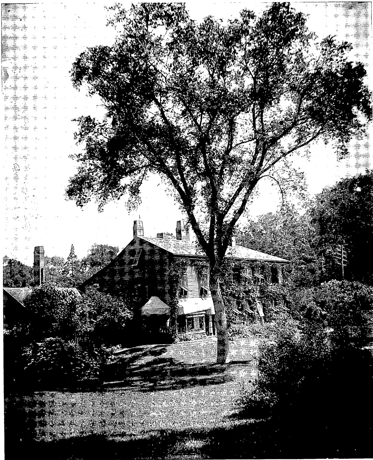
No Date. South Lawn. View Northeast. Note path pattern and plantings where pool and terrace currently stand.
