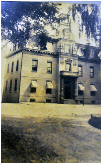
Figure 8. View looking east from the perimeter road at the 1792 State House building prior to its restoration, circa 1898. (Delaware Public Archives)
