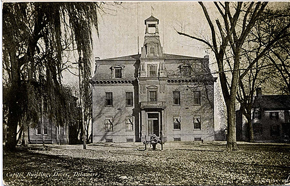
Figure 3. View looking east from the east half of Dover Green to the west facade of the 1792 State House building, circa 1888. Note the cannon in the Green's lawn. (Delaware Public Archives)
