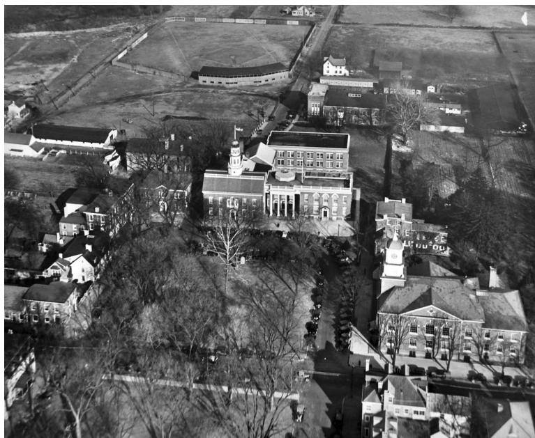
Figure 16. View looking at Dover Green, including 1792 State House and 1875 Court House, c. 1931. A new State House Complex would be built a few years later to the east, just beyond baseball field. (Hagley Museum and Library, Delaware Public Archives)
