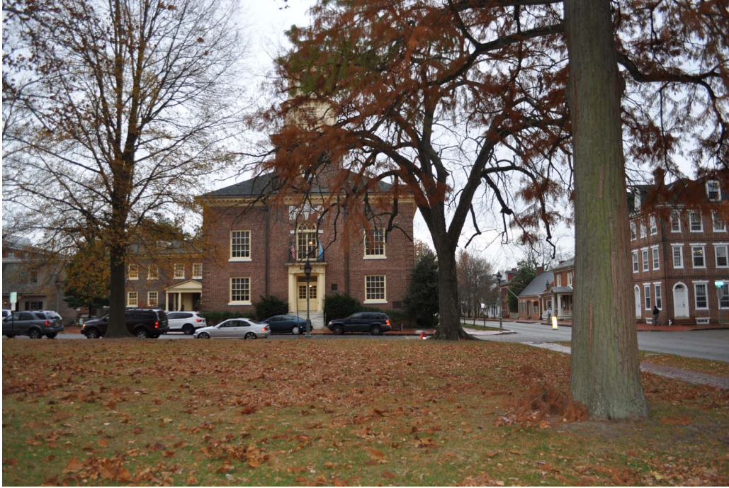
Figure 23. View looking south from the east half of the Green to the north facade of the Kent County Court House. (OCLP 2016)
