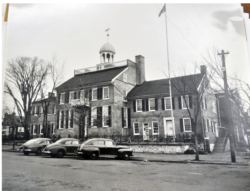
Figure 17. The New Castle Court House, view looking north, c.1945. (Delaware Public Archives)
