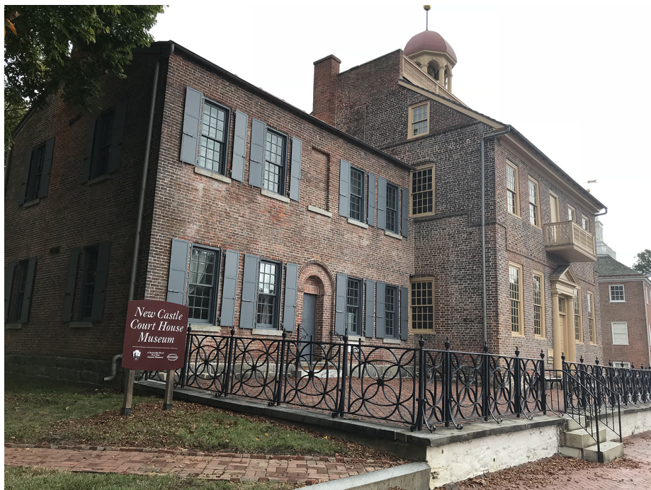
Figure 29. View looking east at the New Castle Court House. The 1845 west wing is at image left, and the original 1731 main block is at image right. (OCLP 2017)
