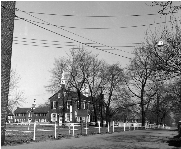
Figure 21. View looking north from Market Street. Note the white fencing (since removed). (Delaware Public Archives)
