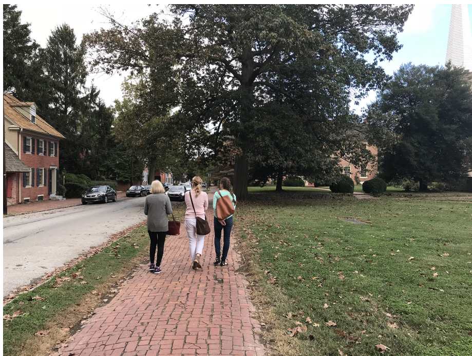
Figure 26. This view looking north along western perimeter sidewalk reveals the crown in the brick sidewalk to promote adequate drainage. (OCLP 2017)
