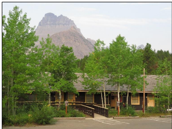
Fig. 22. Modern updates include this ramp and hand rails providing access according to Americans with Disabilities Act (ADA) guidelines. (Author photo.)
