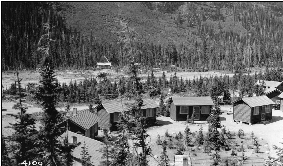
Fig. 10. Newly built Cabin Circle A. The cabin at right is at the opening of the horseshoe-shaped circle. The newly redesigned Many Glacier Campground is visible in the background. The picture was probably taken in 1933, certainly before construction of the general store in 1935 and the Heavens Peak Fire in 1936. (Glacier NP photo GLAC 15546.)
