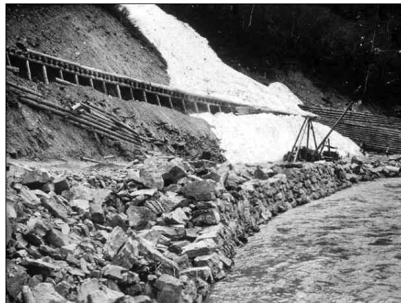
Construction along Red Rock Point, Steven's Brothers Contract to Logan Cr.
