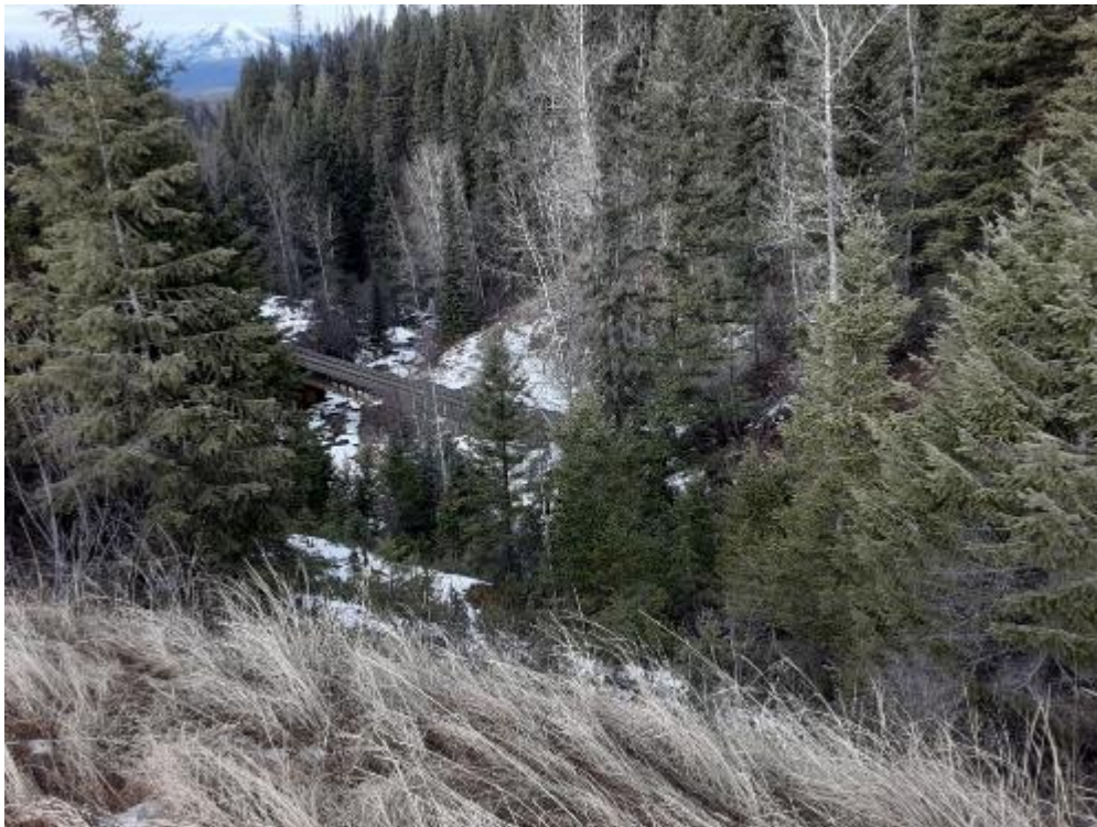
Site 1 - Picture from U.S. Highway 2 at Tunnel Creek- overlooking the train tracks to the northwest.
