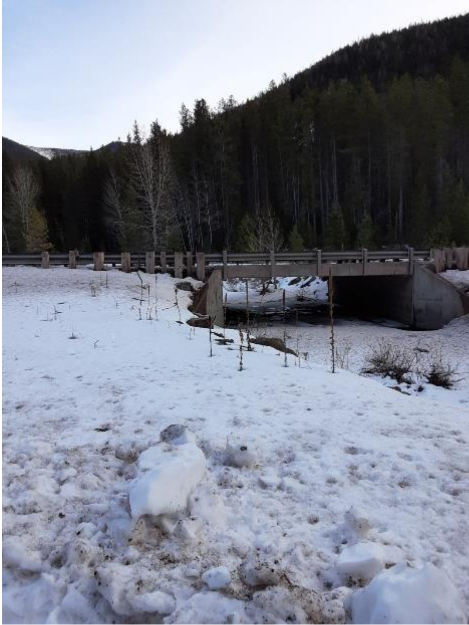
Site 3 - Picture from Devil Creek of the bridge crossing. The cameras are to the east of the bridge.
