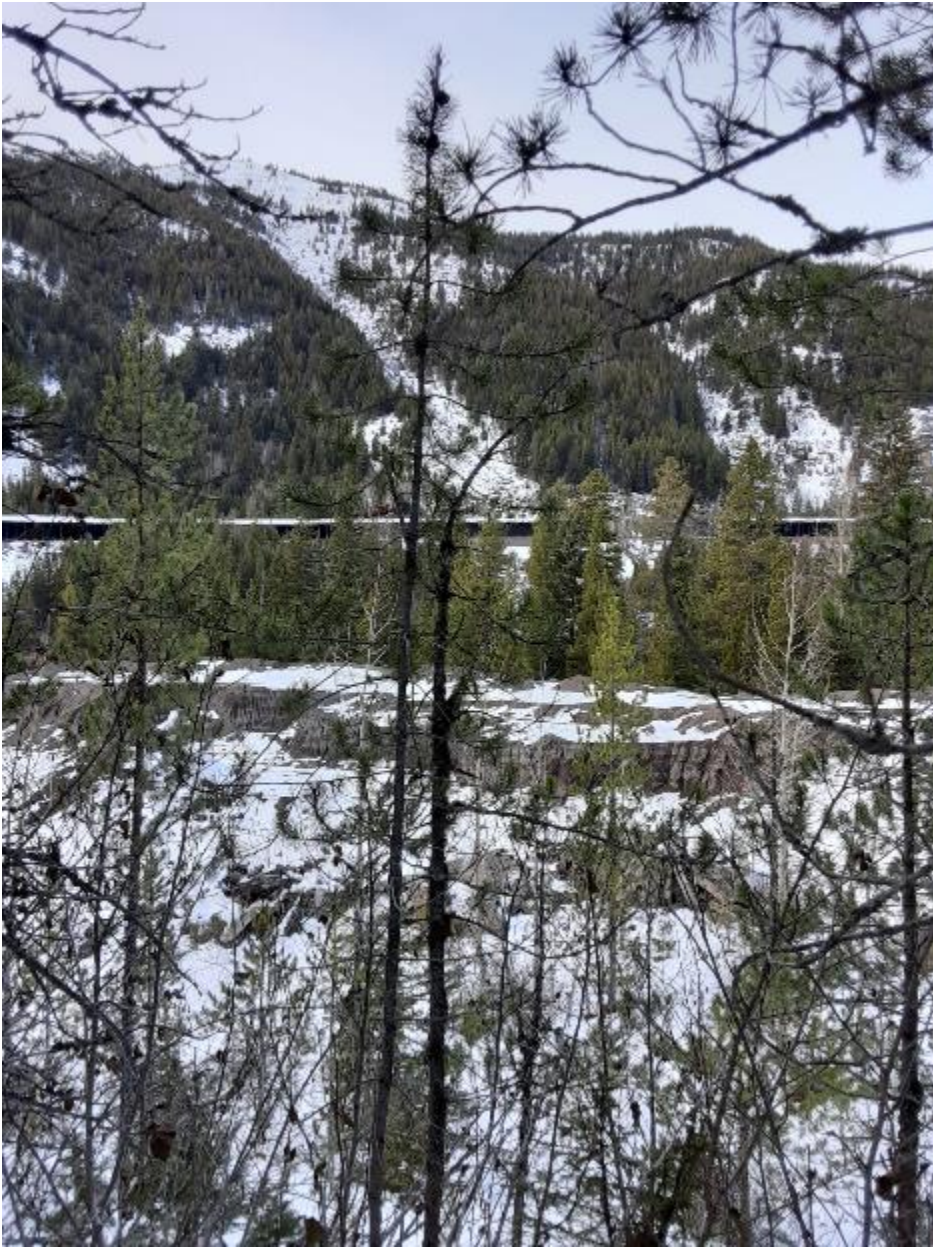
Site 3 - Picture of the railroad tracks with avalanche shed from Devil Creek- taken from U.S. Highway 2.
