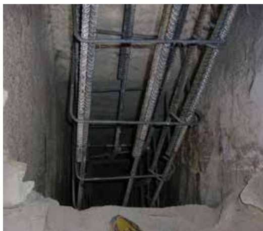
Reinforcing cage inserted into the full-height flue of the dining room chimney. Courtesy of Dan Cooke, JVA, Inc.
