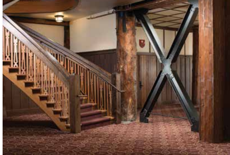
Braced frame in the basement level of the lobby. Courtesy of Mark Bryant Photographics.
