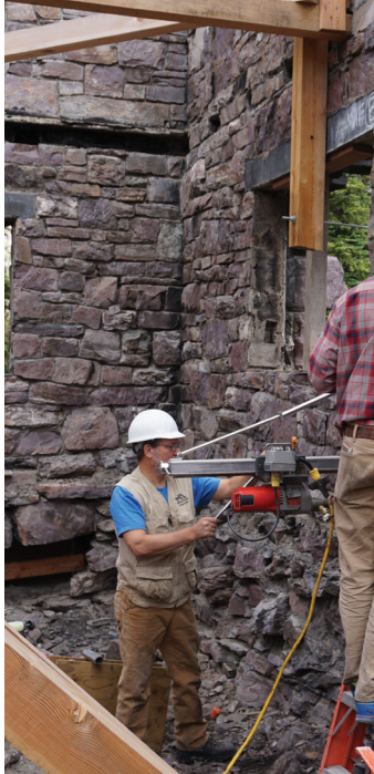
Figure 3. Engineers core-drill the masonry wall.
