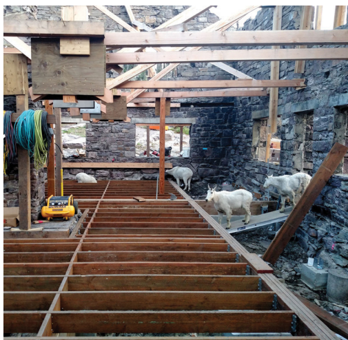
Figure 4. The first floor is framed as interior bracing is progressively removed.
