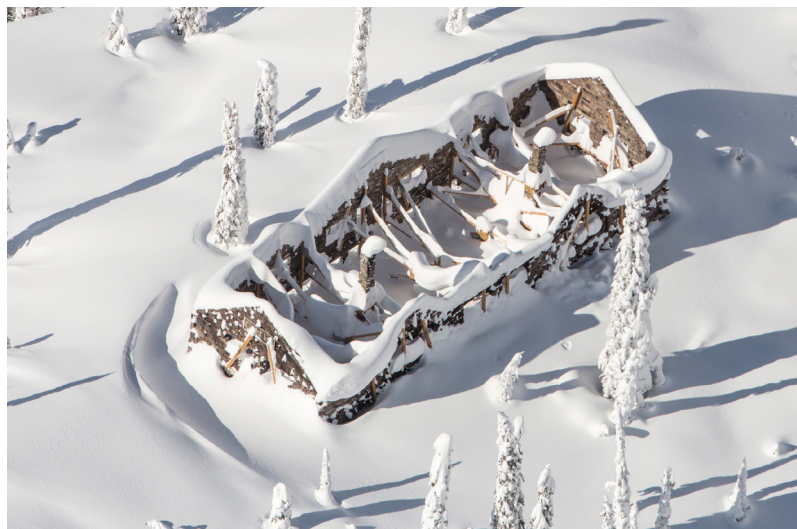
Figure 1. The chalet survives the first winter after the fire, thanks to emergency bracing. Courtesy of GravityShots.com.
