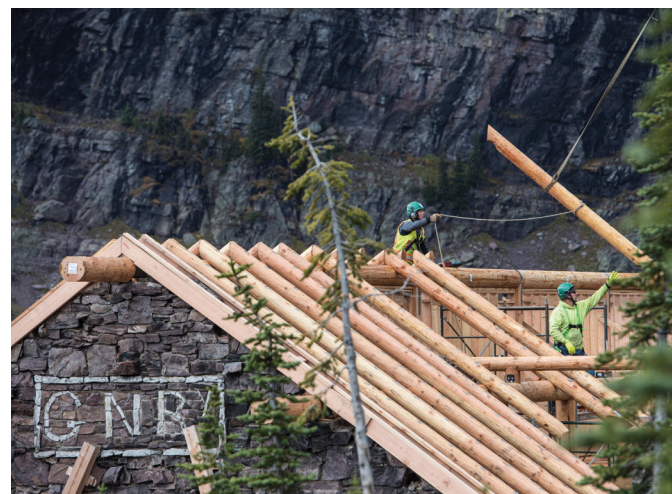
Figure 5. Timber framers set the log rafters via helicopter assist. Courtesy of A Boring Photo.
