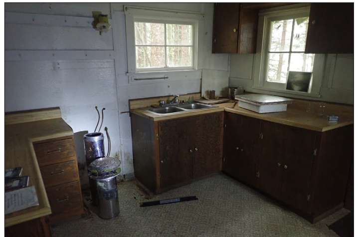
Figure 5.31: The kitchen casework including a vacant space for a stove and the double-basin kitchen sink. The casework likely dates to the 1980s but is still serviceable.
