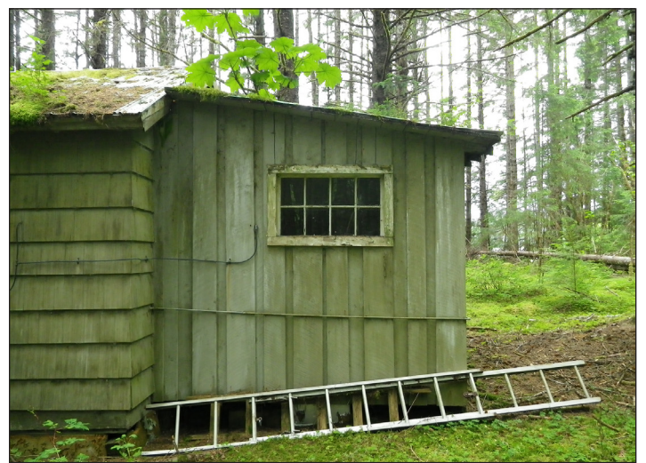
Figure 5.15: The only 8-lite fixed, wood sash window is located on the south elevation of the Shed Addition in Room Three.
