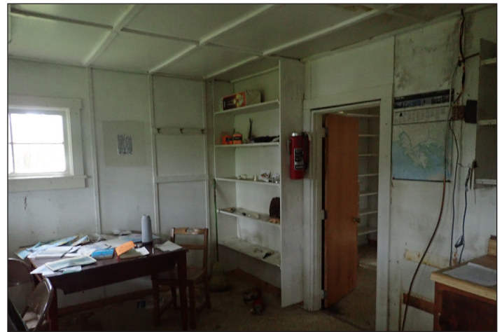
Figure 8.20: The kitchen casework may not be original to the cabin but is in serviceable condition.
