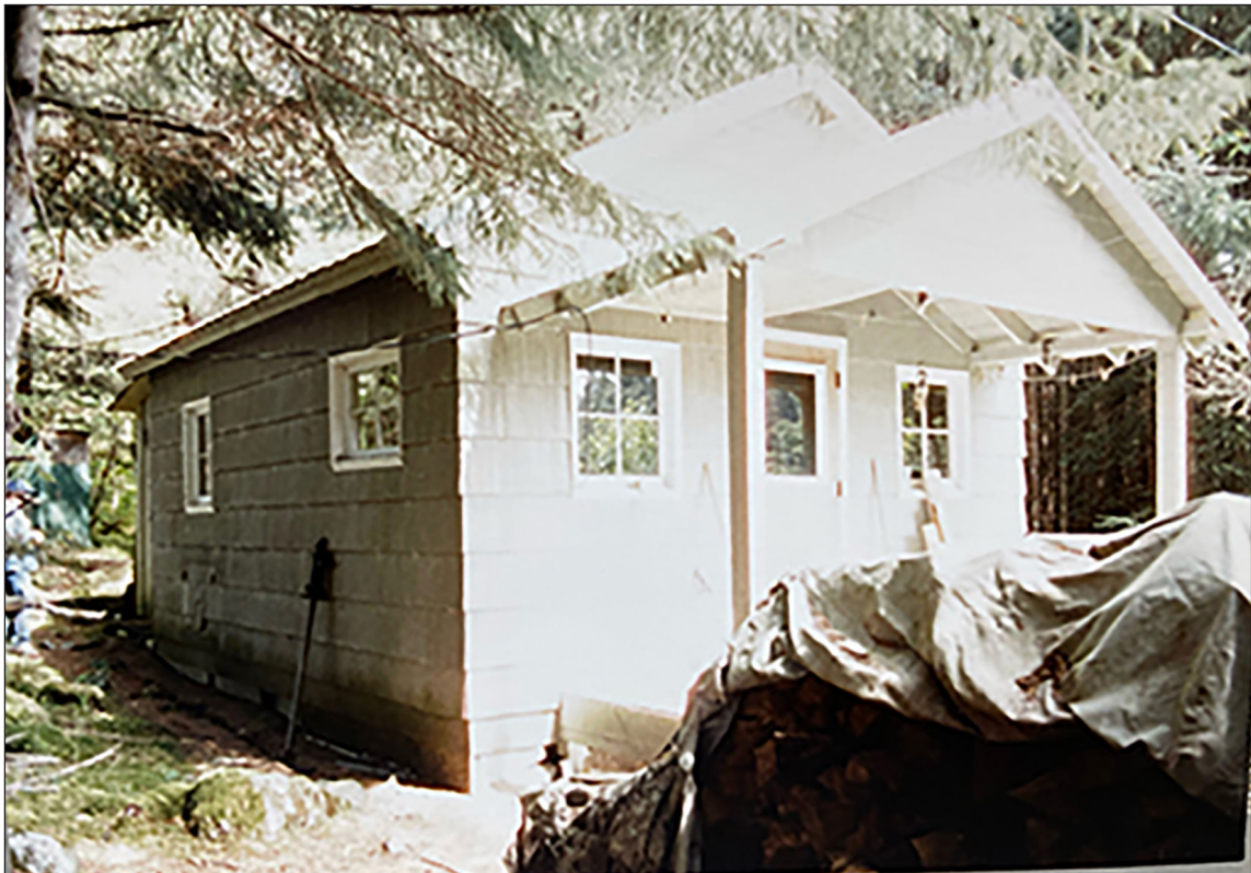
Figure 4.8: Another photo found in the Alaska Region Facility Management files from the 1990s illustrating the Lagoon Island Cabin from the northwest. Alaska Region Facilities Files. NPS Photo.
