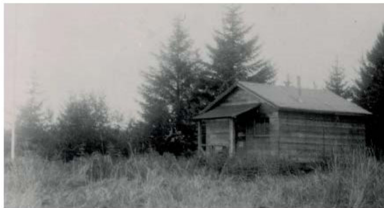
Figure 10: Southwest and southeast elevations, view towards north. No windows were extant on the southeast elevation, and the porch had a shed roof. 1951, NPS photo.
