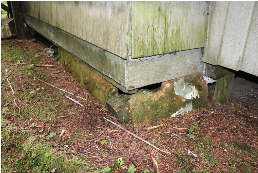
Figure 8.1: Detail of the northeast corner of the Lagoon Island Cabin's foundation which is comprised of untreated post and pad configuration. The 1 ½" x 5 ½" floor joists are oriented east-west, perpendicular to the roof ridge, and cantilever 2'-0" beyond the primary 12 7/8" square foundation beams. The reason is unknown but may be attributed to the relocation effort.
