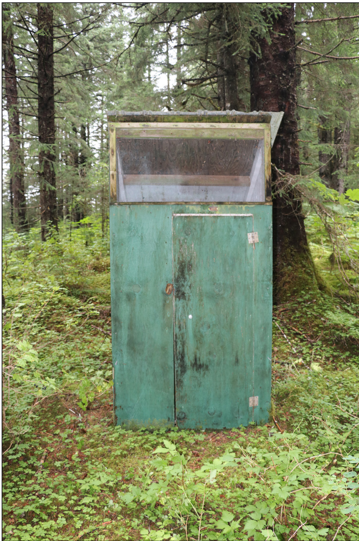
Figure 5.35: South elevation of the shed roofed outhouse.
