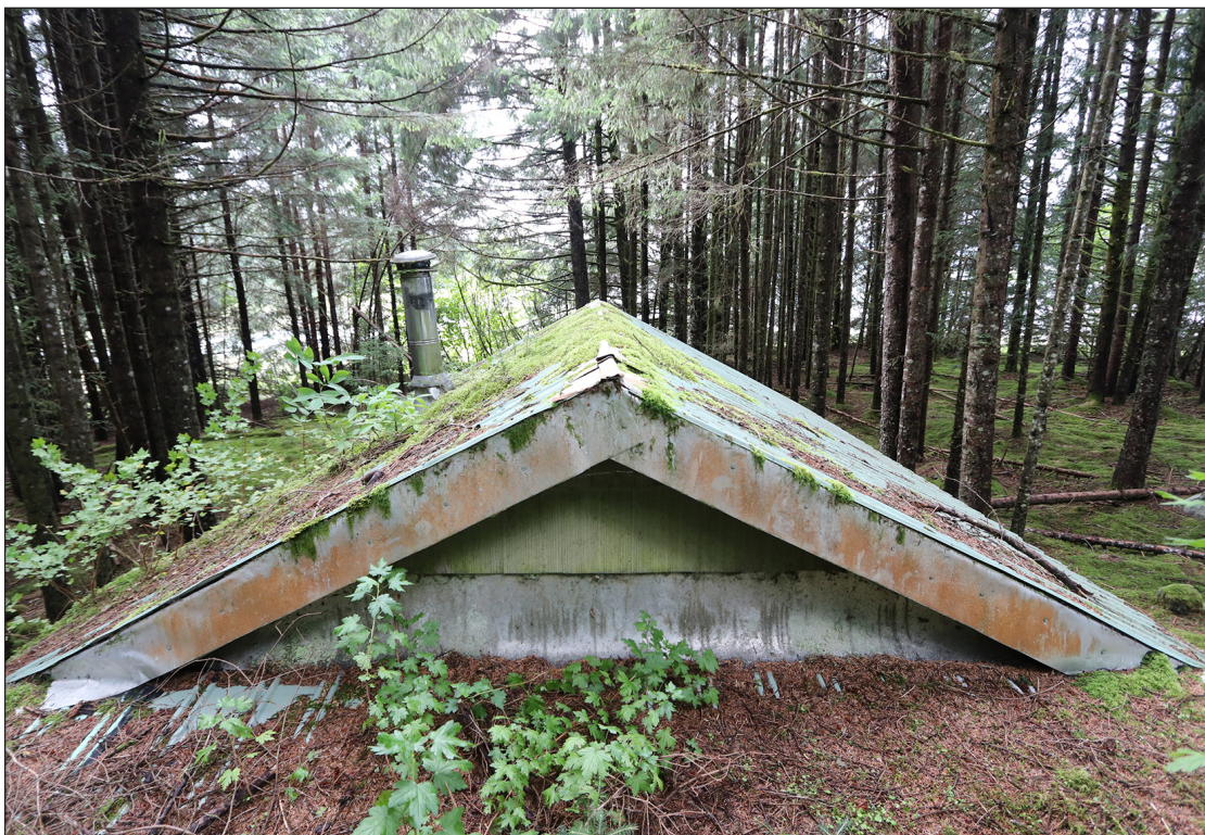
Figure 5.8: View looking south where the addition's shed roof joins the main gable roof. Note the metal fascia flashing on the gable end of the cabin roof. The roof was covered in vegetation and duff during the 2018 inspection. The park cleaned the roof off in the fall of 2018.
