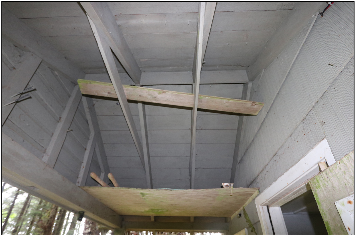
Figure 5.18: View of the porch roof and enclosed gable framing.
