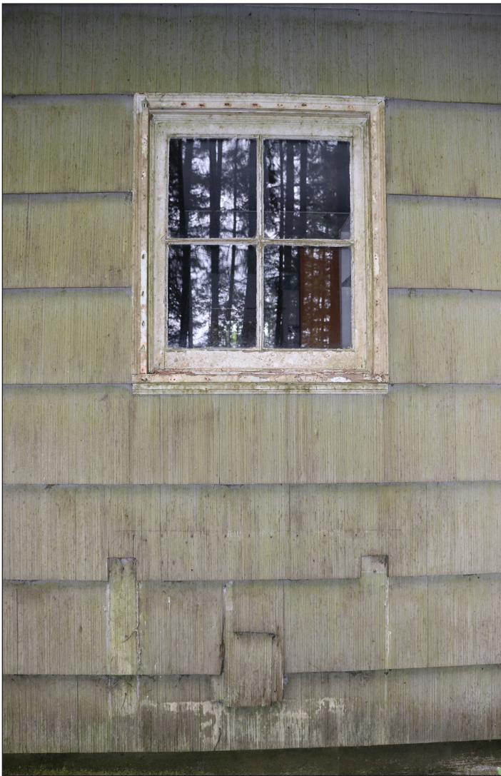
Figure 5.13: The cabin includes six 4-lite, fixed, wood sash window and one 8-lite fixed, wood sash window. The windows remain intact, are well placed and proportional to the small cabin.
