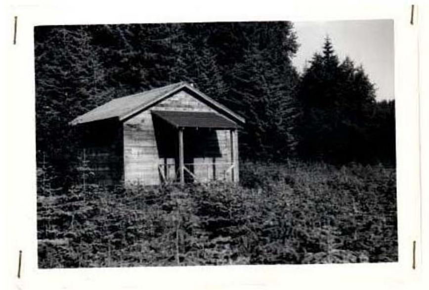
Figure 9: Southwest façade, view towards northeast. 1951, NPS photo.
