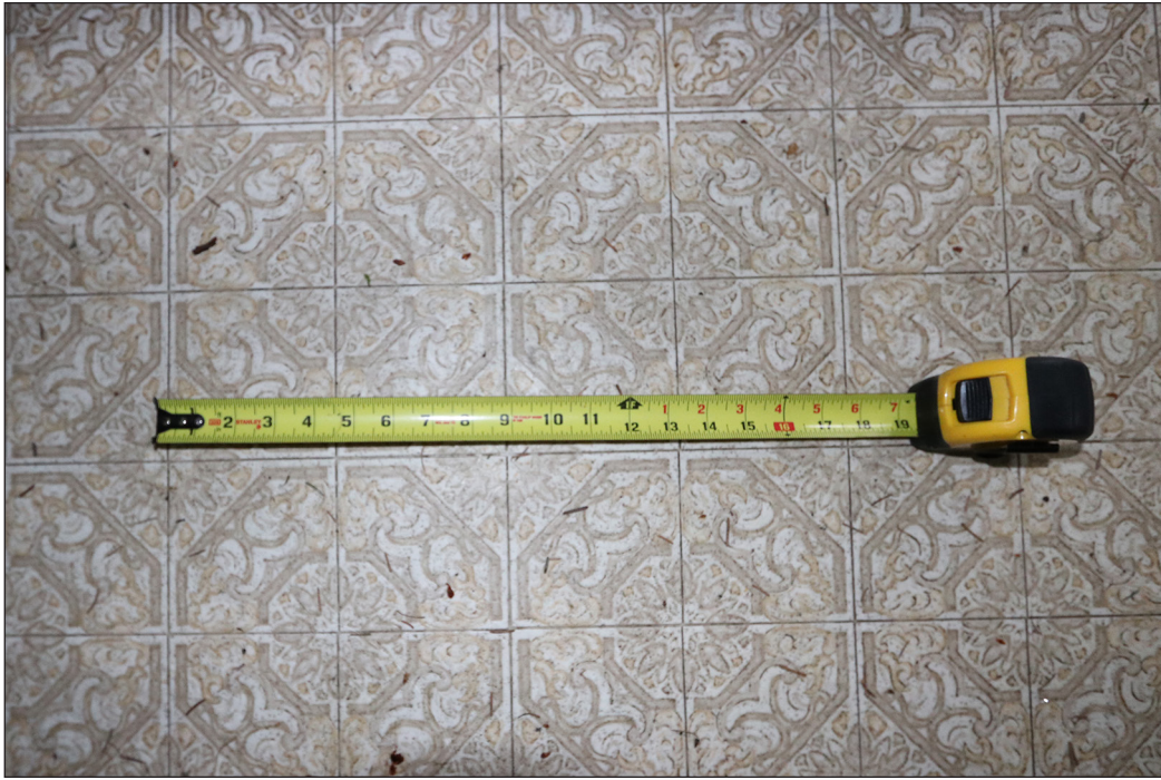
Figure 8.3: The flooring in Rooms One and Two is comprised of a sheet linoleum which is in fair condition.
