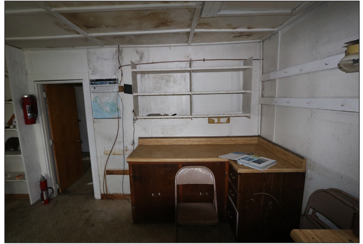
Figure 5.29: Existing shelving and casework on the east interior wall of the kitchen in Room One.
