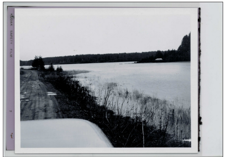
Figure 4.6: View of the Lagoon Island Cabin across Bartlett Cove along a roadbed that no longer exists. The date of this photograph is unknown but likely the 1970s. GLBA Archives, Accession # 00491, Box 6, Folder 6 GLBA 10885.
