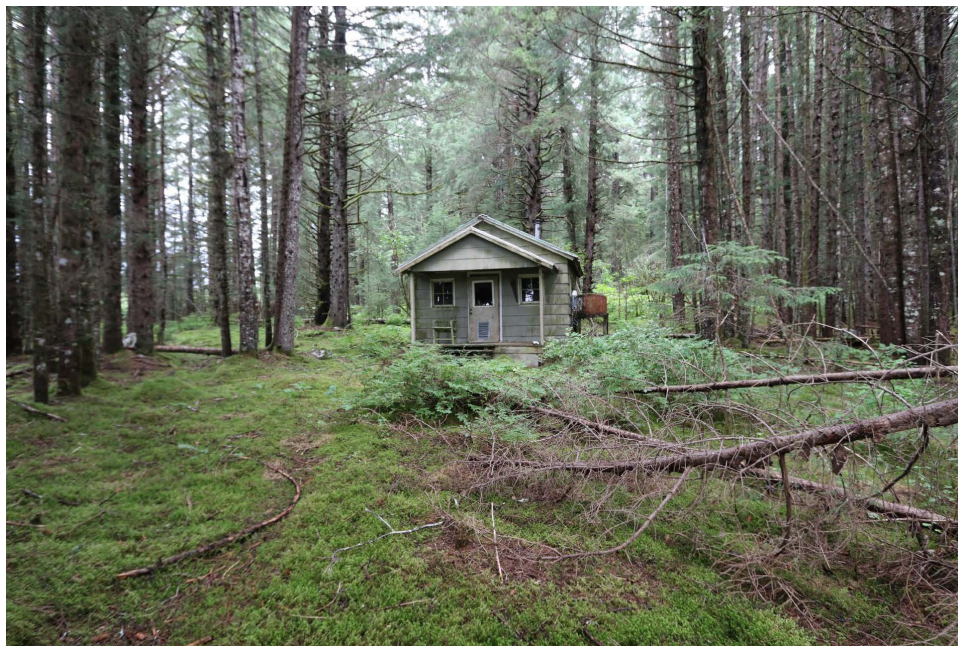
Photo 1: Overview of Lagoon Island Cabin, Toward Northeast, 2018.
