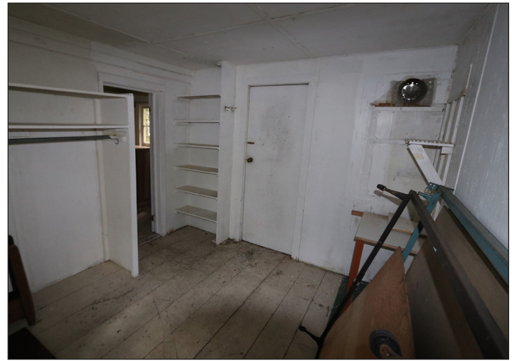
Figure 5.12: Interior view of the door providing exterior access from Room Three.
