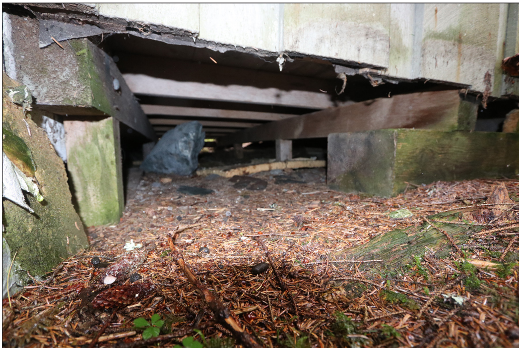
Figure 8.2: Detail photo of the shed addition foundation from the south elevation.
