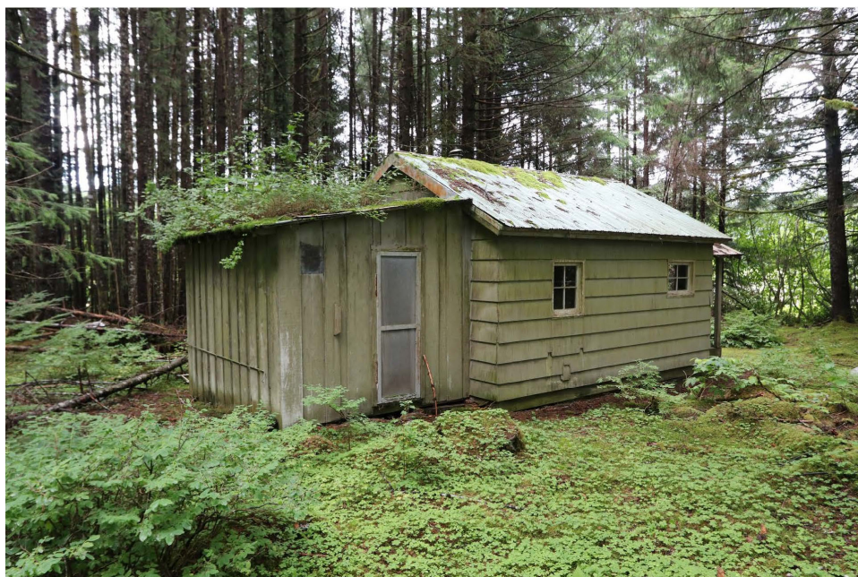
Photo 6: Lagoon Island Cabin, Toward South, 2018.
