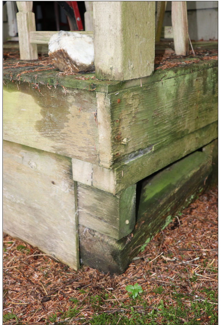
Figure 8.16: Detail view of the cabin's porch foundation at the southwest corner.
