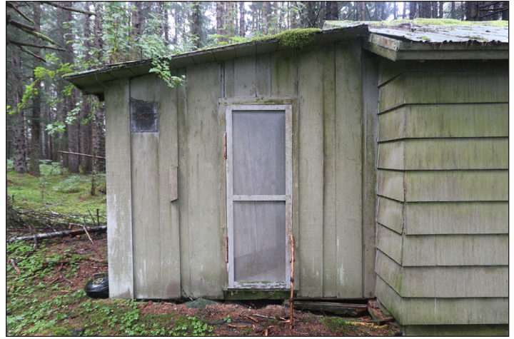
Figure 5.11: The shed roof addition (Room Three) has an exterior door on the north elevation which is a solid core door with a screen door.
