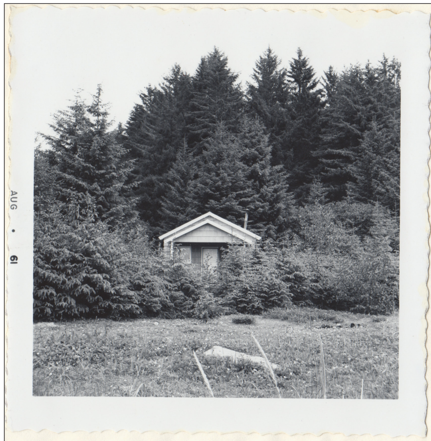
Figure 4.3: Another 1961 view of the Lagoon Island Cabin from the southeast illustrating the small, shed roof porch, only one window and a stove pipe protruding from the roof's east elevation. The cabin is set in an open meadow of beach grass with the coniferous taiga forest behind. GLBA Archives, Accession # 00491, Box 6, Folder 6 GLBA 10885.
