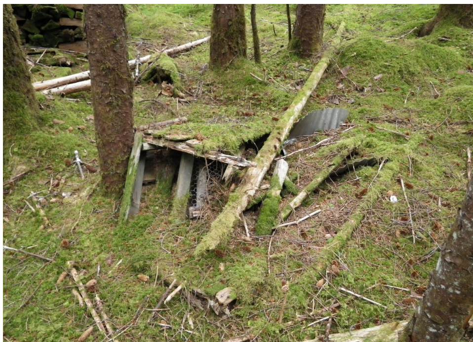
Photo 14: The auxiliary shed ruins, a non-contributing site, 2013.
