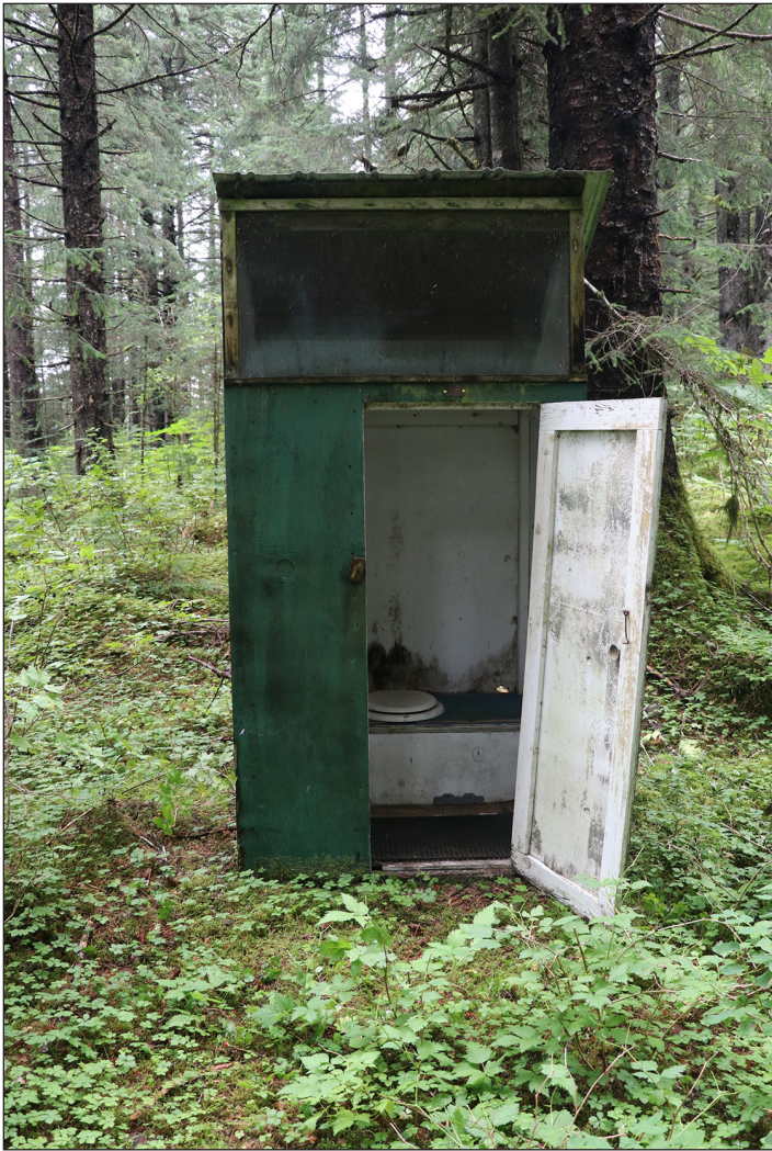
Figure 8.24: South elevation of the existing outhouse which is no longer in use.
