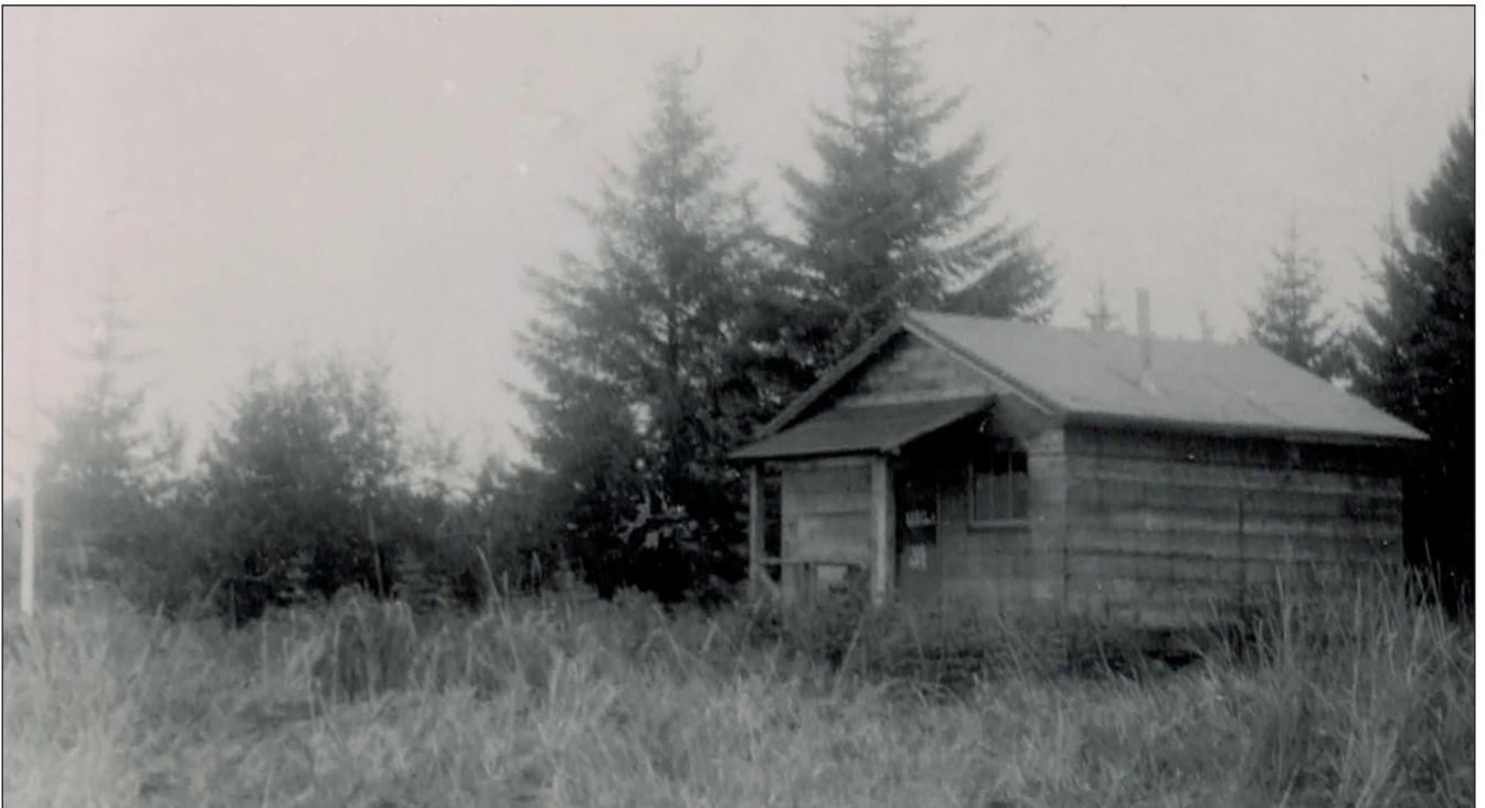
Figure 3.3: This 1951 image of the Lagoon Island Cabin was taken from the southwest and illustrates the cabin with the small, centrally located shed roof porch and bare wood horizontal sub sheathing. The roof appears to be clad in cedar shingles and the windows on the south elevation have not been installed. GLBA Archives, Accession # 00491, Box 6, Folder 6 GLBA 10885.
