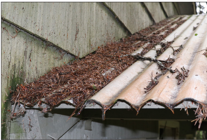
Figure 8.8: The forested environment deposits considerable duff throughout the year as seen here at the junction of the porch roof west gable wall of the cabin.
