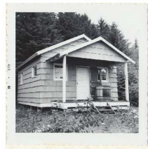
Figure 12: Southwest façade, view towards northeast. New windows installed include two on the façade and two to the northwest elevation. The porch has been converted to a gable roof. 1961, NPS photo.
