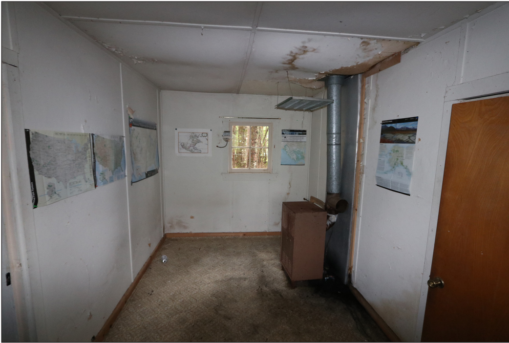
Figure 5.23: View of the south interior elevation of Room Two.
