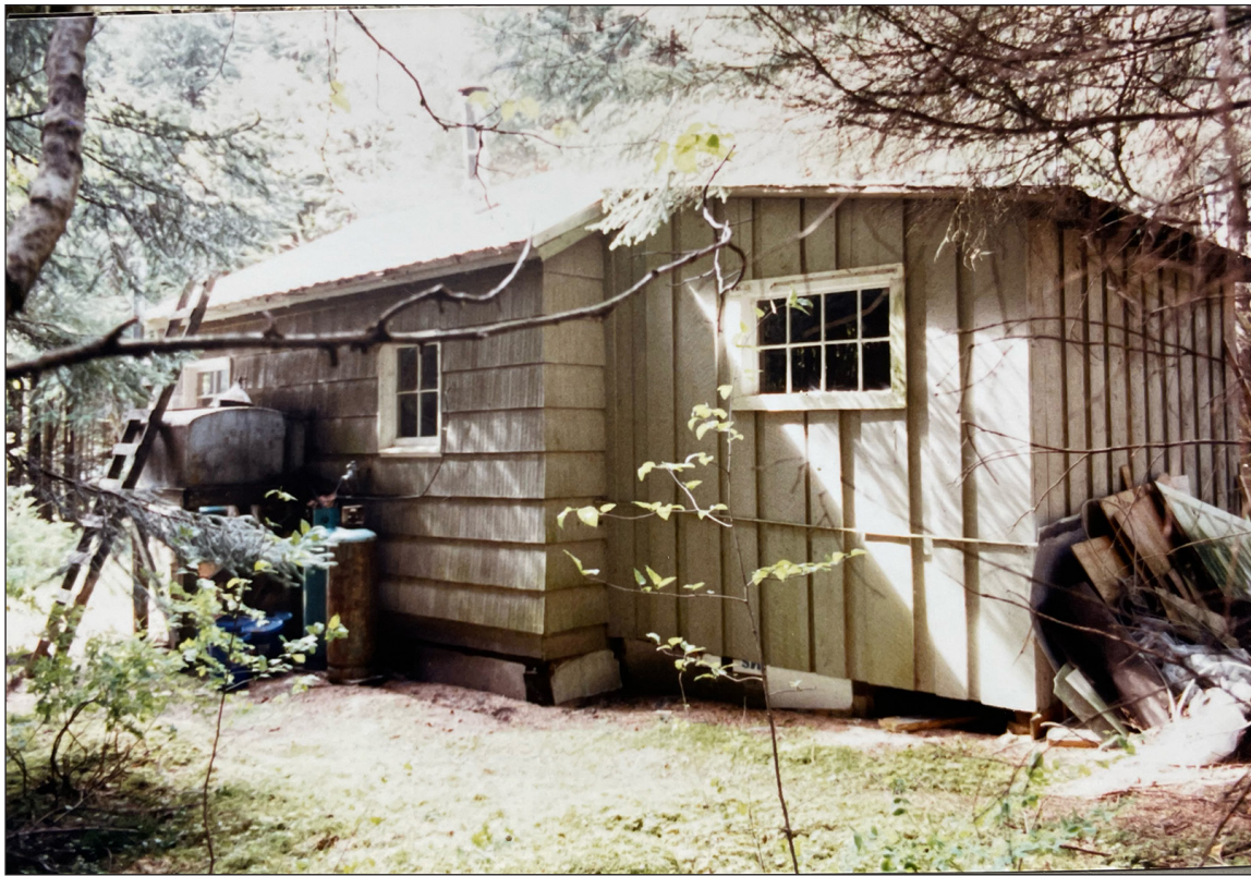
Figure 4.9: View from the southeast of the Lagoon Island Cabin dating to the 1990s. Alaska Region Facilities Files. NPS Photo.
