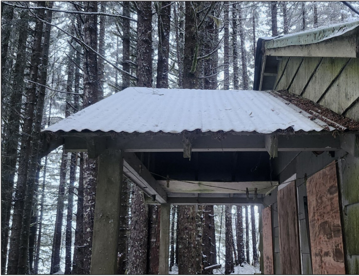
Figure 8.14: View of the south elevation of the porch roof.
