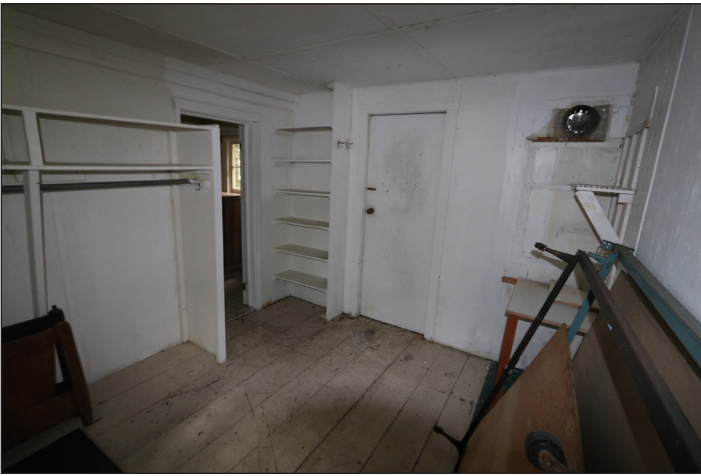
Figure 5.25: Northwest interior perspective of Room Three.
