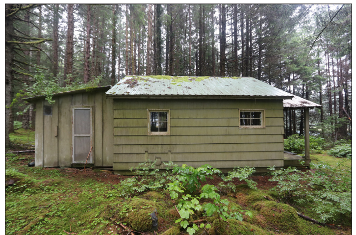
Figure 5.14: The 4-lite windows are used in a vertical and horizontal configuration as seen on the cabin's north elevation.
