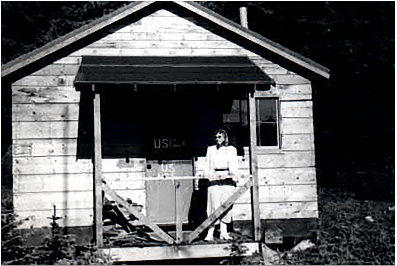
Figure 3.2: Closeup view of the Lagoon Island Cabin from 1951 with an unidentified visitor standing on the shed roofed porch with a diagonal braced railing. Note the small coniferous trees sprouting around the cabin. National Archives, Record Group 79 Box 292, Glacier Bay National Monument.
