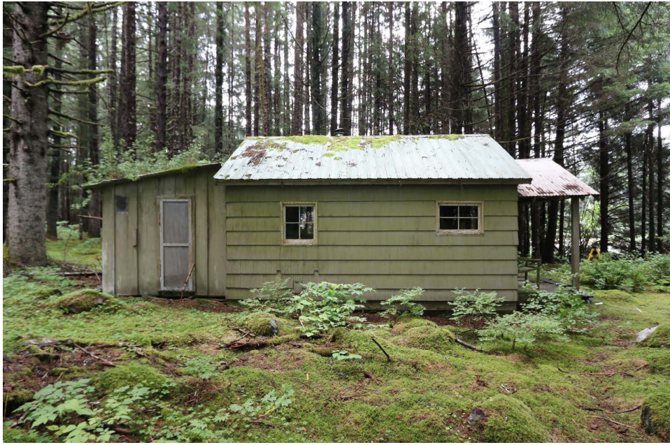
Photo 7: Lagoon Island Cabin, Toward Southeast, 2018.
