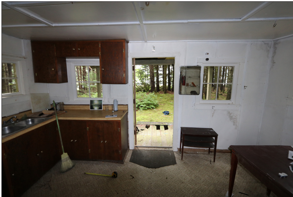
Figure 5.20: View of the west interior elevation of Room One with the cabin's primary entry.
