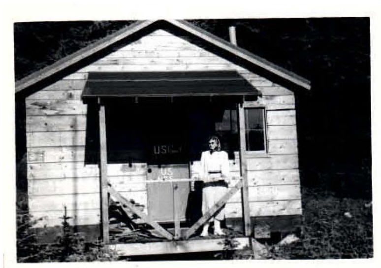
Figure 8: Southwest facade, view towards northeast, showing only one window and a door with U.S. government markings. 1951, NPS photo.
