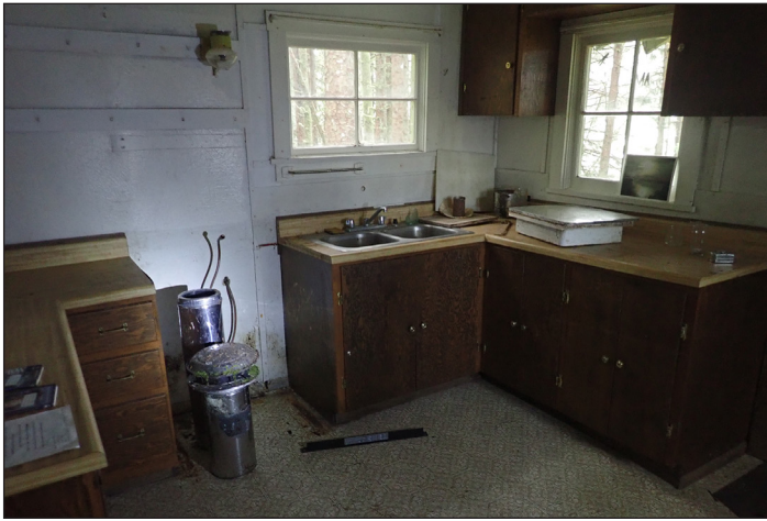
Figure 8.17: The kitchen casework may not be original to the cabin but is in serviceable condition.
