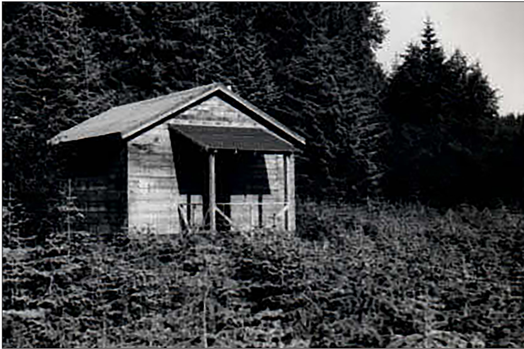
Figure 3.1: View of the Lagoon Island Cabin in August 1951. The majority of exterior Character Defining Features remain intact contributing to the cabin's high degree of integrity. Note the five-panel wood door which is likely original and the foundation lacking a skirting. GLBA Archives, Accession # 00491, Box 6, Folder 6 GLBA 10885.
