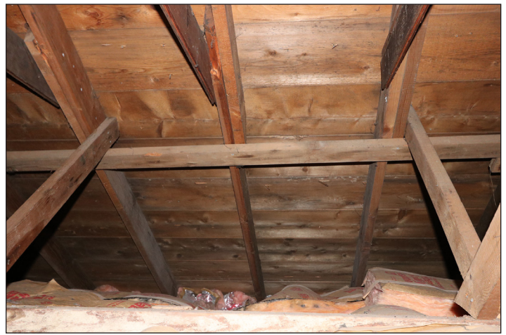
Figure 8.7: View of the roof framing from the attic access hatch in Room One. The ceiling is insulated with fiberglass batt. The attic is dry with no rot concerns.
