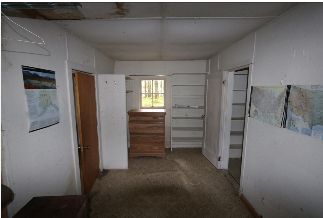
Figure 5.24: View of the north interior elevation of Room Two.
