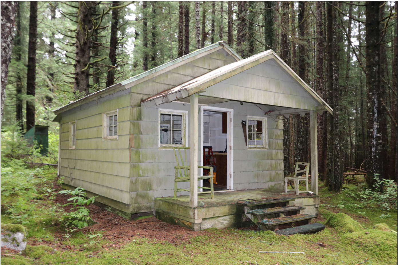
Figure 1.1: Perspective view of the Lagoon Island Cabin from the southwest.
