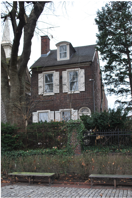
Figure 30. Rectory, east elevation, view looking west from the Swanson Street Forecourt. The rectory is set back from the forecourt plaza, historically South Swanson Street, making it less prominent in the original streetscape than the church, which is to the left of this view. It is now used as office space. (CLR 2022: 111)
