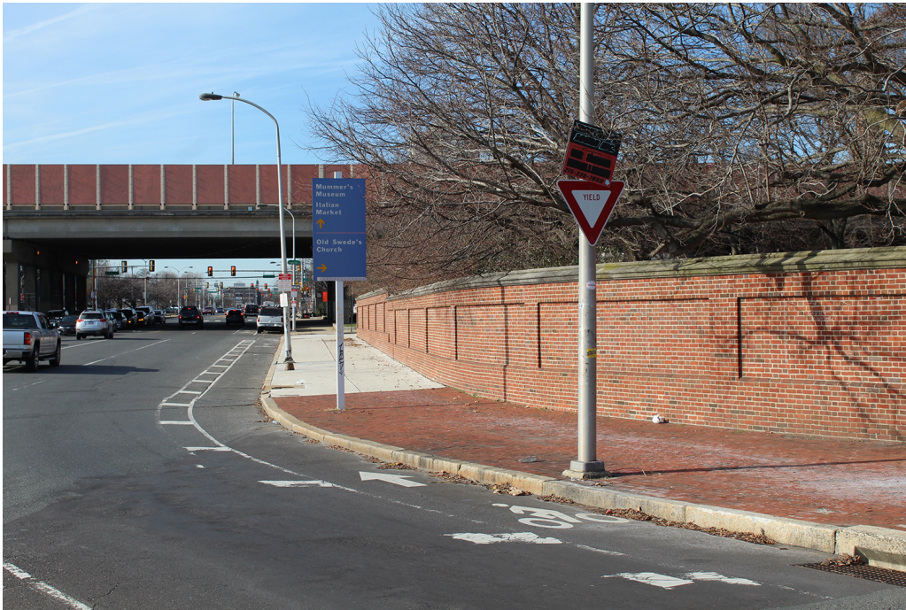
Figure 35. Perimeter wall section that is noncontributing, view looking west on Washington Avenue from Christopher Columbus Boulevard. Built in 1978-1979 by the National Park Service to enclose the property. Its design was intended to be compatible with an earlier wall of 1898 east of the burial ground (see Figure 33). (CLR 2022)
