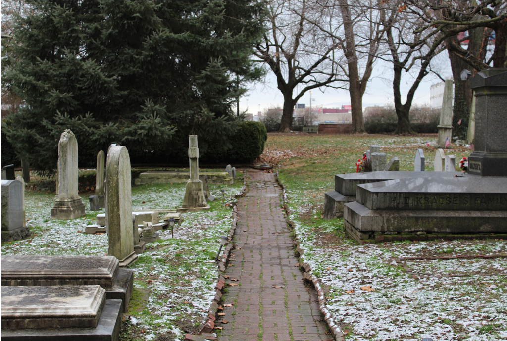
Figure 38. Burial ground, typical brick path conditions, view looking south from south of the sexton's house. (CLR 2022: 145)
