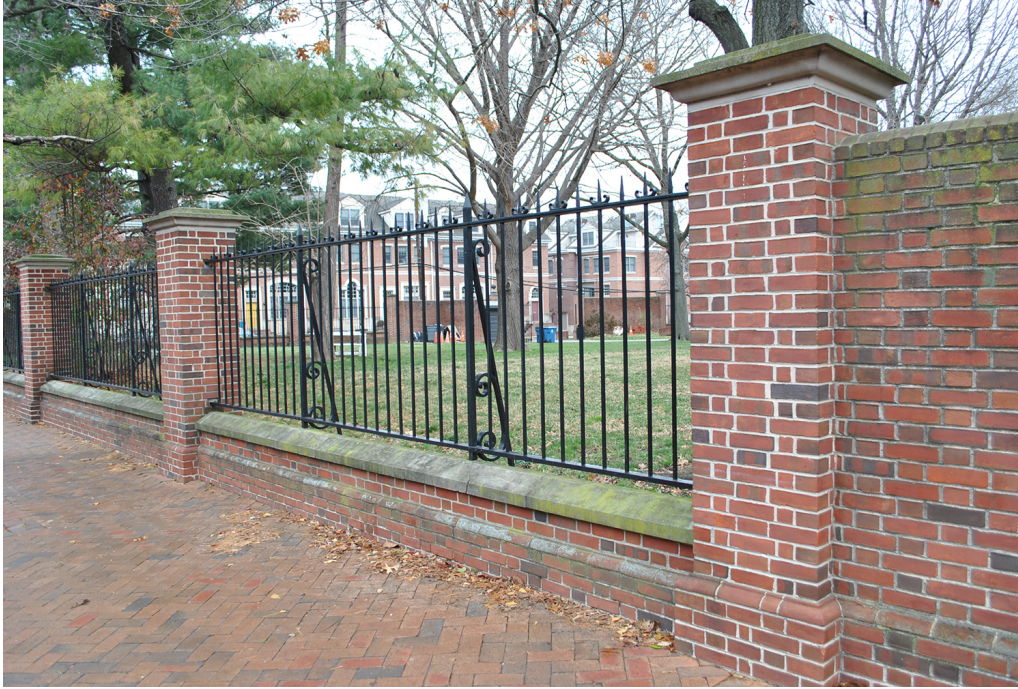
Figure 36. Perimeter wall and fence, view looking southeast on Christian Street from near South Water Street, built in 1978-1979 by the National Park Service to enclose the Gloria Dei property. Its design was intended to be compatible with the 1898 section east of the rectory (see Figure 34). (CLR 2022: 126)
