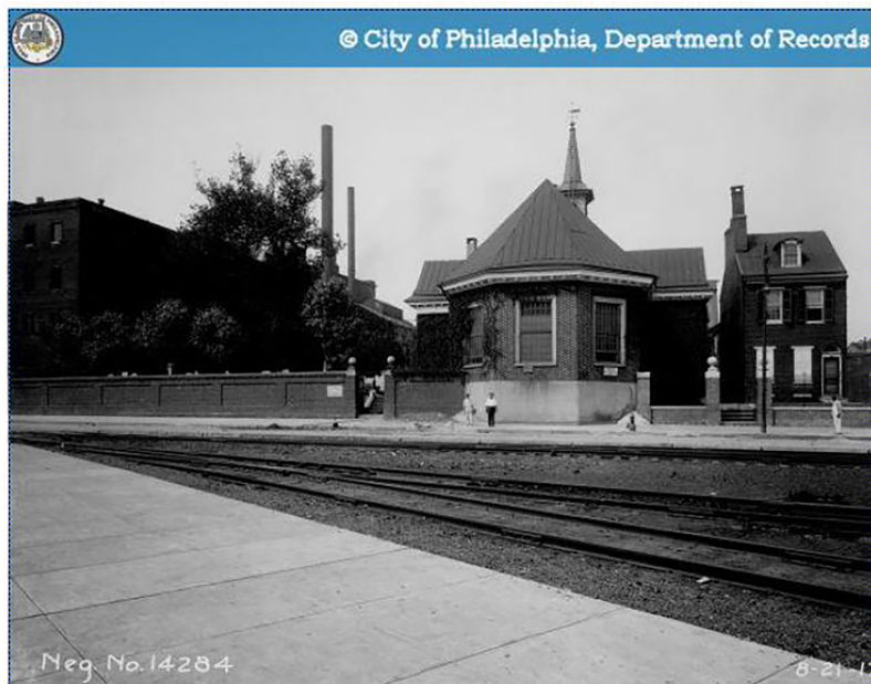
Figure 19. View west-southwest from South Delaware Avenue (present-day Columbus Avenue), 1917. Note proximity of the railroad tracks to the brick wall, gates, and fence erected along the church's Swanson Street frontage in 1898. Four young trees are growing on the burial ground side of the wall, apparently the four London plane trees extant today. (City of Philadelphia, Department of Records, #8401, from CLR 2022: 65)
