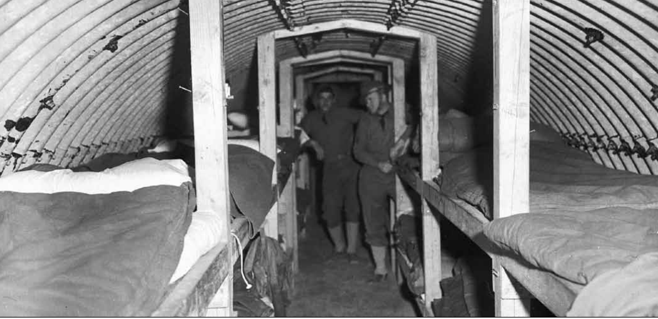
Once on high alert, Fort Cronkhite soldiers manned their guns around the clock. This photo shows the men's sleeping arrangements on Wolf Ridge, in a temporary corrugated metal shed, similar to a Quonset hut, built into the side of the hill. (Photo 1942)
