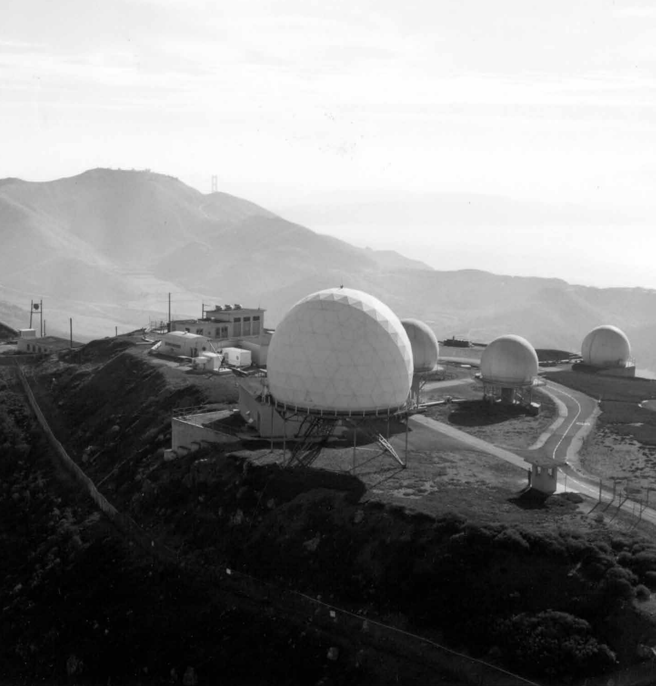
Above: The Integrated Fire Control radars at the Nike Site SF-88, atop Wolf Ridge, overlooking Fort Cronkhite. The role of this site was to watch for incoming enemy planes, track them as they approached the coast, plot their course and direct the Nike missiles to the planes' location all via radar. (Photo circa 1965)
