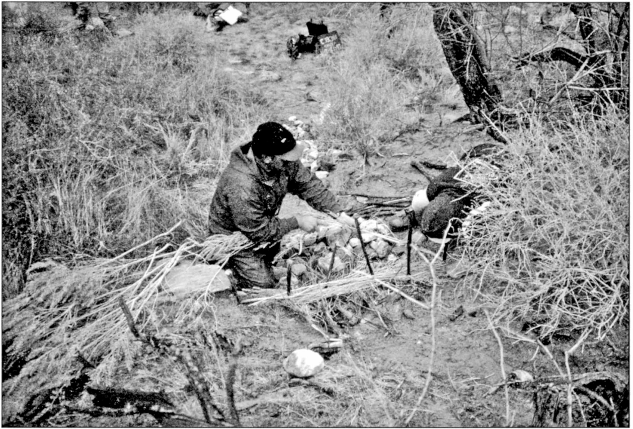
Figure 33. Soil conservation specialists from the Pueblo of Zuni installing erosion-control checkdams at site AZ C:13:381 (courtesy of Grand Canyon National Park Archaeology Program).
