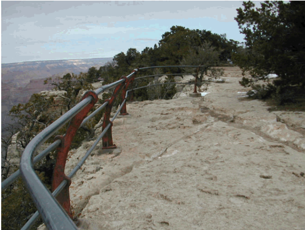
Metal railings at West Rim Drive overlooks were bent to fit the contours and topography along the canyon rim. (Photo by J. Galbraith, 2003)
