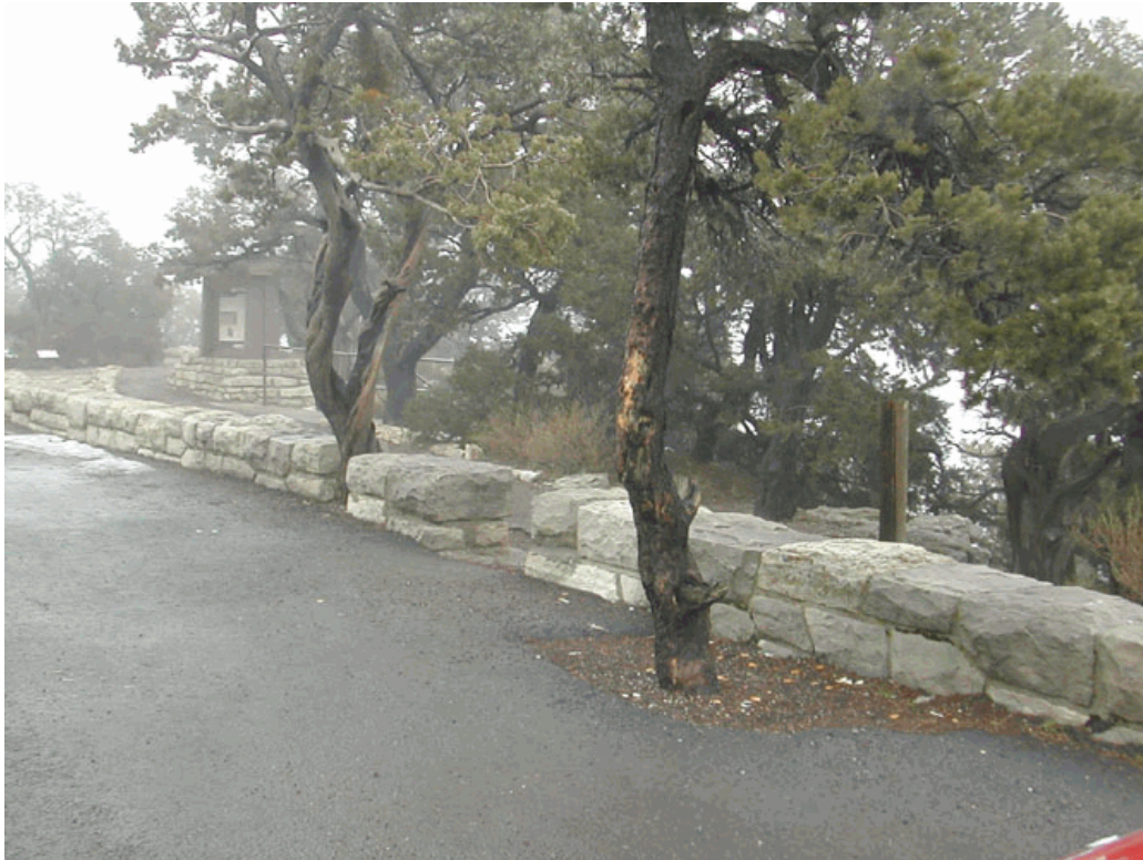
Example of paving and masonry walls incorporating existing trees at a West Rim Drive overlook. (Photo by J. Galbraith, 2003)
