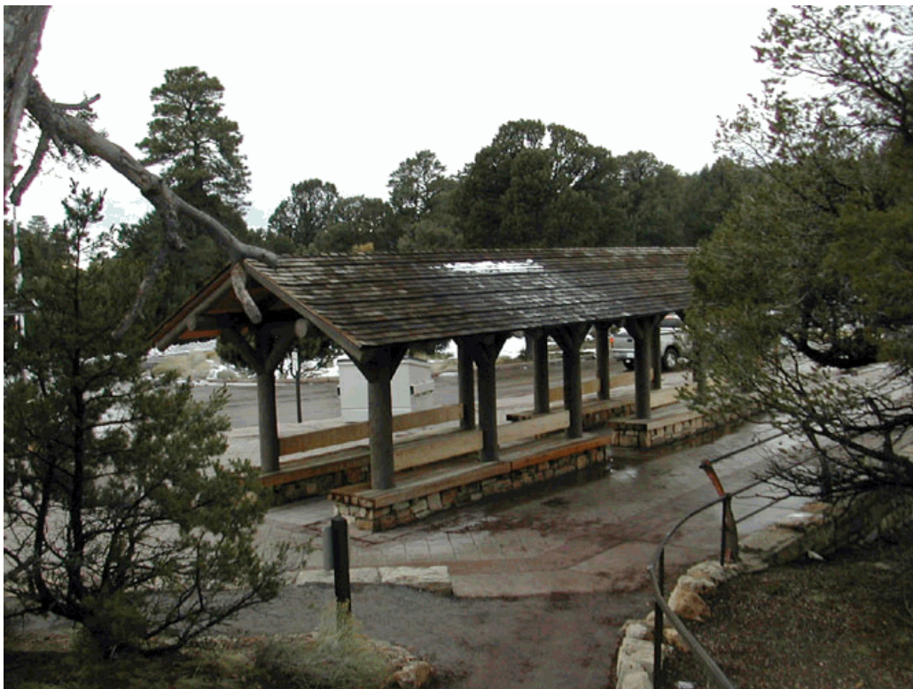
Shuttle stop at the entrance to the West Rim Drive and Trail. (Photo by J. Galbraith, 2003)
