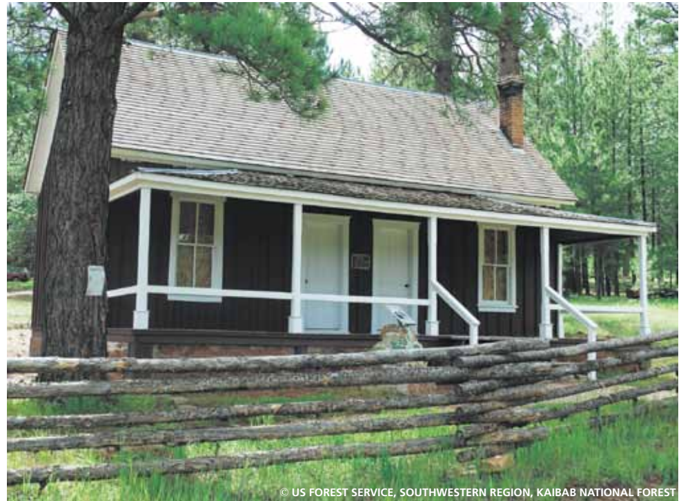
Jacob Lake Ranger Station, built in 1910, connects us with the beginning of the US Forest Service and stands today on its original site near Jacob Lake.
