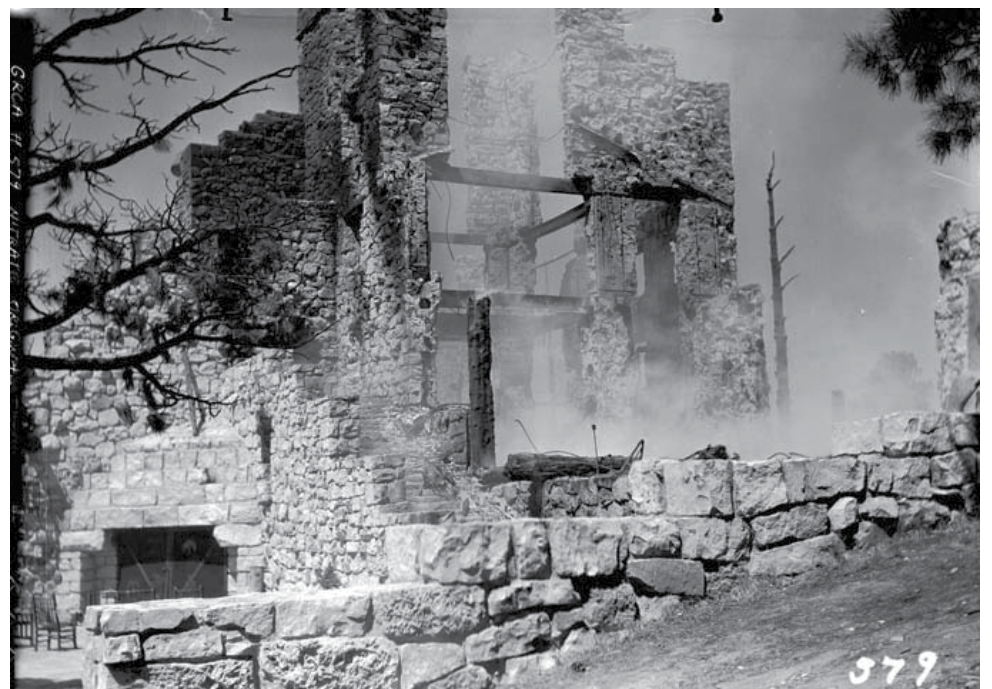
The original Grand Canyon Lodge's outside fireplace and stairwell smolder in ruins after being destroyed by a kitchen fire in 1932.
