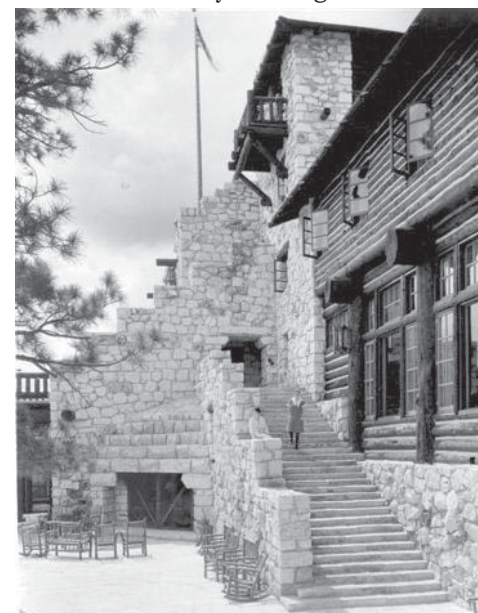
A view of the back porch, stairway, and patio of the Grand Canyon Lodge in 1930.
