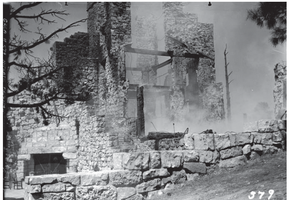
The original Grand Canyon Lodge’s outside fireplace and stairwell smolder after being destroyed by a kitchen fire in 1932.
