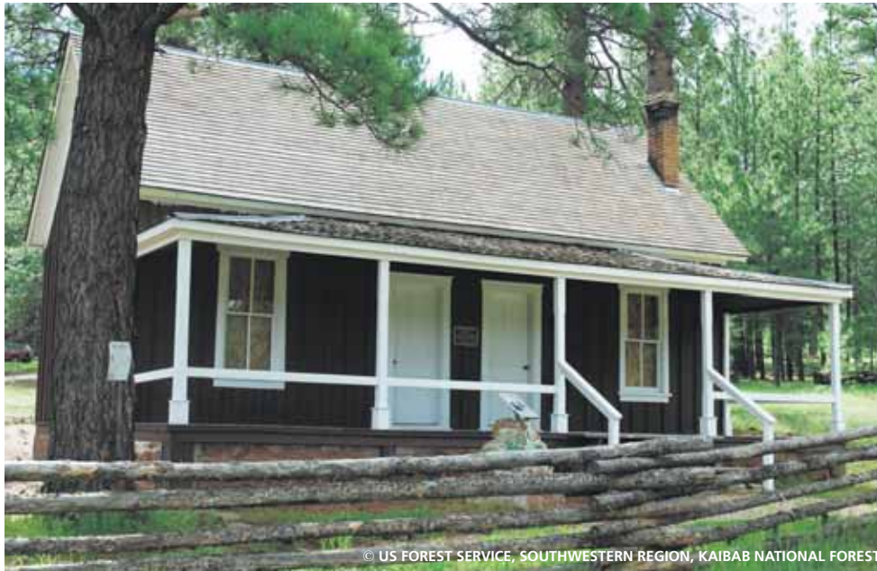
Jacob Lake Ranger Station, built in 1910, connects us with the beginning of the US Forest Service and stands today on its original site near Jacob Lake.
