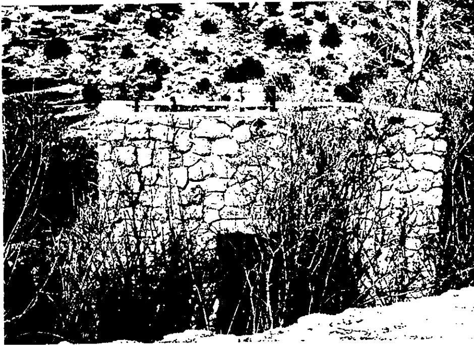
Figure 12. Pumphouse below the junction with the Tonto Trail, facing northwest. (#20)
