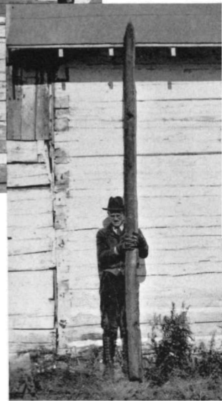
Above: Original picket and tie pole, showing method of fastening pickets together.
