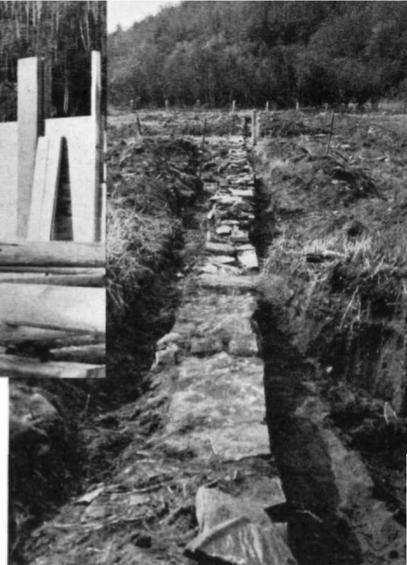
Original foundation of main hall, 95x30 feet.
