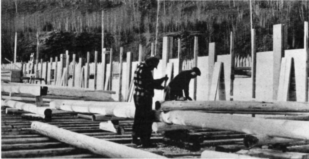
Rebuilding the main hall, December 1939. Note the palisade.
