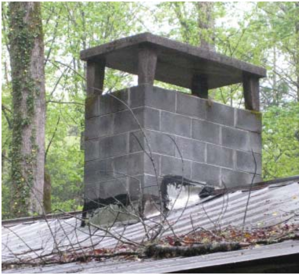
Figure 21, C. 1970 concrete block chimney.
