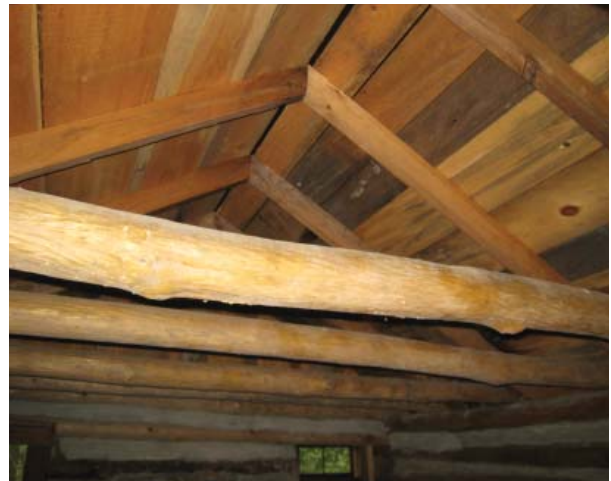
Figure 74 , Open framing above main room of Adamless Eden.
