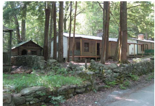
Figure 2, View towards Adamless Eden and Addicks Cabin with river stone retaining wall along Daisy Town Road.
