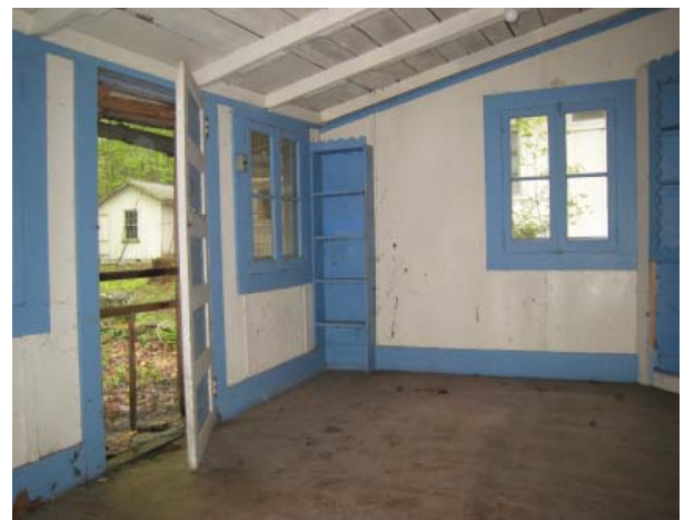
Figure 55, Southeast oblique of dining room, Room 106.
