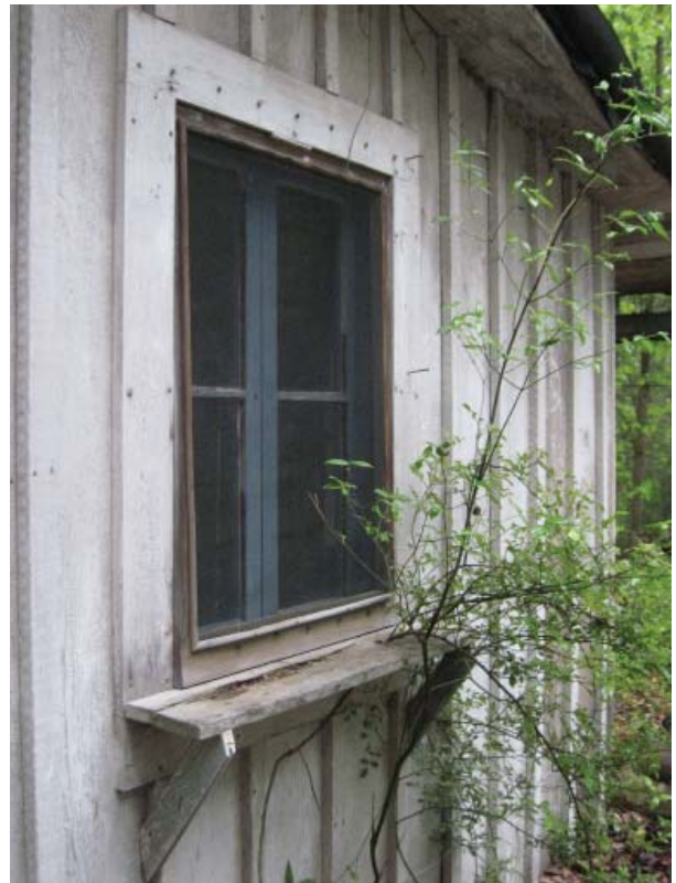
Figure 26 , Casement window and window shelf at southeast dining room.
