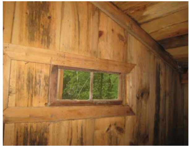
Figure 73 , Small sliding-sash window at Adamless Eden's bathroom.
