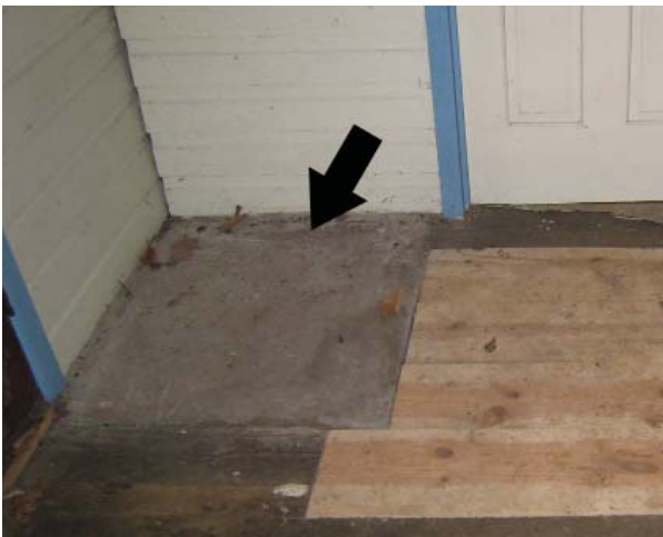
Figure 19 , Concrete pad in kitchen floor, presumably for a hot water heater.
