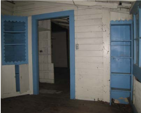
Figure 56 , North wall of dining room looking through doorway into kitchen, Room 107.
