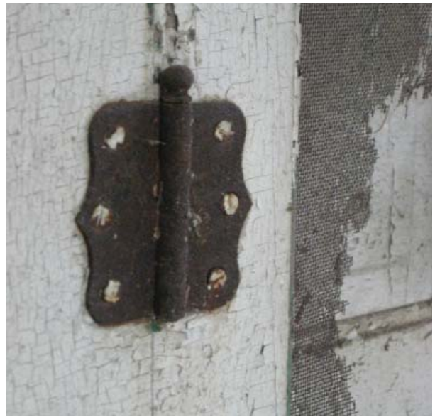
Figure 33, Original scalloped-edge ball-pin hinges at all three front elevation screen doors.
