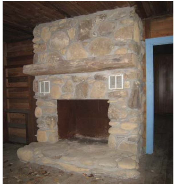
Figure 49, Fireplace at south wall of living room.
