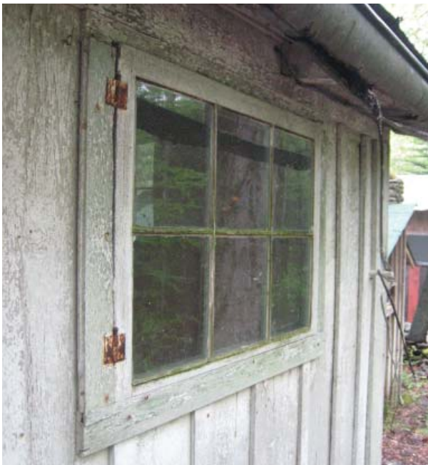
Figure 28 , Casement window at bathroom.
