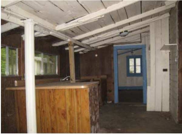
Figure 16, Kitchen with four generations of rafters.
