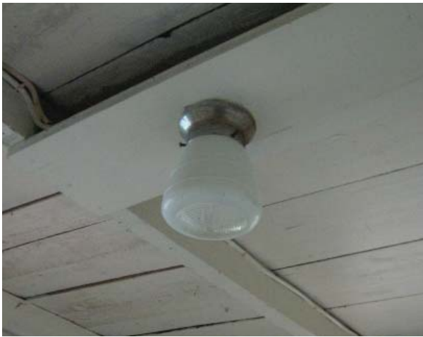
Figure 67, C. Mid-twentieth century ceiling light fixture in the northeast bathroom.
