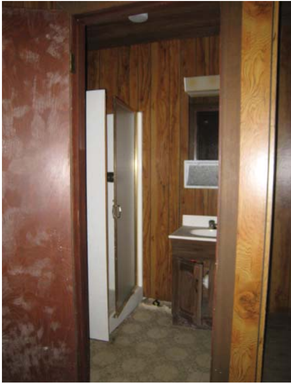
Figure 54, Fiberglass shower stall and base cabinet in master bathroom, Room 105.
