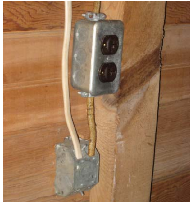
Figure 43 , Mid-twentieth century outlets at south wall.
