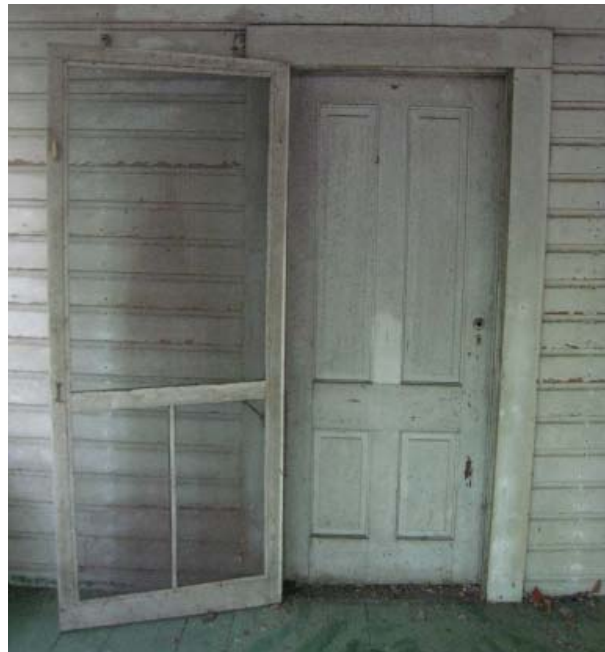
Figure 22, Early four-panel entrance door typical of west elevation.
