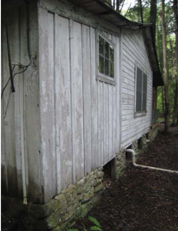
Figure 10, Board-and-batten siding of bathroom at northeast corner of cabin.
