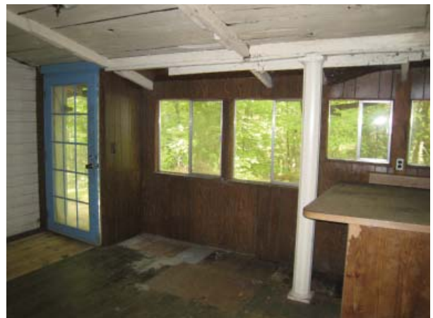
Figure 60, Northeast oblique of kitchen, Room 107.
