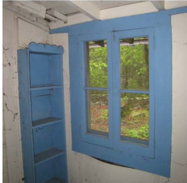
Figure 57 , Typical casement window and scallop-trimmed shelving in dining room.
