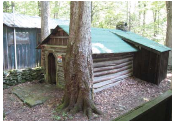
Figure 69, View of Adamless Eden from Addicks Cabin's front porch. The bathroom wing extends to the right.
