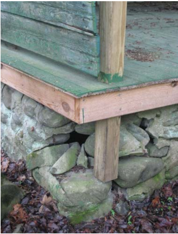
Figure 77 , Temporary shoring of front porch.
