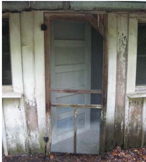
Figure 23, Five-panel rear entrance door at dining room, Room 106.
