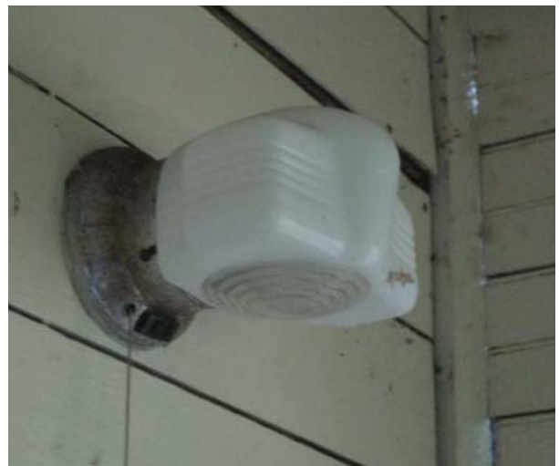
Figure 66, Light fixture above lavatory.
