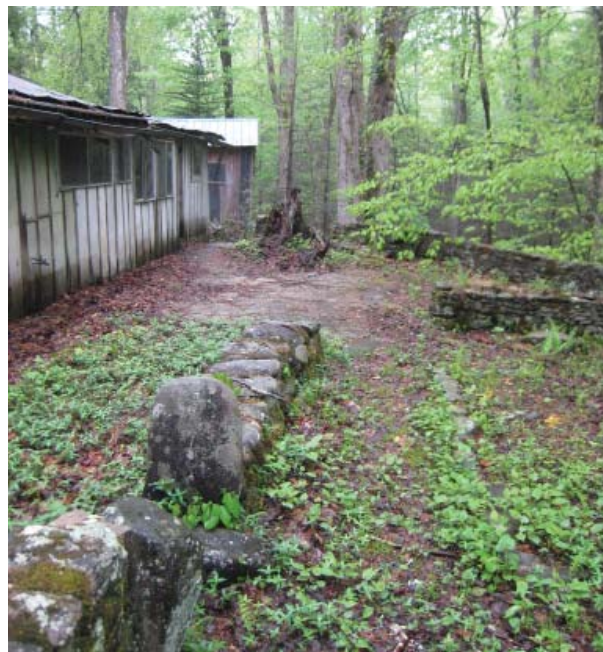
Figure 5, View of river stone walls, planters and flagstone patio on east side of cabin.
