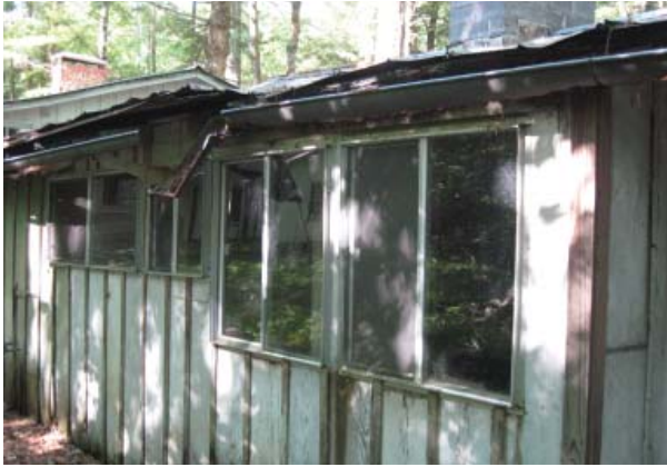
Figure 27 , Aluminum sliding-sash windows at east elevation of kitchen.
