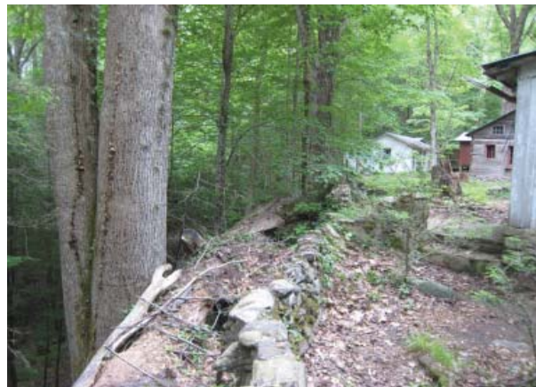
Figure 4, Stone retaining wall at back edge of property.
