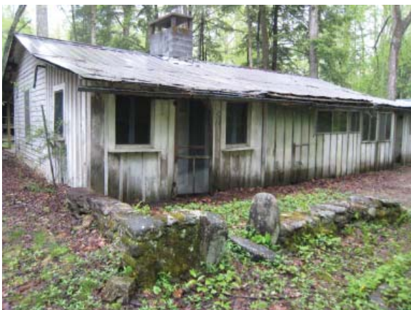
Figure 11, Southeast oblique view of cabin.
