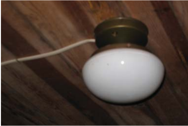
Figure 44, Ceiling light c. 1970.
