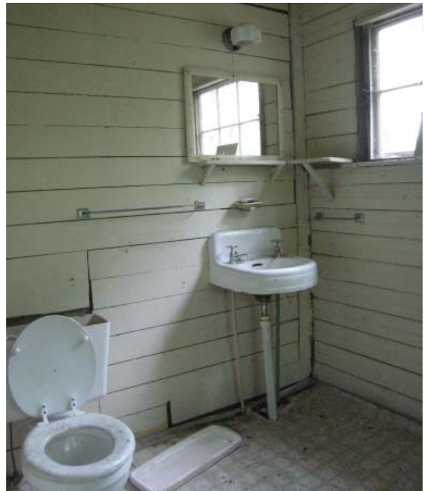
Figure 20 , Room 108 northeast bathroom with c. 1920 fixtures.
