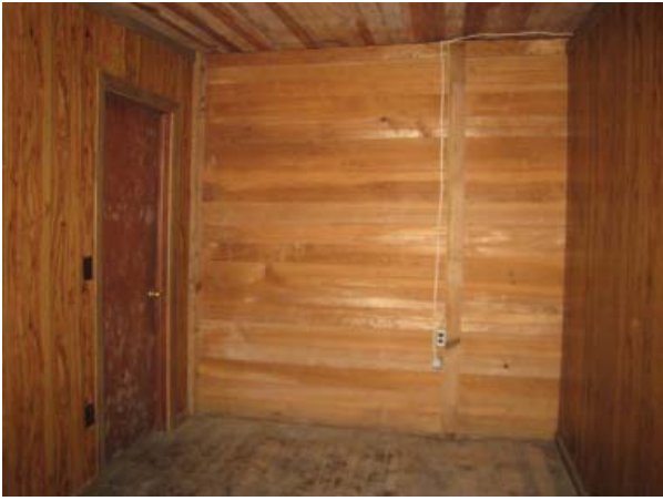
Figure 41 , View looking south in Room 102, North Bedroom. Modern c. 1970 veneer paneling on east and west walls plus flush-panel door on east wall.
