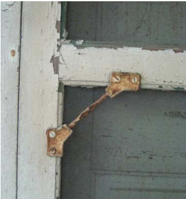
Figure 32, Original cast-metal screen door brace, typical of three front doorways.
