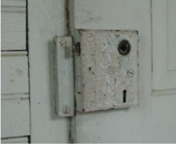
Figure 63, Original rim lock of northeast bathroom door.
