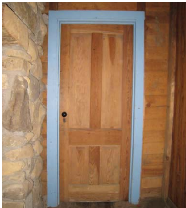
Figure 36, Typical four-panel interior door of main block.
