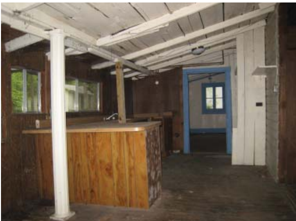
Figure 59, Southeast oblique of kitchen and dining room, Room 106, beyond.
