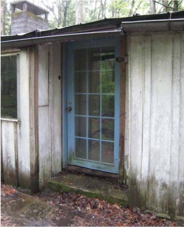
Figure 24 , C. 1970 fifteen-light door at kitchen, Room 107.
