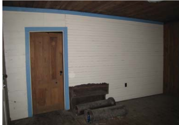
Figure 47, North wall of living room with early 5¼" boards applied horizontally.
