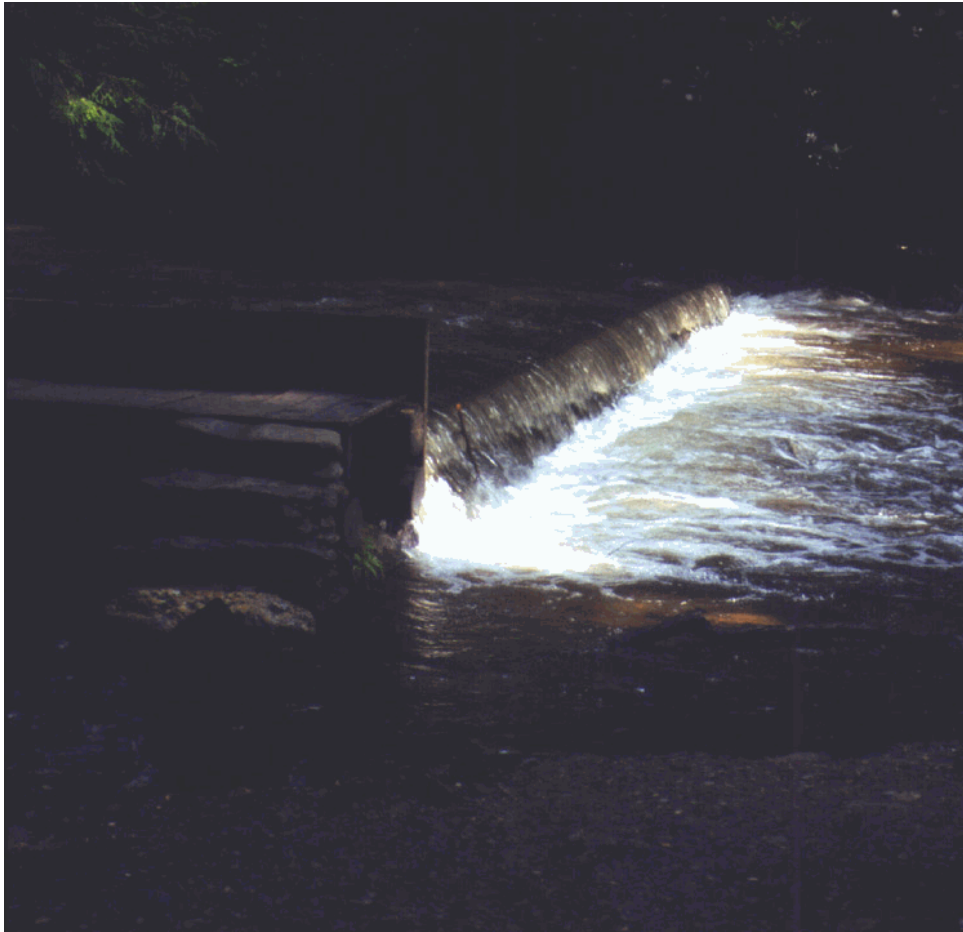
Point where water is diverted from Forge Creek to Mill Creek (2000)
