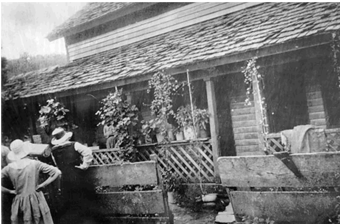
Figure 1. 1915 view of the Becky Cable House
