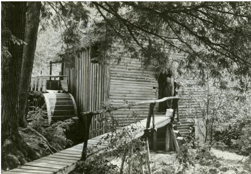
Figure 2. John P. Cable Overshot Mill following restoration (c.1937)
