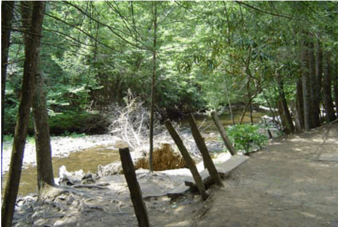
Hillside erosion and collapse of the fence line behind the drive-in barn (2006).
