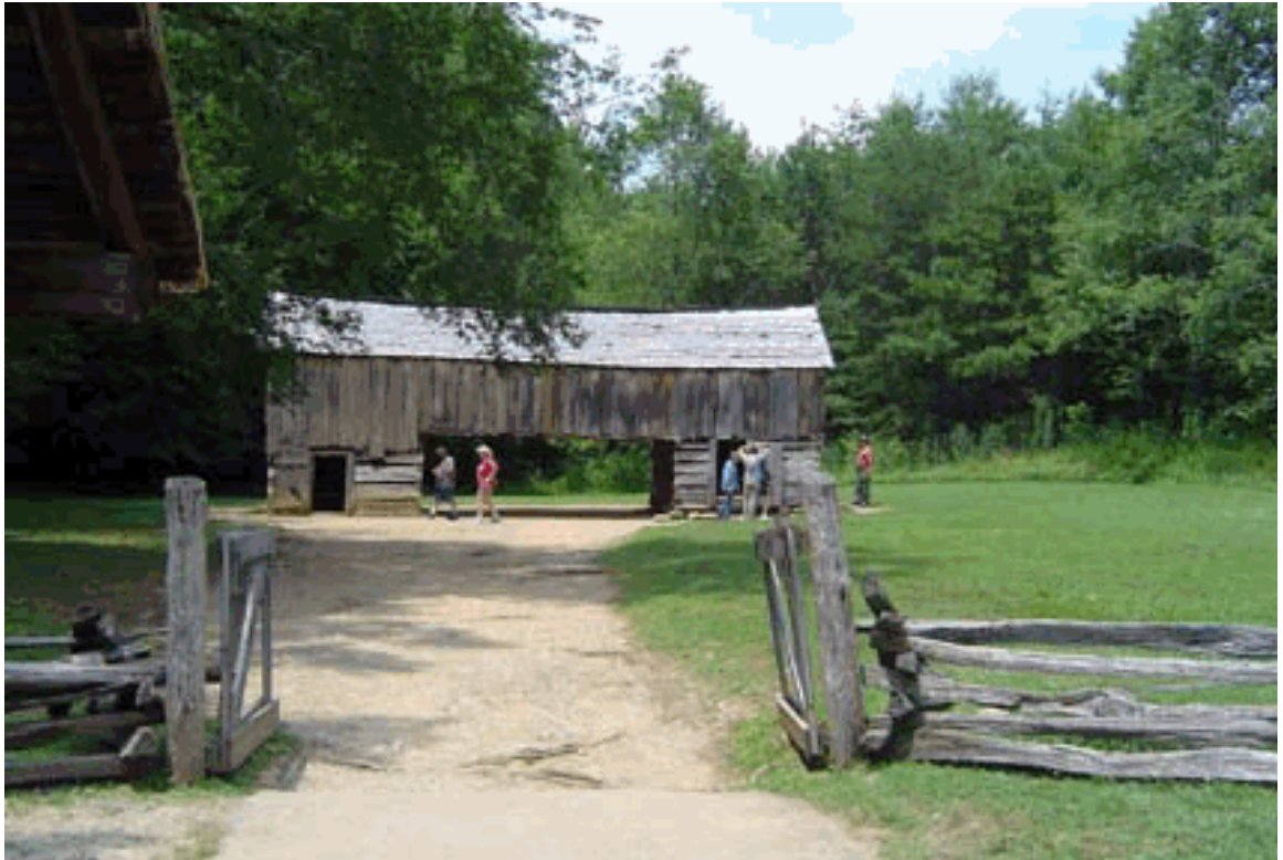
Slight erosion along pathway to barn behind the Becky Cable House (2006).
