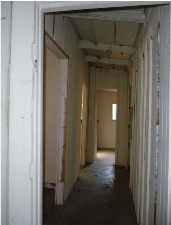
Figure 97. Hallway (Room 109a) looking south.
