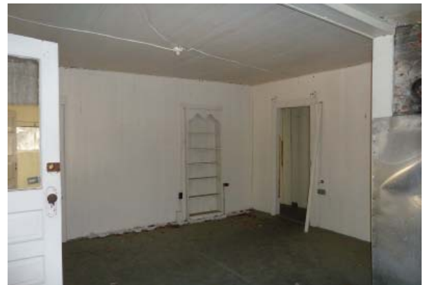
Figure 65. Southwest oblique of the Living Room (Room 102).
