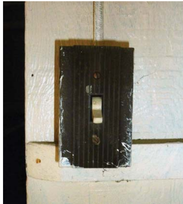
Figure 87. Light switch with mid-twentieth century brown plastic plate on the east wall of Room 106.
