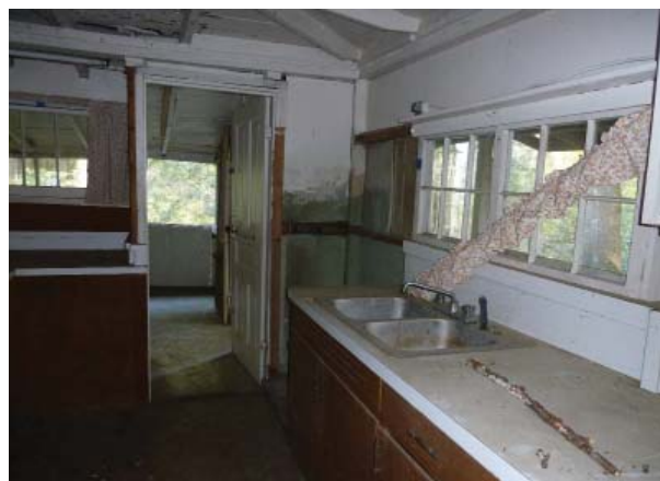
Figure 78. Northwest oblique of Room 105.
