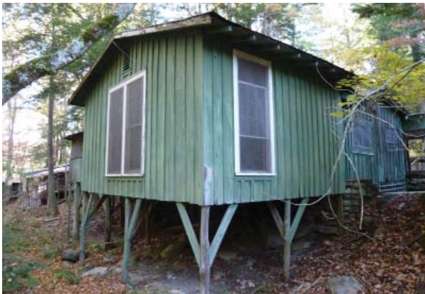
Figure 56. Nine-over-nine-light windows of the southwest addition.
