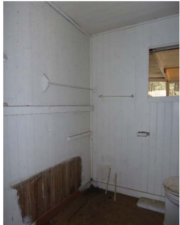
Figure 89. Southwest oblique of Room 107.
