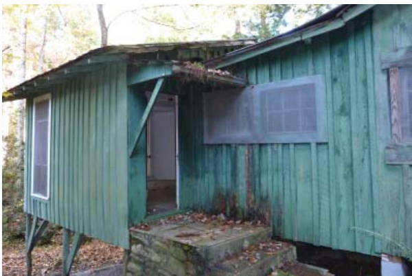
Figure 57. Paired windows arranged horizontally at the south elevation.
