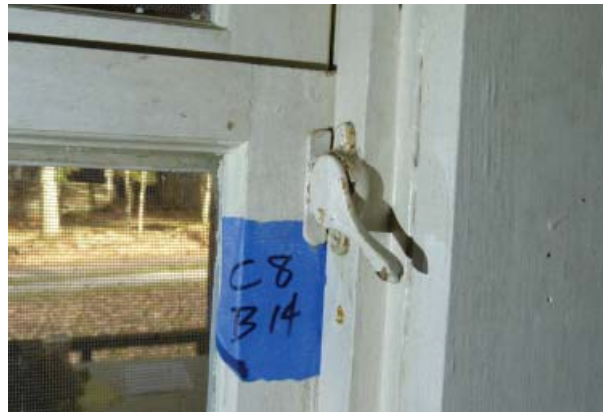
Figure 63. Jamb-mounted compression latch on the window.
