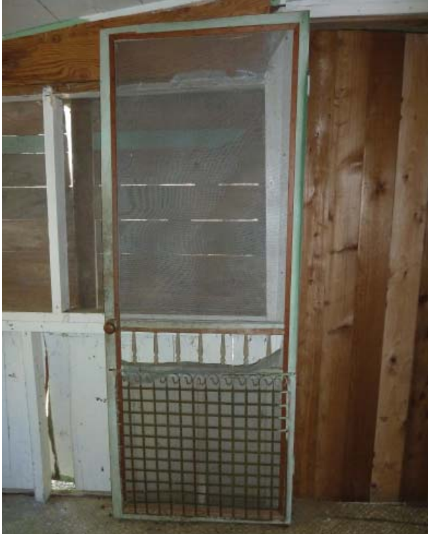
Figure 49. Screened door of Enclosed Porch (Room 106).
