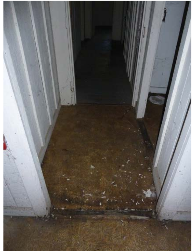
Figure 101. Floor of Room 109b.
