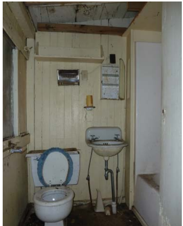
Figure 43. Bathroom fixtures of Room 108.
