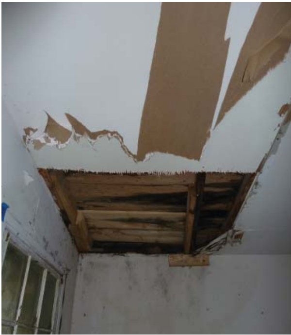
Figure 112. Exposed roof rafters and decking in the ceiling of Room 112.
