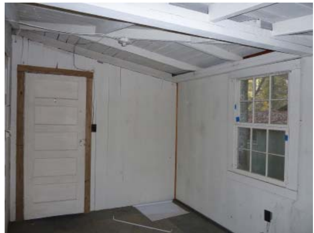
Figure 71. Northwest oblique of Room 103.
