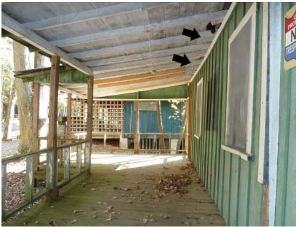
Figure 37. Front porch with overhanging roof rafters of the main block.
