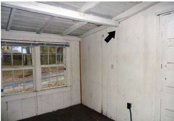
Figure 38. Porch rafters and header (foreground) with added rafters in distance, room 103.
