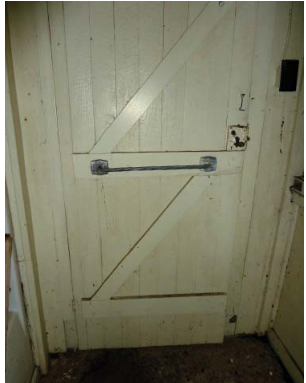
Figure 94. Board-and-batten door of Room 108.
