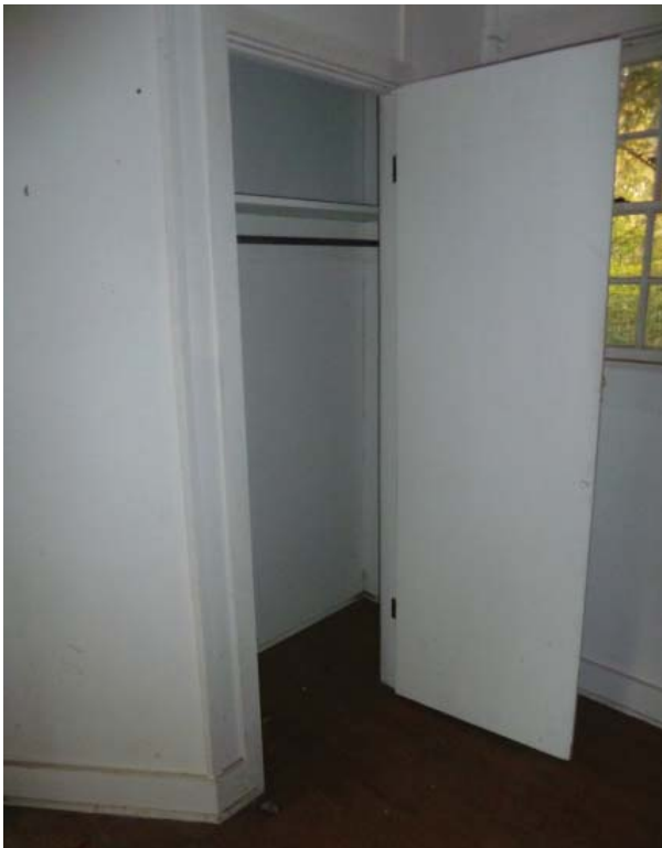
Figure 106. North closet of Room 111.
