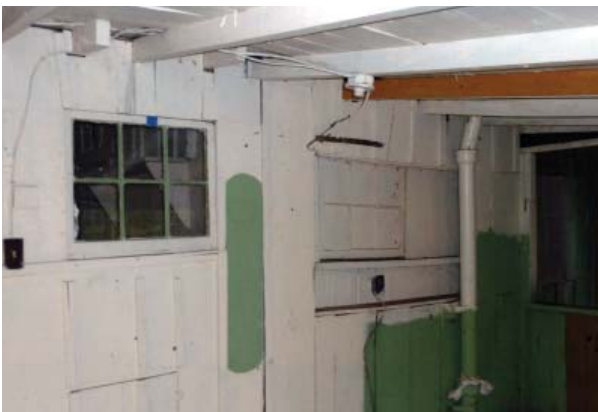
Figure 54. Casement window (left) and sliding window (right) of the enclosed porch.
