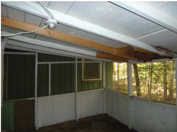
Figure 86. Southwest oblique of Room 106.
