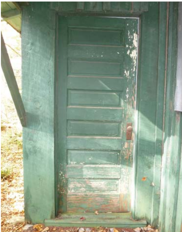
Figure 50. Entrance door, southwest addition, Room 111.
