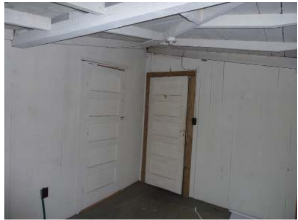
Figure 70. Southwest oblique of Northeast Bedroom (Room 103).
