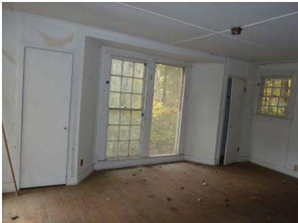
Figure 104. Northwest oblique of the Southwest Addition (Room 111).
