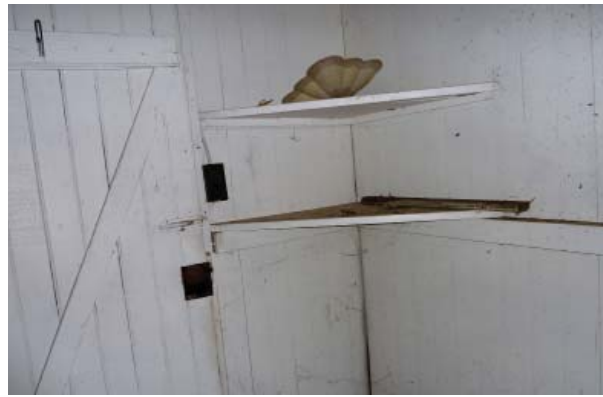
Figure 91. Corner shelves in Room 107.
