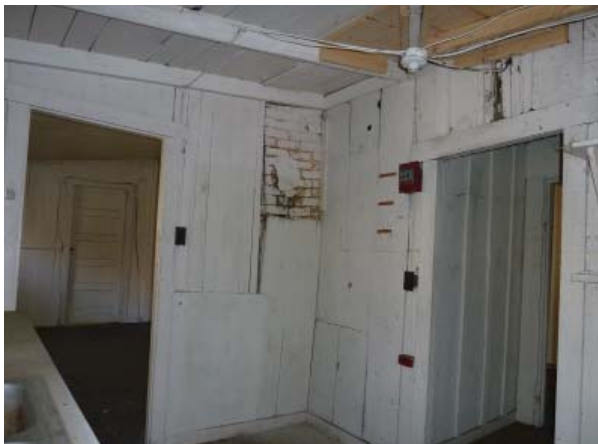
Figure 80. Southeast oblique of Room 105.
