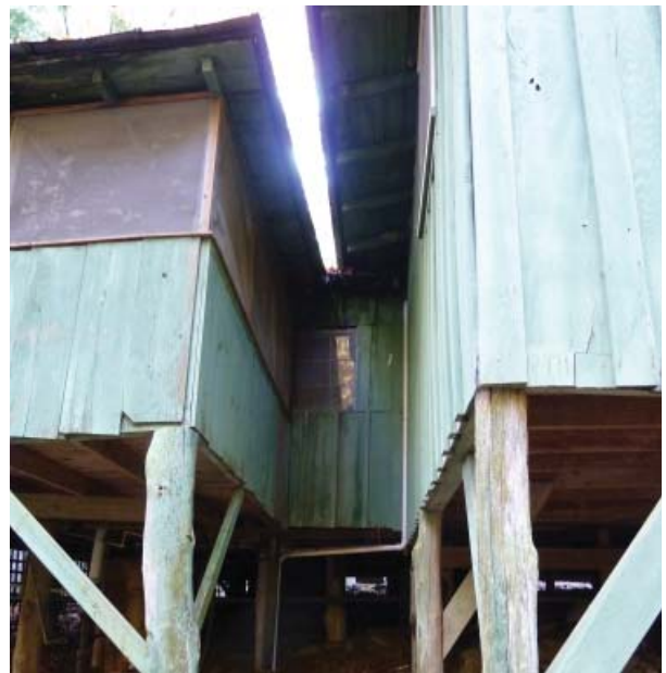
Figure 55. Six-light sash window between the two back additions.
