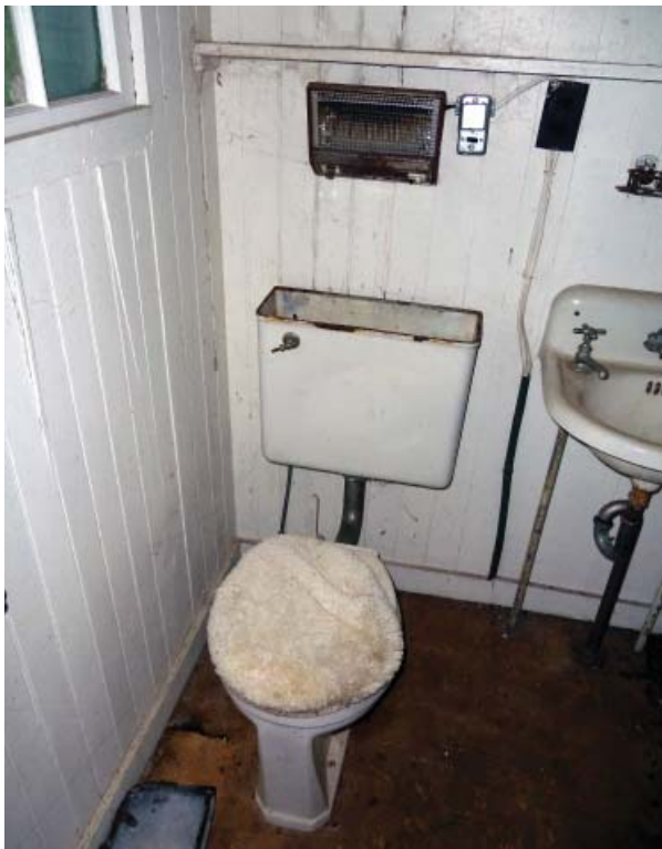
Figure 88. Northwest oblique of the Half-Bathroom (Room 107).
