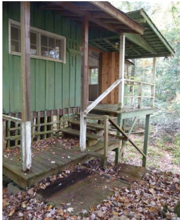
Figure 45. Two levels of the north porch.
