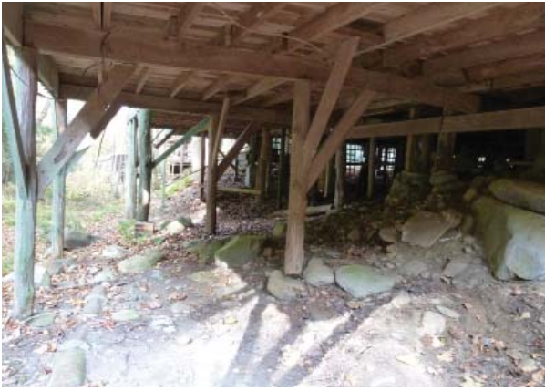
Figure 36. Floor framing and posts below southwest addition.
