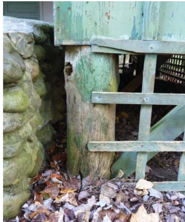
Figure 35. Typical unmilled foundation post.
