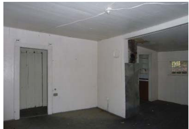
Figure 66. Northwest oblique of Room 102.
