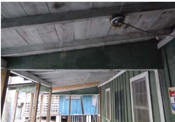
Figure 44. Remains of a dividing wall at the front porch.
