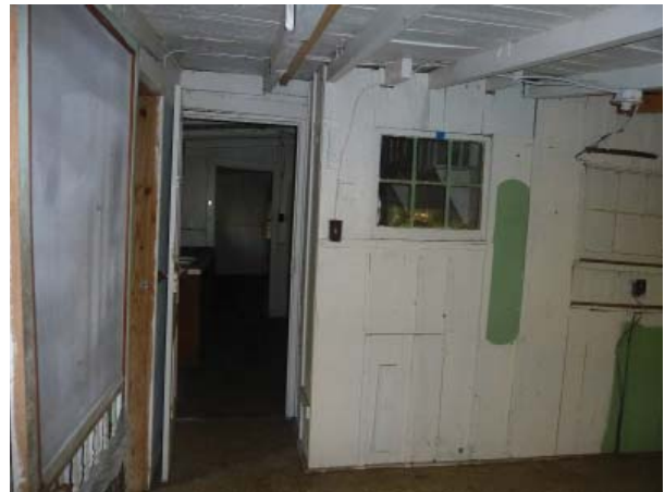
Figure 84. Enclosed porch (Room 106) looking east toward the Kitchen (Room 105).
