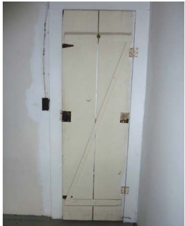
Figure 111. Board-and-batten door and light switch on the north wall of Room 112.
