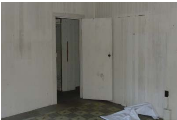
Figure 62. Board-and-batten door on the west wall of Room 101b.
