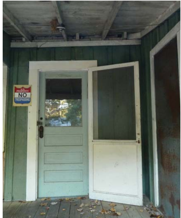
Figure 47. Front door with screen door at the east elevation.
