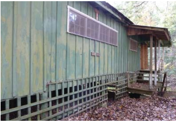
Figure 52. Four early window sash reused on the north elevation.
