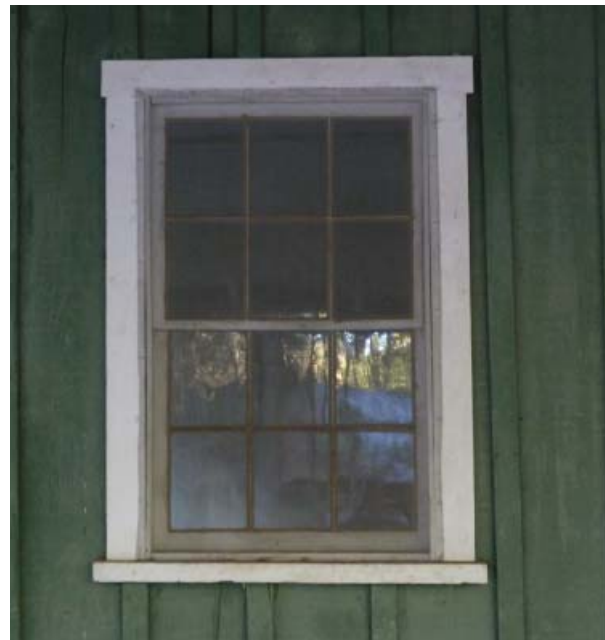
Figure 51. Original south window on the east elevation with Type B sash, Room 101a.
