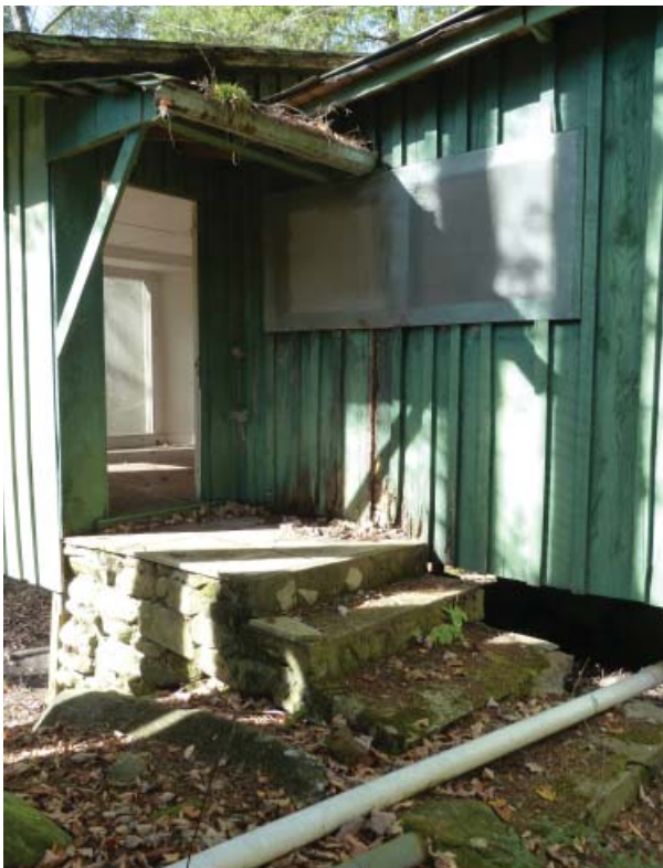
Figure 30. South patio and entrance to Room 111.
