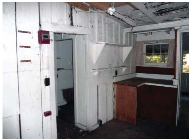
Figure 77. Southwest oblique of the Kitchen (Room 105).
