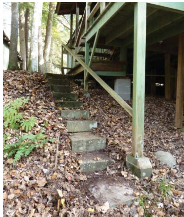
Figure 31. View of north steps from the back yard looking east.
