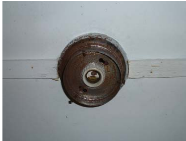
Figure 108. Chrome-plated light fixture of Room 111.
