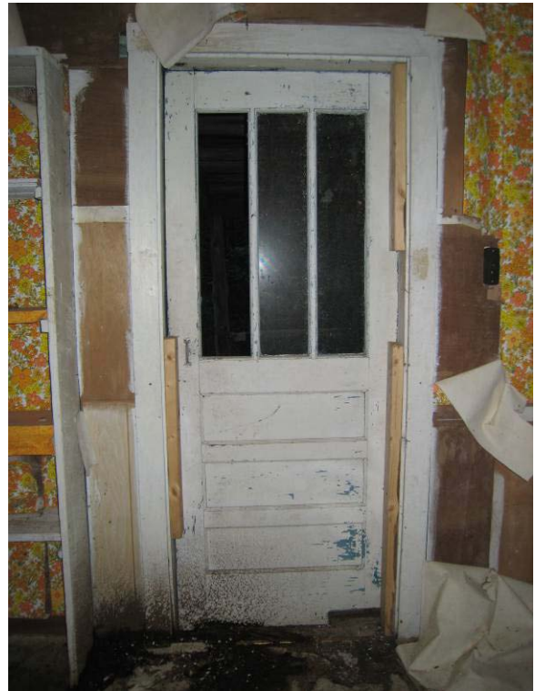
Figure C- 9. Exterior Door in Room 102.
