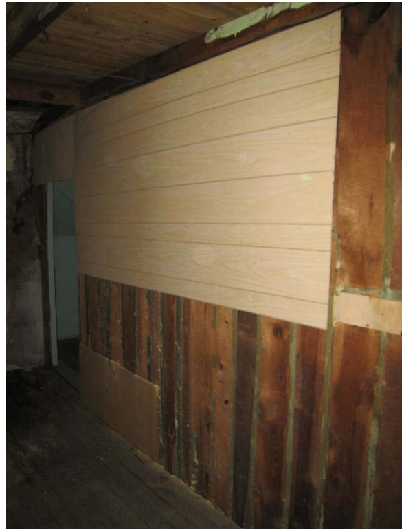
Figure C- 48. Room 201, north wall.
