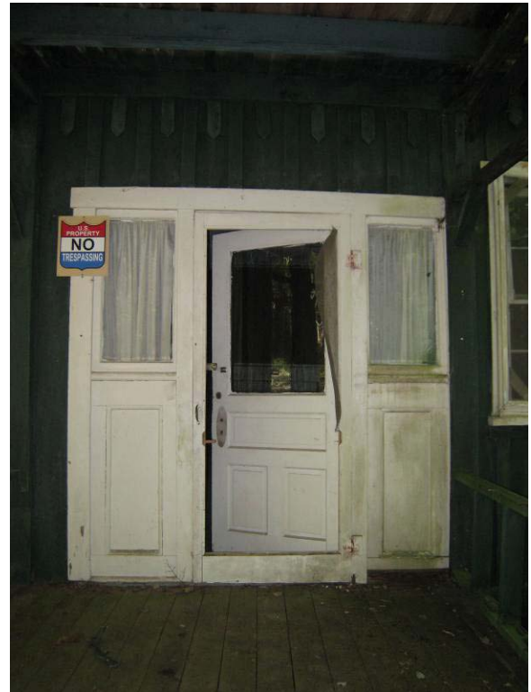
Figure C- 7. Front screen and exterior door.
