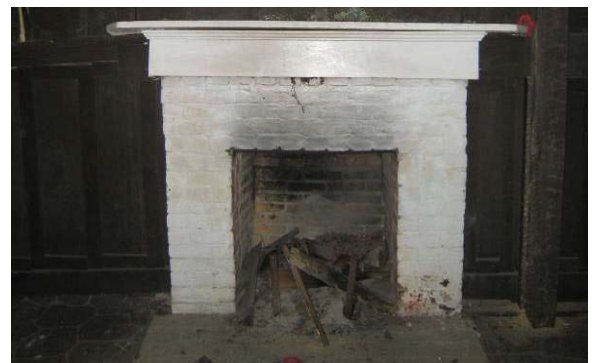
Figure C- 19. Fireplace in Room 101.
