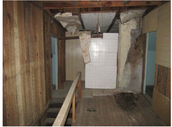
Figure C- 45. Room 201, looking west.
