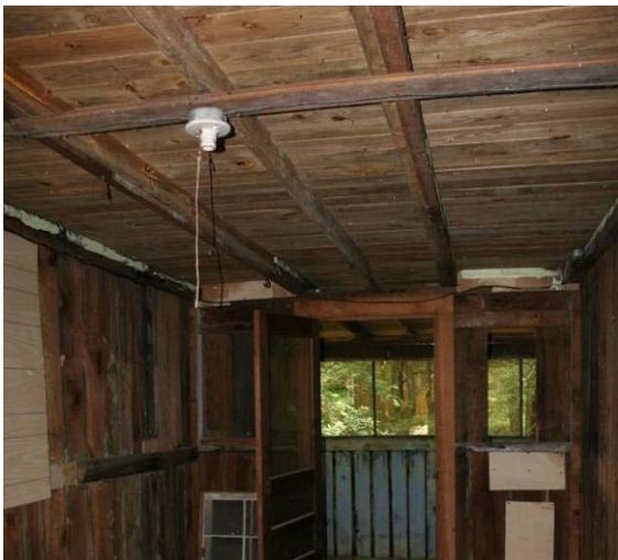
Figure C- 5. Second floor hall looking east with roof framing visible.
