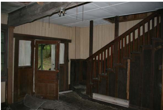
Figure B- 4. Room 101 showing remnants of the Craftsman interior.
