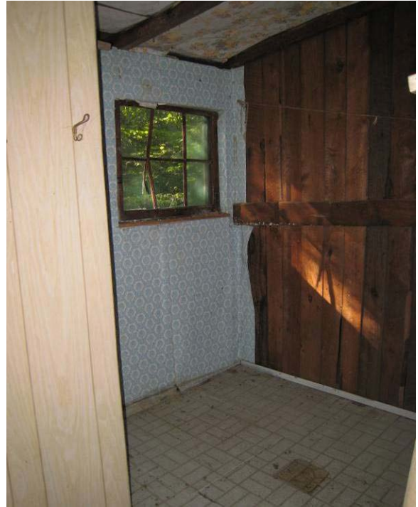
Figure C- 58. Room 203, looking northwest.
