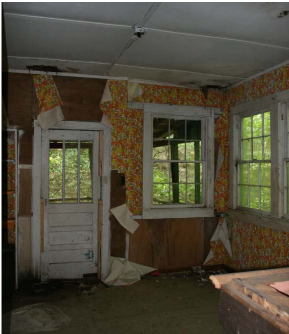
Figure C- 22. Room 102, looking northeast.
