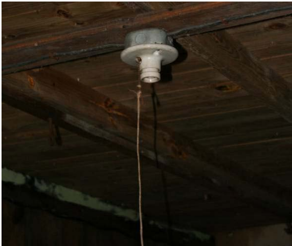
Figure C- 53. Ceramic light socket in Room 201.
