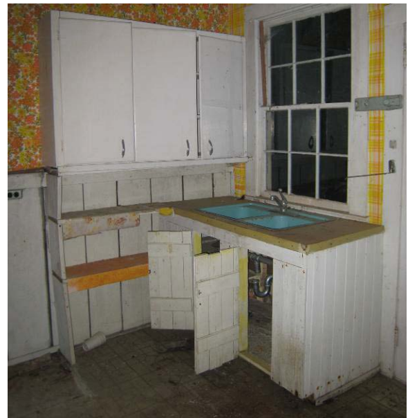
Figure C- 28. Kitchen cabinetry and sink in Room 103.
