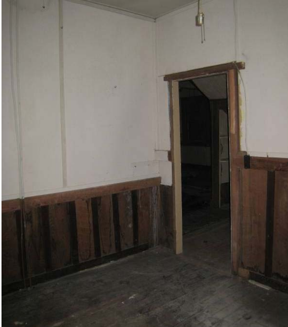
Figure C- 29. Room 104 looking northeast.
