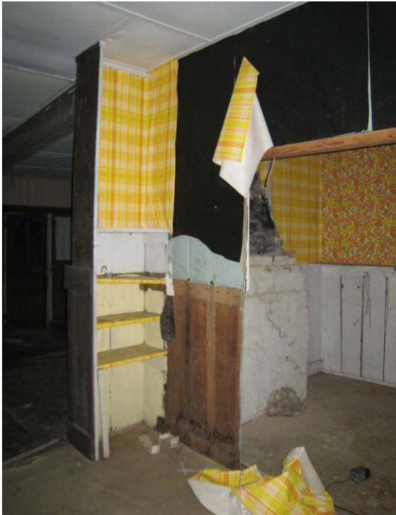
Figure C- 23. Room 102, looking at the southeast corner.
