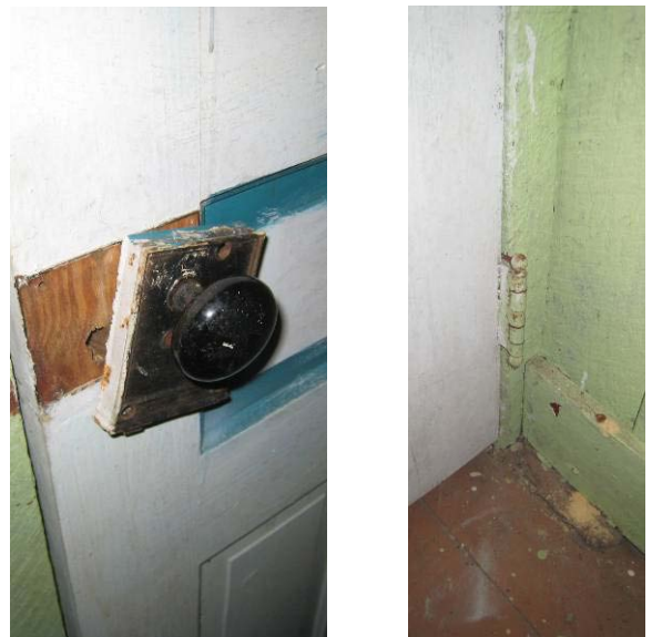
Figure C- 38. Hardware on door to Room 107.
