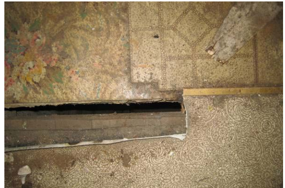
Figure B- 7. Multiple layers of flooring.
