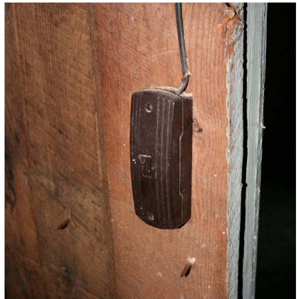
Figure C- 68. Early wall-mounted light switch.
