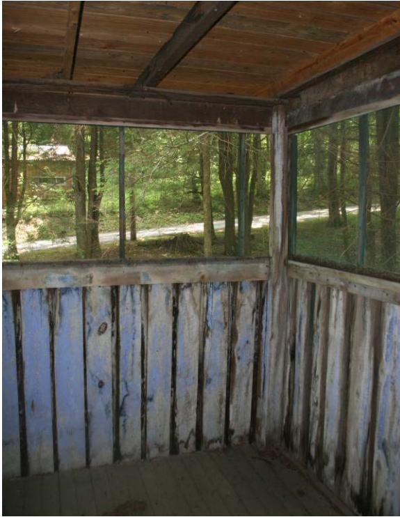
Figure C- 64. Screened-in sleeping porch, Room 205, looking east.
