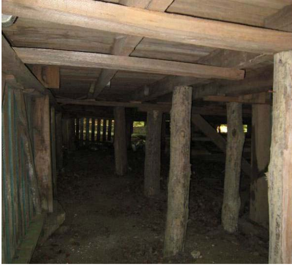
Figure C- 4. Log posts set in the ground, support girders and joists.
