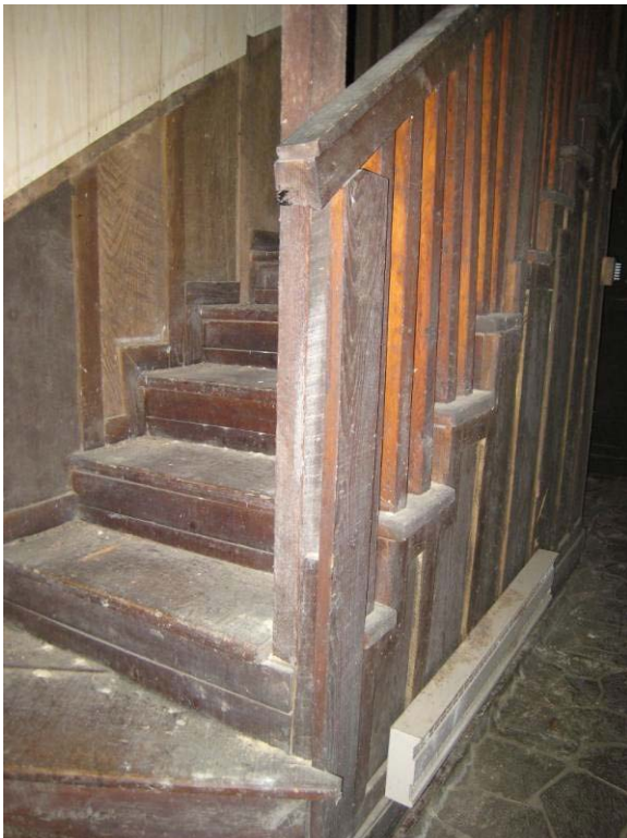
Figure C- 20. Stairway in Room 101.
