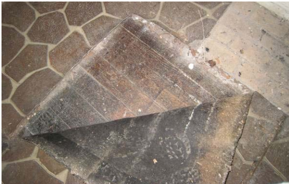
Figure C- 17. Original hardwood floor under sheet vinyl flooring in Room 101.
