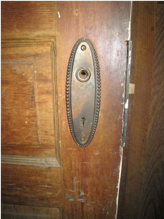
Figure C- 8. Decorative escutcheon and dead bolt at interior face of front exterior door.
