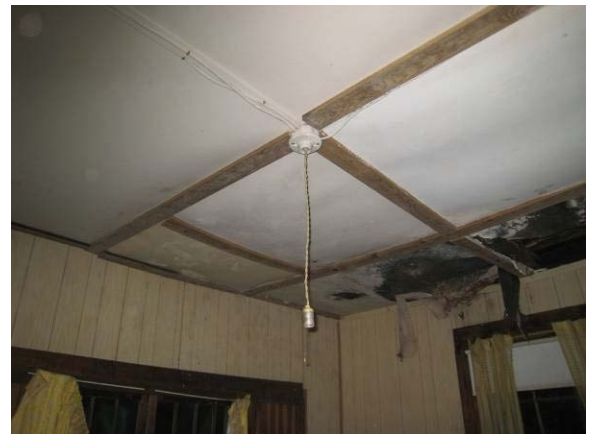
Figure C- 32. Ceramic light socket in Room 104.
