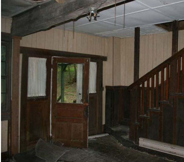
Figure C- 16. Room 101 looking toward the southeast.
