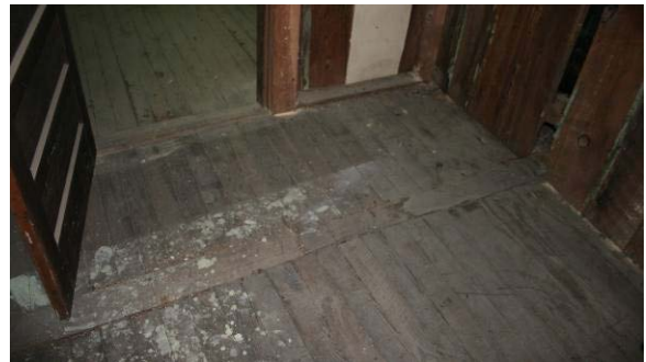
Figure C- 46. Transverse floorboard in Rm. 201.
