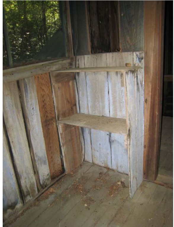
Figure C- 65. Room 205, looking southwest.
