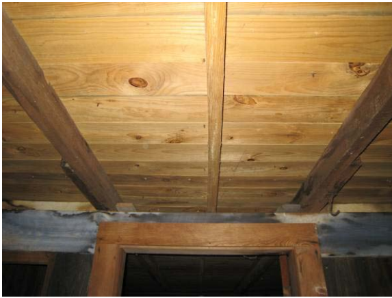
Figure C- 66. Looking west at the exposed rafters and deck boards in Room 205.
