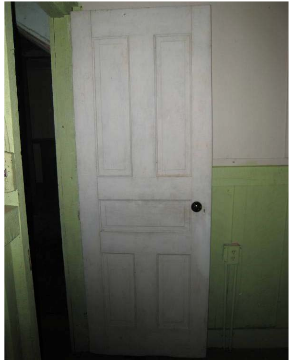
Figure C- 37. Door to Room 107.
