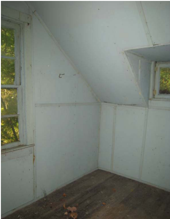
Figure C- 62. Room 204, looking northeast.
