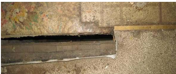
Figure C-26. Multiple layers of vinyl flooring in the Room 103 (top half) and Room 102 (bottom half).
