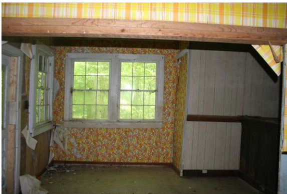
Figure C- 24. Room 102's north wall.
