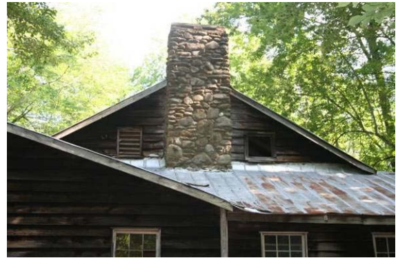
Figure A- 9. The 1934 Appalachian Clubhouse showing uses of natural materials and simple geometric forms.
