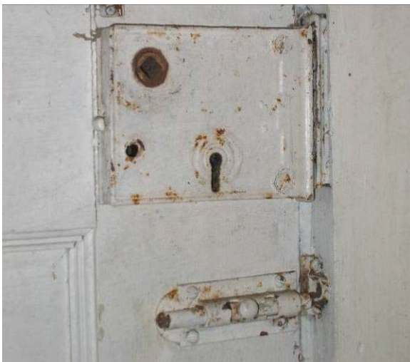
Figure C- 11. Rim lock and barrel bolt on door in Room 103.
