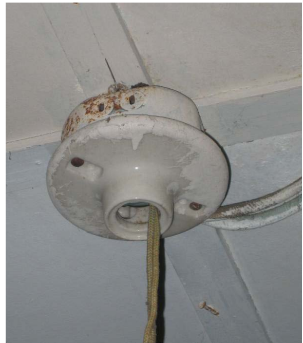
Figure C- 42. Ceramic light socket in Room 107.
