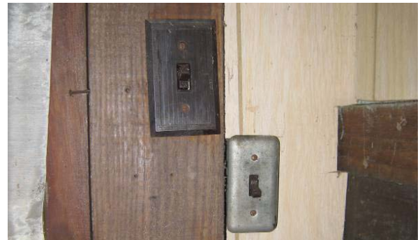
Figure C- 18. Toggle light switches in Room 101.
