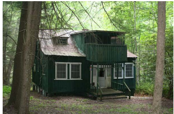
Figure C- 1. Chapman-Byers Cabin viewed from the southeast showing the sleeping porch addition over the front porch.
