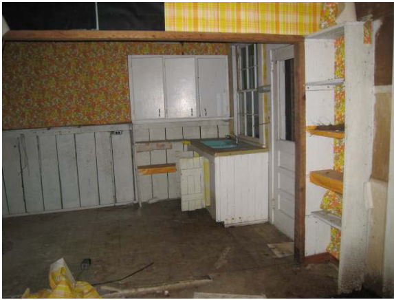
Figure C-25. Room 103, or the kitchen, looking south from Room 102.
