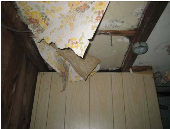
Figure C- 60. Ceiling in Room 203.
