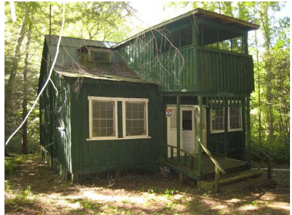
Figure B- 1. Front, east, elevation.
