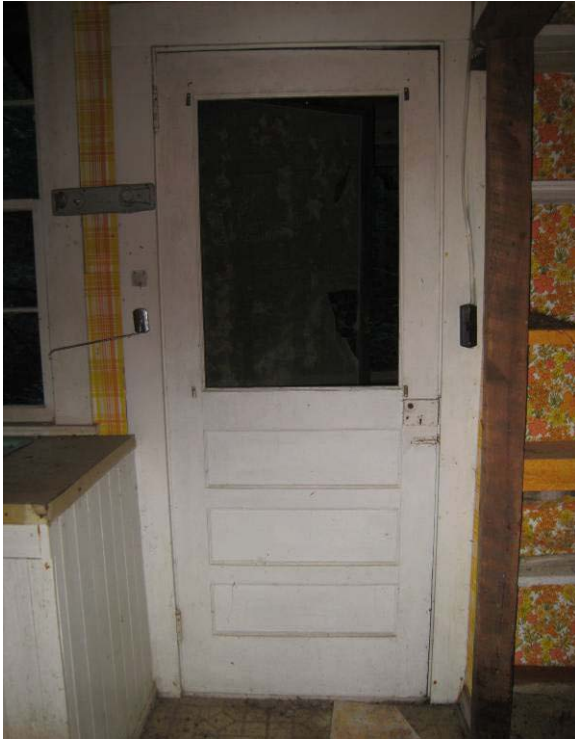
Figure C- 10. Exterior Door in Room 103.
