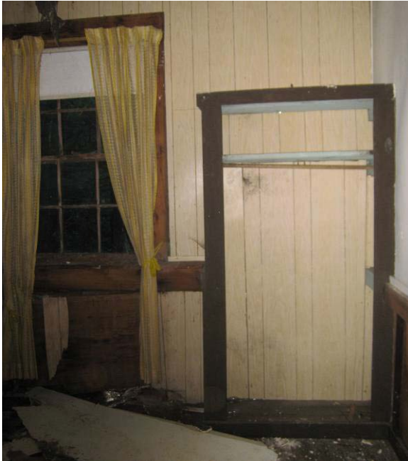
Figure C- 33. Storage closet at west wall of Room 104.
