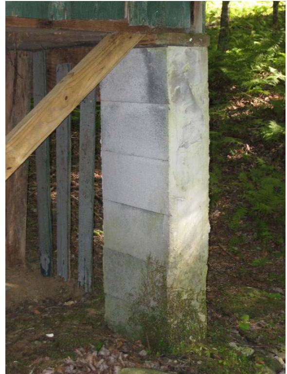
Figure C- 3. New CMU pier.
