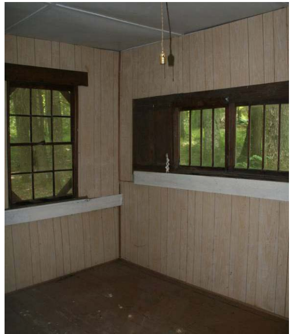
Figure C- 41. Room 107, looking southeast.
