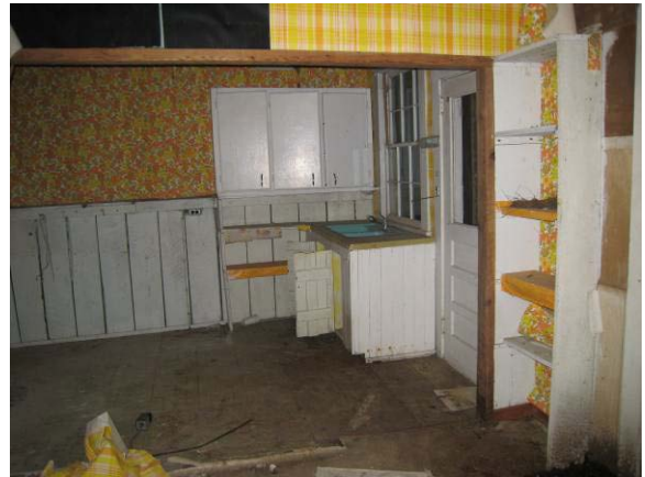
Figure B- 10. Enlarged opening between Rooms 102 and 103.
