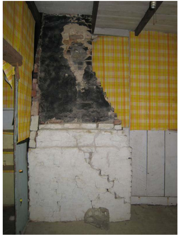
Figure C-27. East wall of Room 103.
