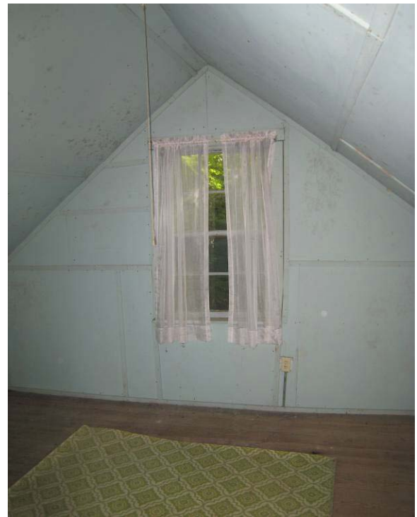
Figure C- 54. Room 202, looking south.
