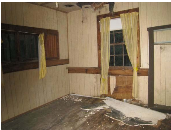
Figure C- 30. Room 104 looking southwest.
