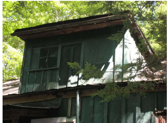
Figure C- 59. West dormer, showing in-filled window opening (right).
