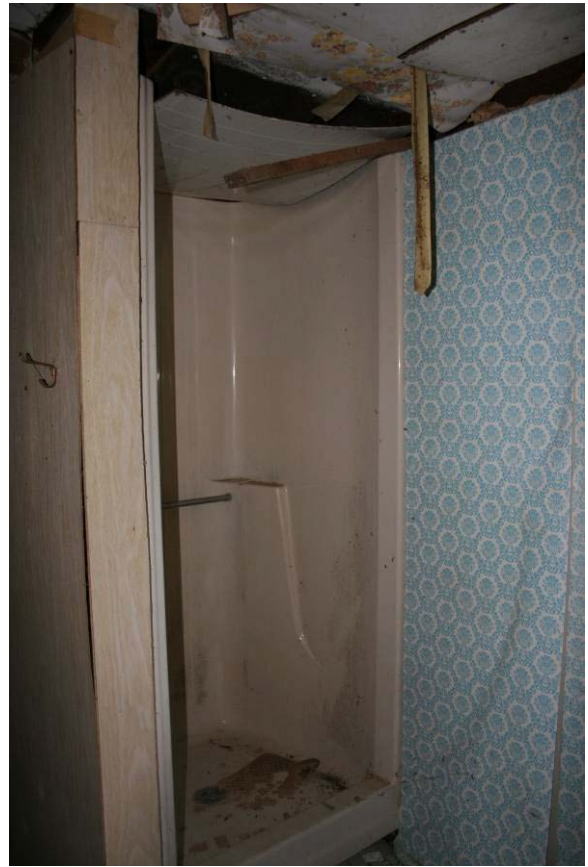
Figure C- 61. Prefabricated shower stall unit in Room 203.
