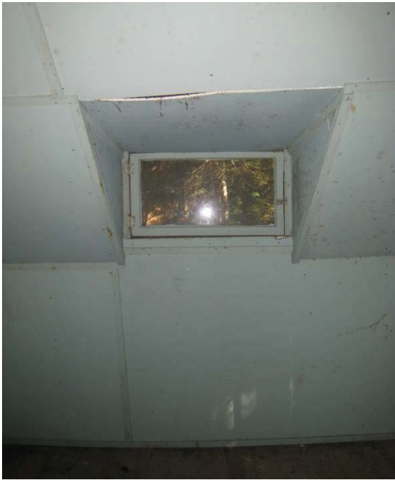
Figure C- 55. Room 202, looking east.
