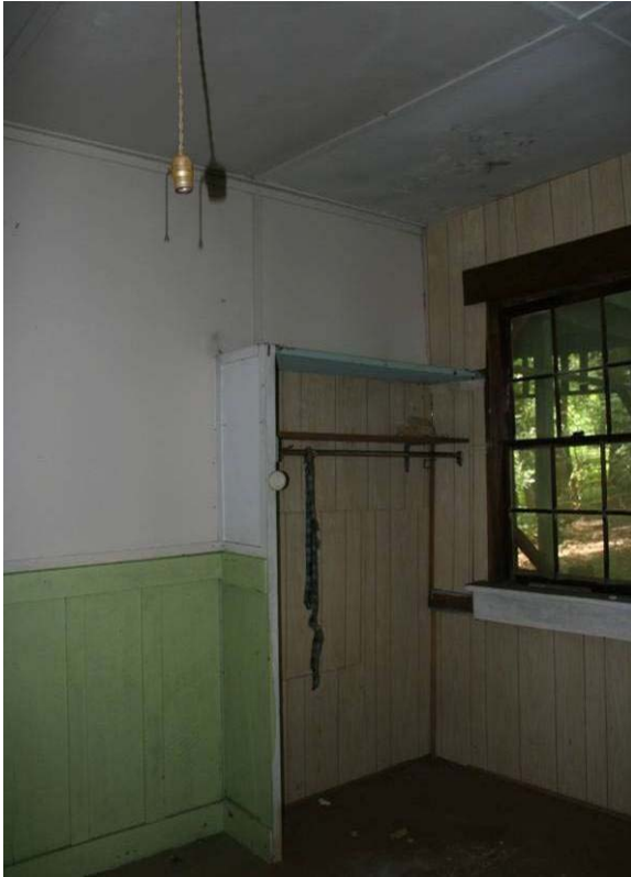
Figure C- 43. Storage closet at northeast corner.
