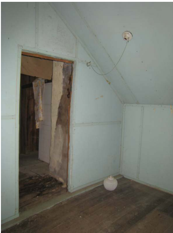
Figure C- 63. Room 204, looking southwest.
