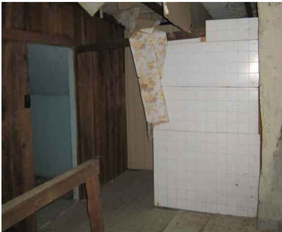
Figure C- 51. Room 201, west wall.
