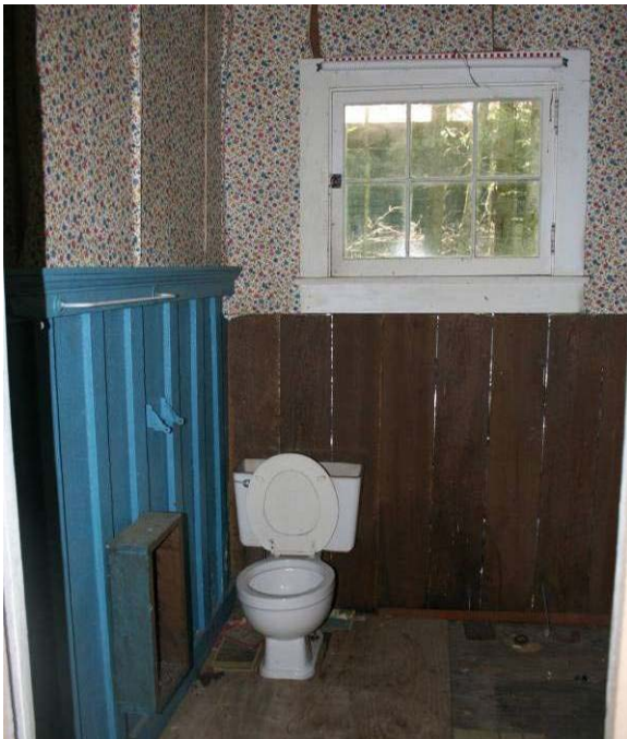
Figure C- 34. Room 105 looking south.
